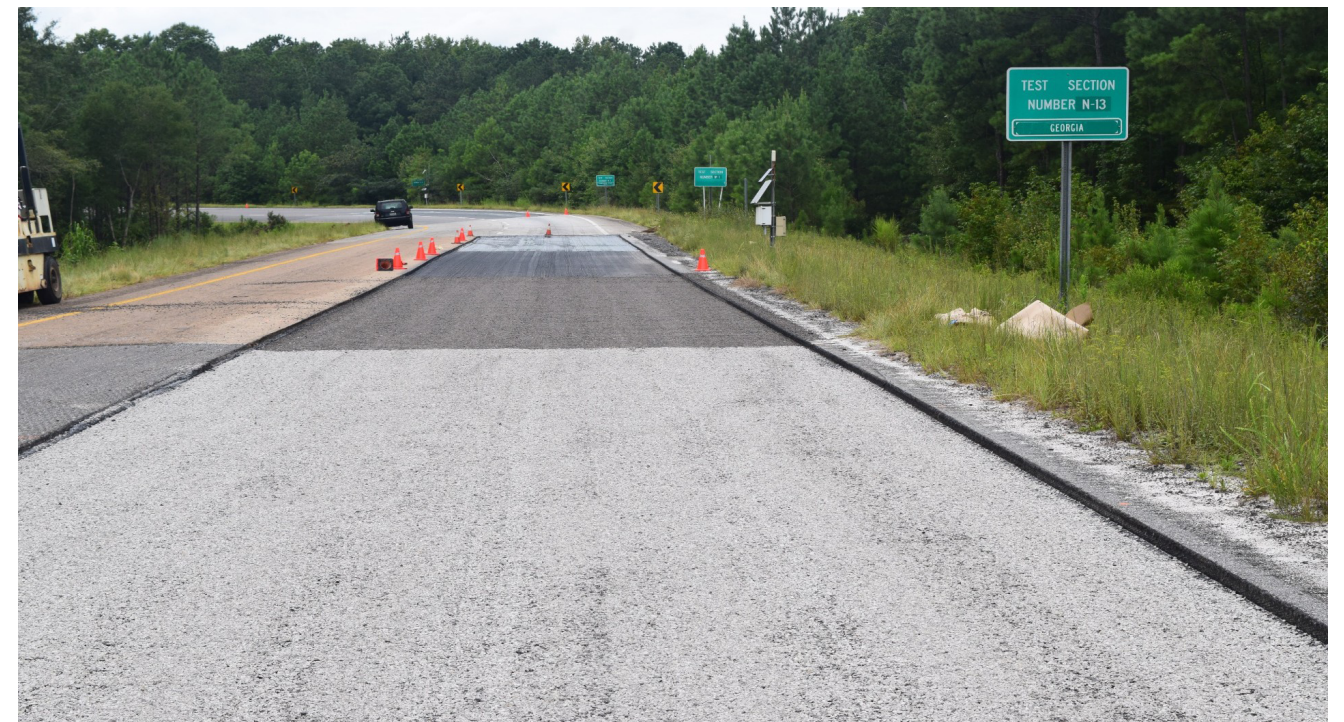
Figure 13. Interlayer section on NCAT Test Track
