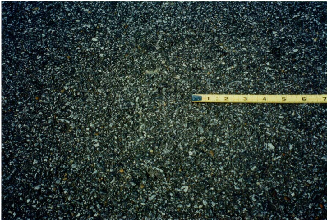
Figure 9. Tallapoosa Project - Closeup of Dense-Graded Wearing Course Mix After 3-3/4 Years
