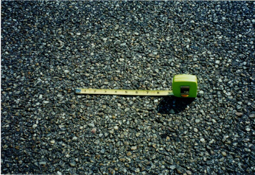
Figure 8. Tallapoosa Project - Closeup of Gravel Novachip Surface After 3-3/4 Years
