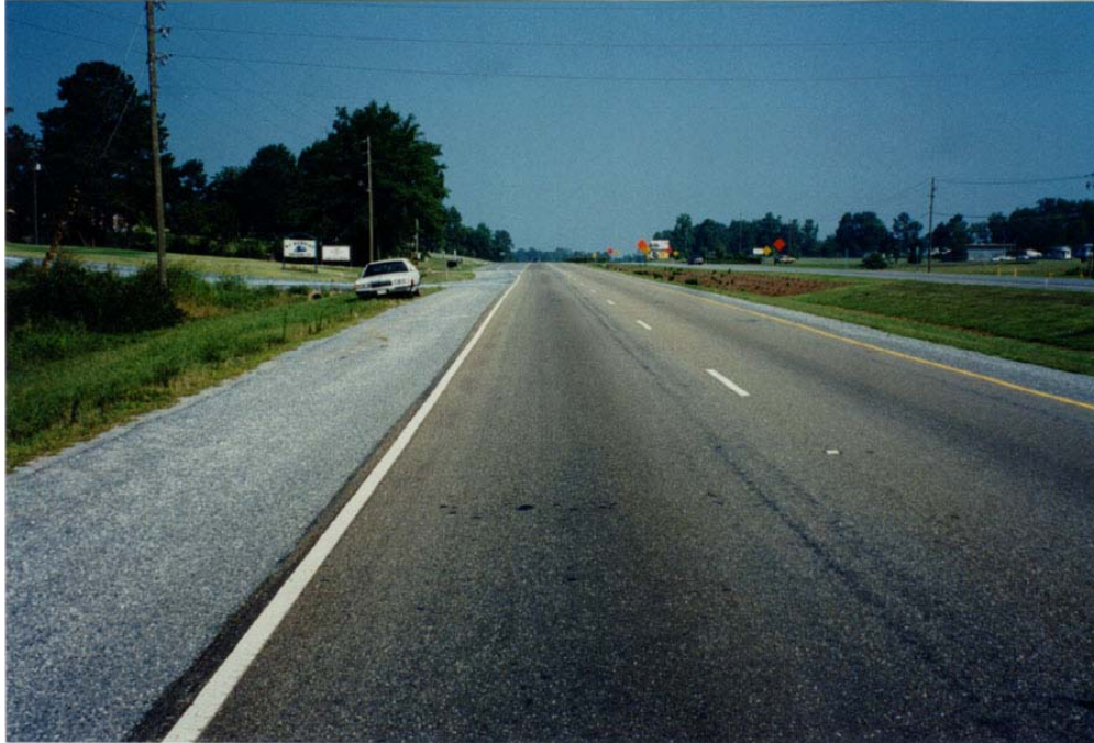
Figure 7. Tallapoosa Project - Gravel Section Showing Slight Flushing in Travel Lane (Left) and no Flushing in Passing Lane (Right)
