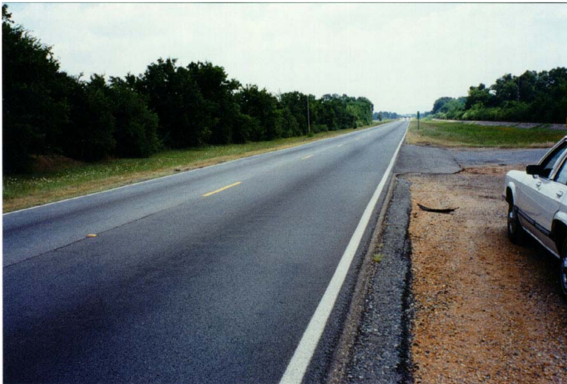
Figure 10. Talladega Project - General Uniform Appearance of Novachip Surface
