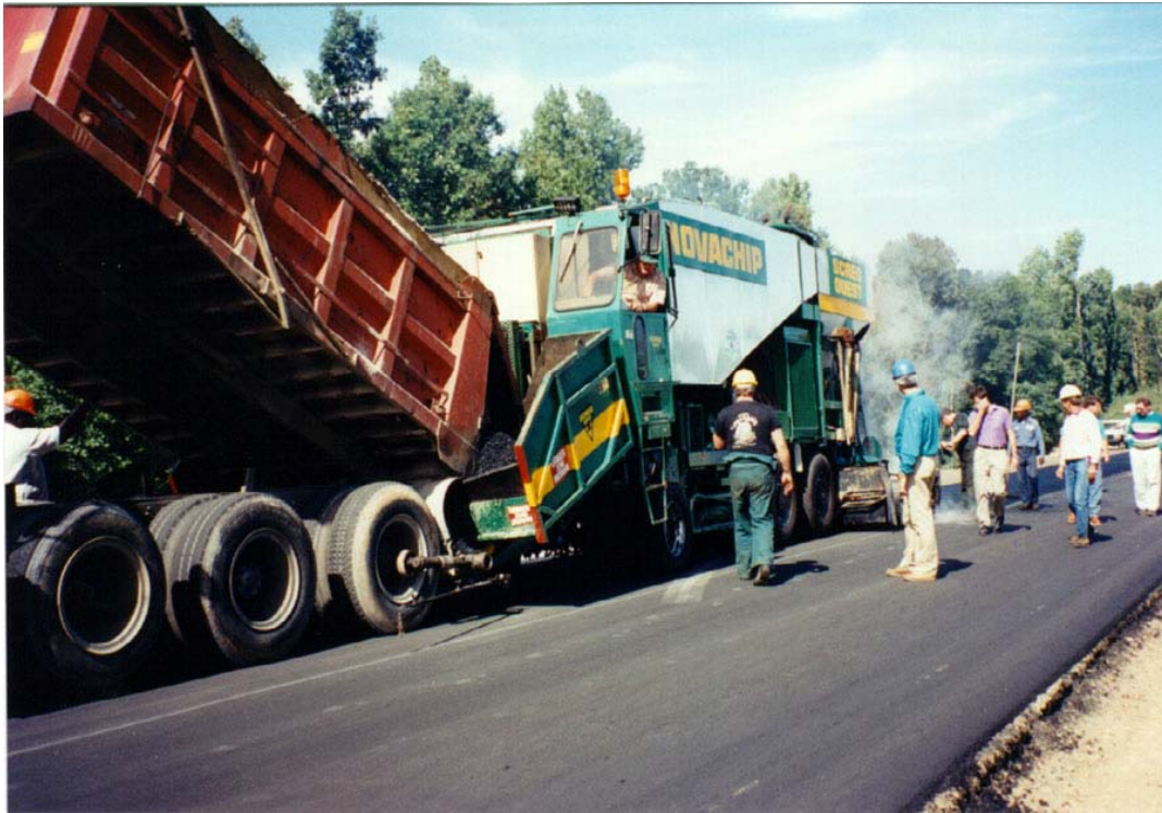
Figure 3. Truck Discharging Mix into Hopper
