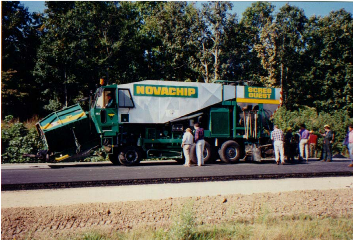
Figure 2. Novachip Paving Machine Used in Alabama
