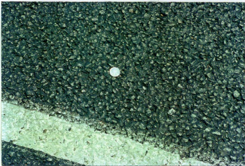
Figure 16. Close-Up Showing Coarse Aggregate Surface Texture
