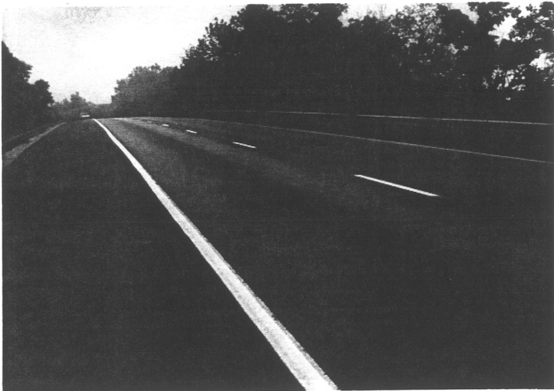
Figure 80. Project 32, I-70 (E.B.), Fulton County
