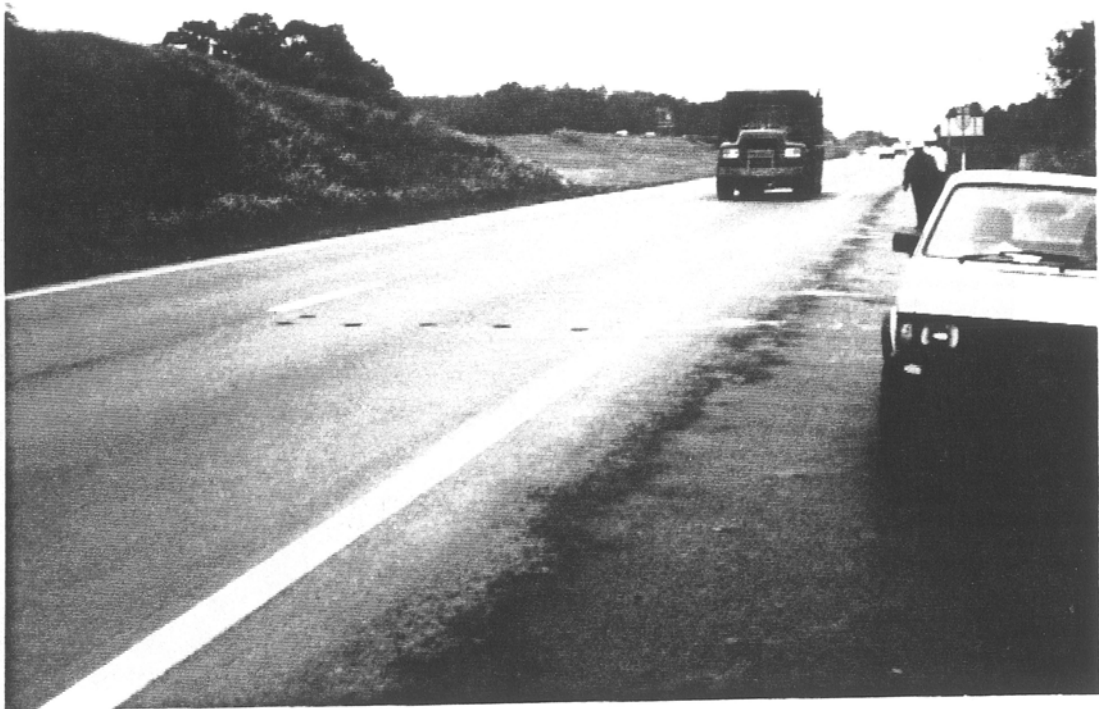
Figure 60. Project 13, I-81 (S.B.) Luzerne County
