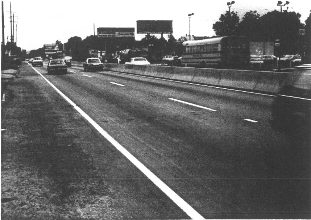
Figure 67. Project 20, Route 222, Berks County
