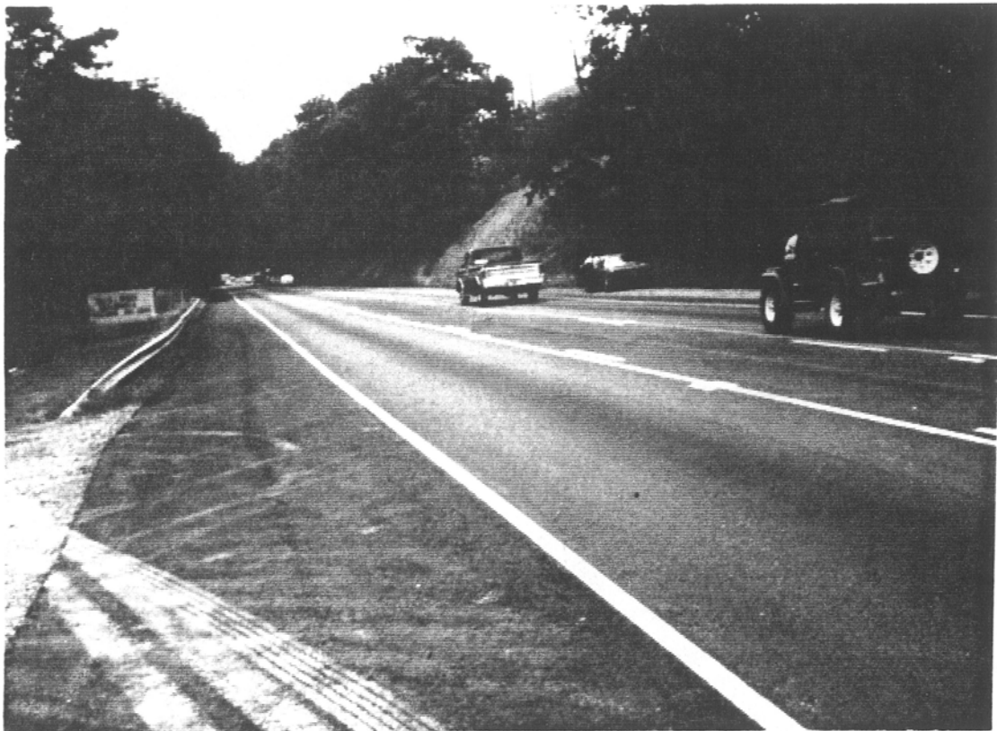
Figure 74. Project 28, Route 22, Dauphin Boro
