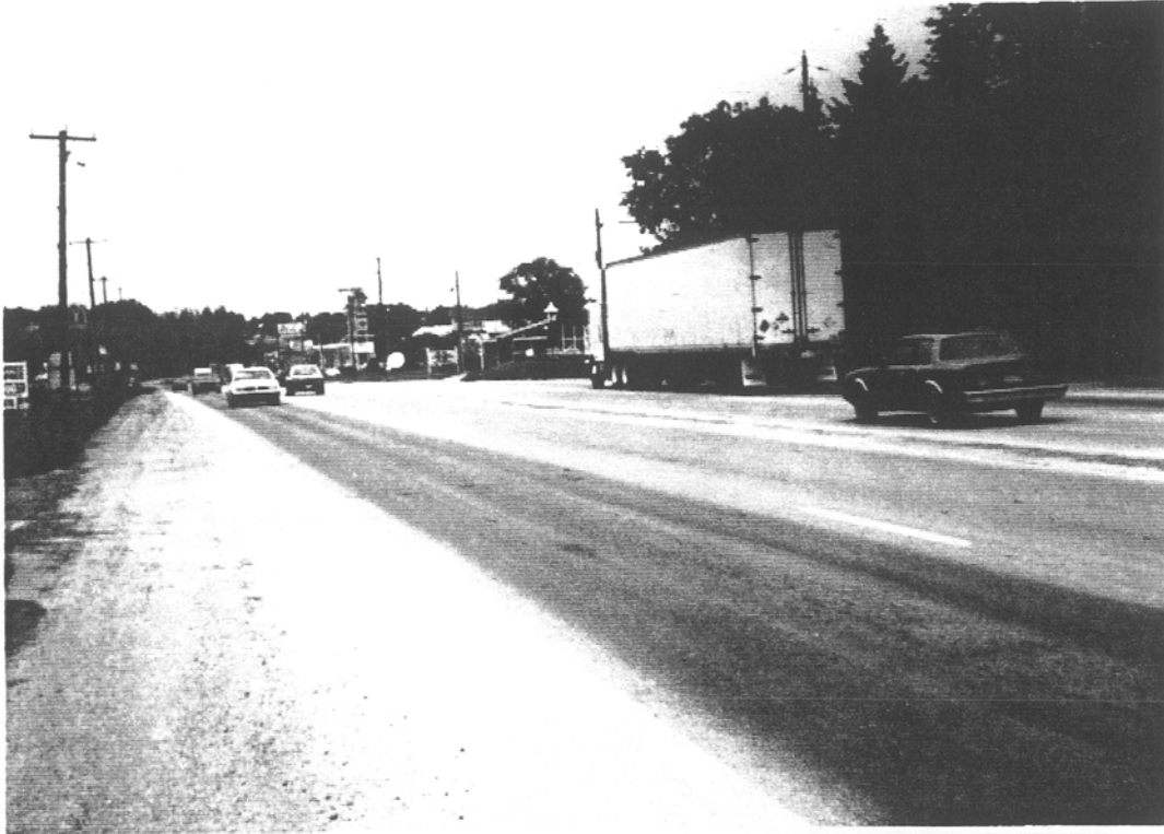
Figure 77. Project 30, Route 11 (Between Mechanicsburg and Carlisle)
