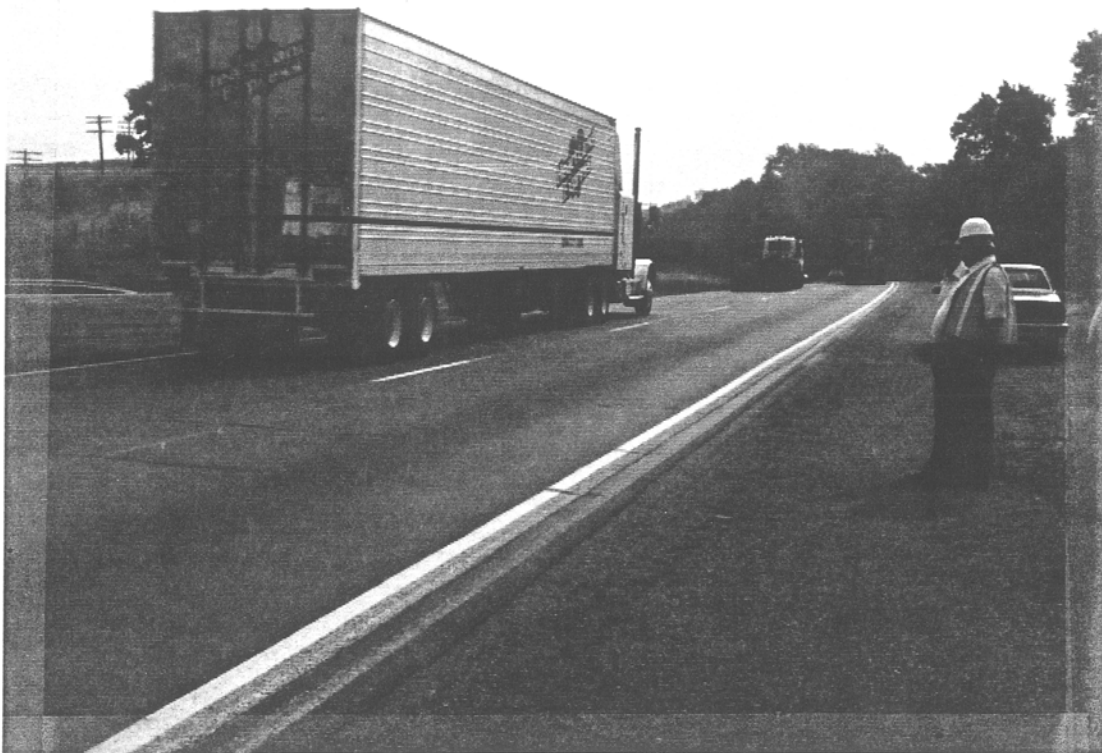
Figure 56. Project 7, I-70 (E.B.)
