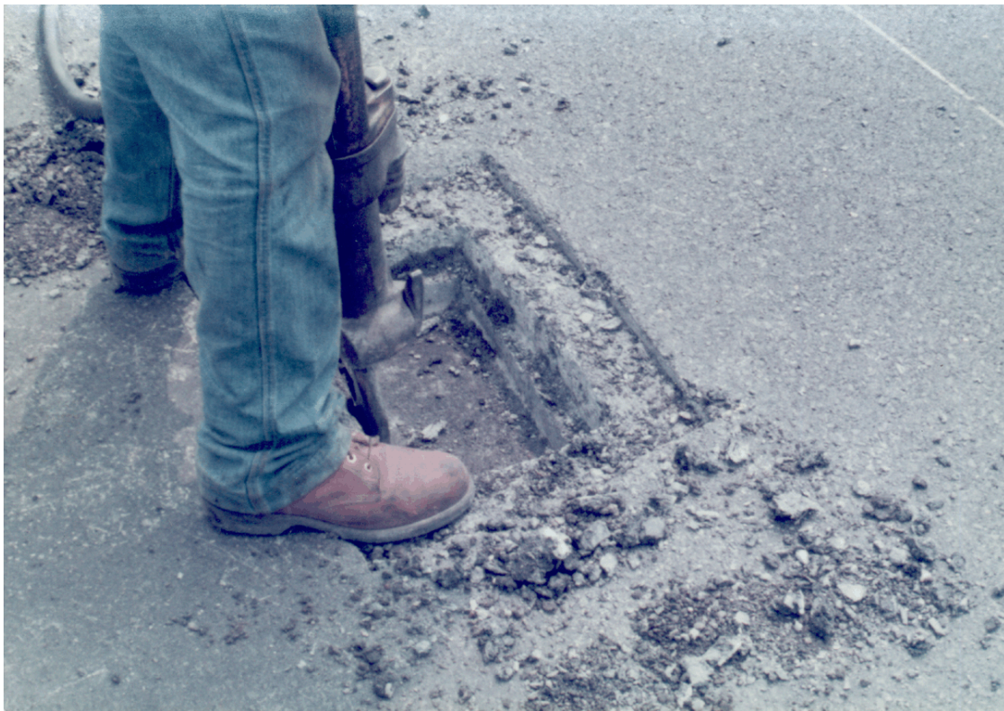
Figure 13. East-West Turnpike (Wearing, Binder, and Leveling Courses Removed)
