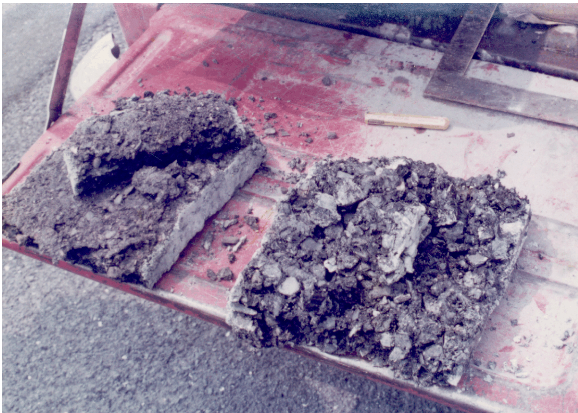
Figure 15. East-West Turnpike (Removed Slabs Placed Upside-Down to Show Stripping)
