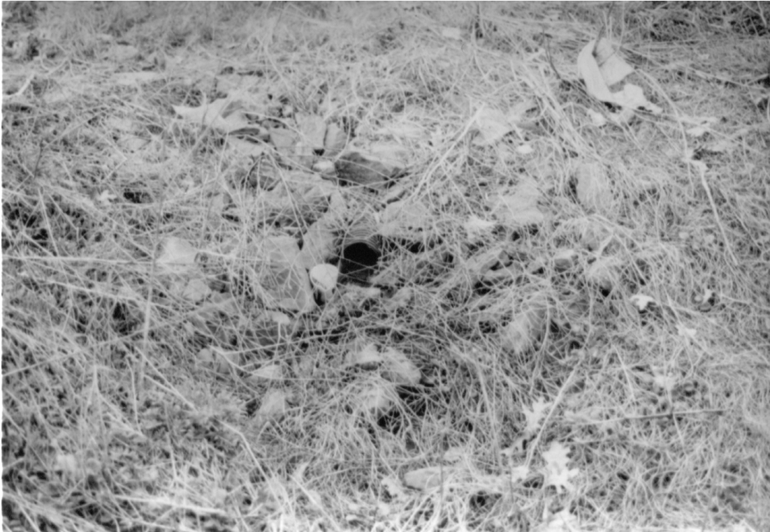
Figure 22. Outlet of the Pavement Edge Drain
