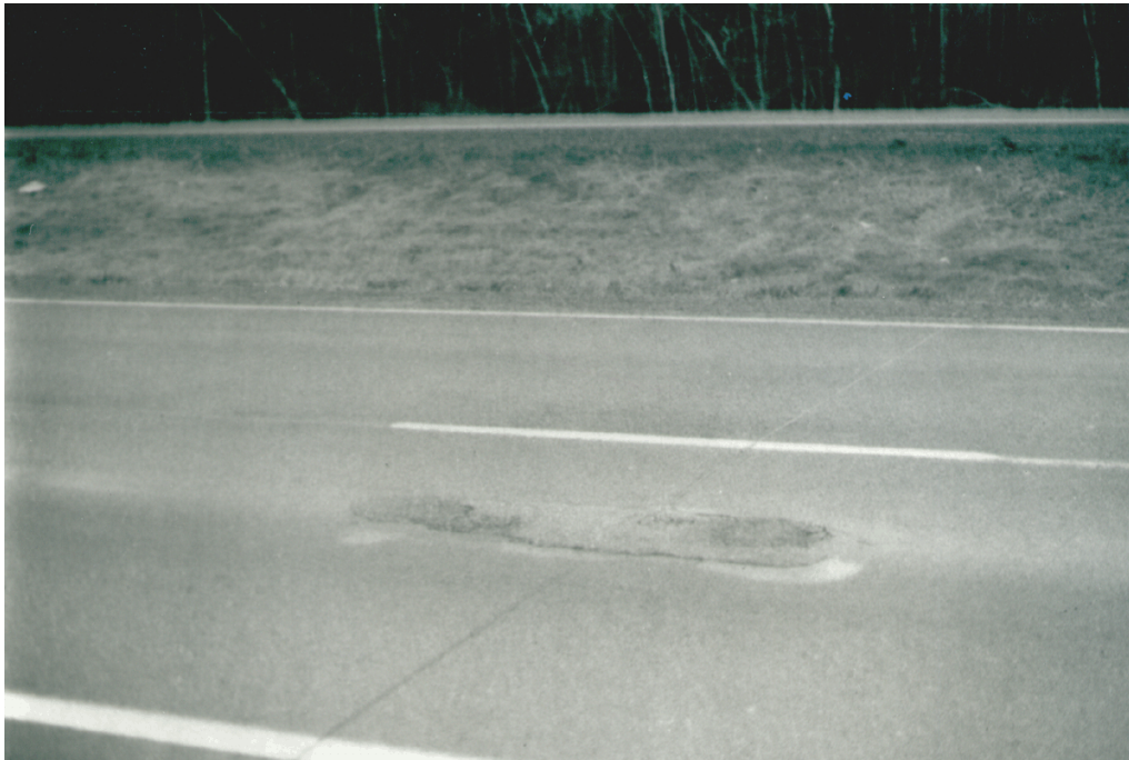
Figure 21. Patched Pothole in Asphalt Overlay on Either Side of Transverse Joint of Underlying PCC Pavement
