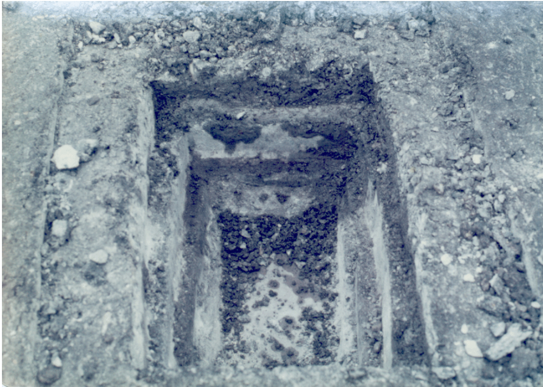
Figure 14. East-West Turnpike (Older Overlays Removed)
