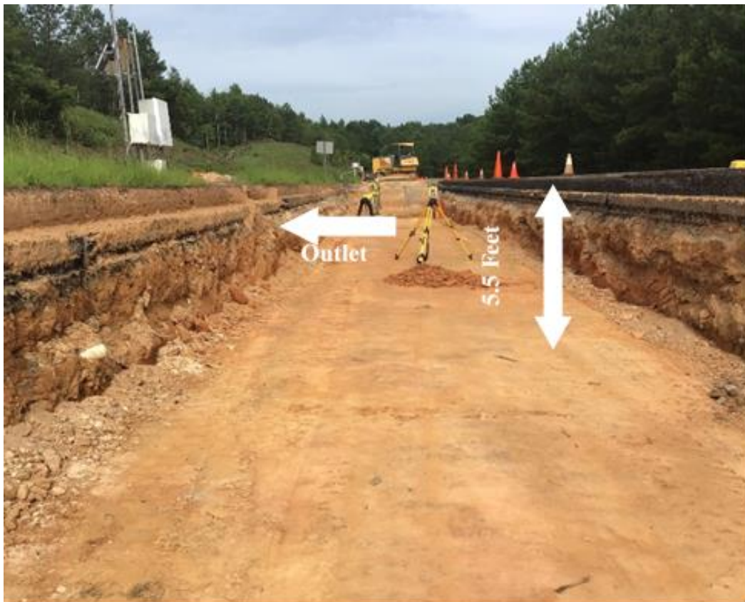
Figure 3. Section S2 Excavation
