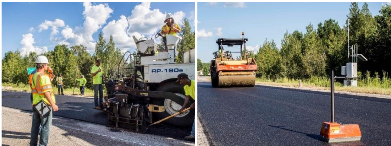
Figure 5. Construction of Section S11 with a Volumetric Mix
