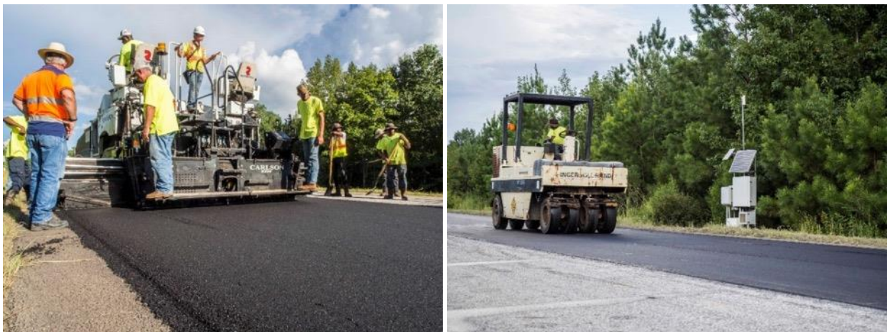
Figure 5. Construction of Section N9
