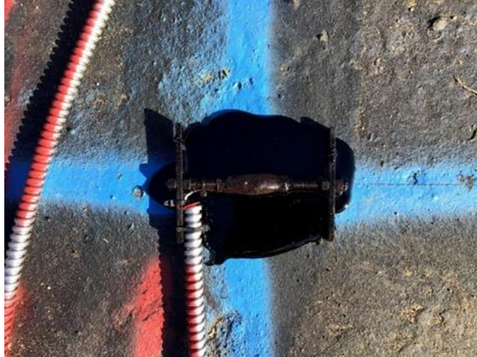
a) ASG Tacked in Place with Sand/Asphalt Mixture
