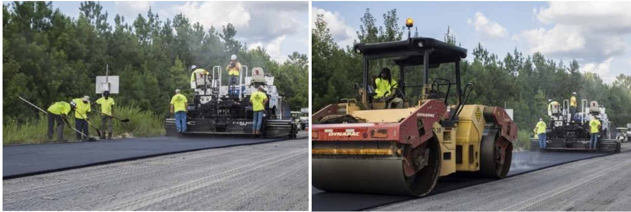
Figure 5. N10 Mix Placement and Compaction
