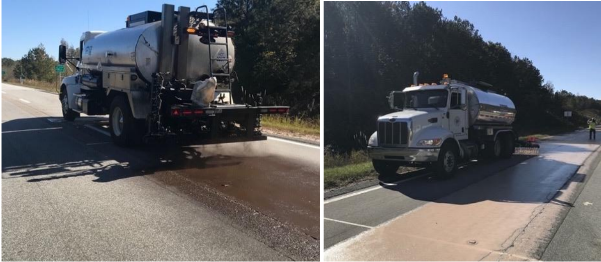
Figure 36. S4-A and S4-B Application of Spray-on Rejuvenators
