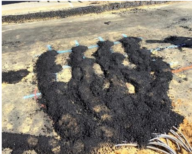
c) ASGs covered with Sieved Mix Prior to Paving
