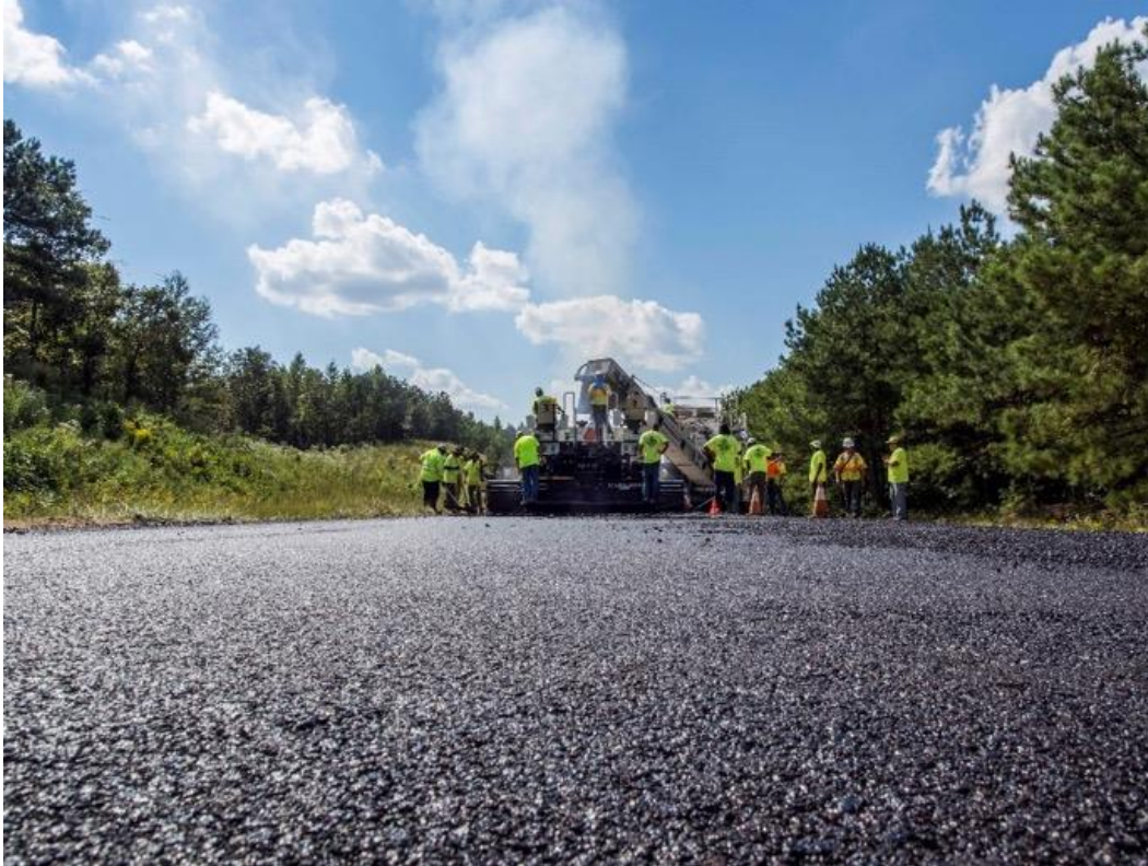
Figure 2. Paving a Test Section for the 2018-2021 Research Cycle
