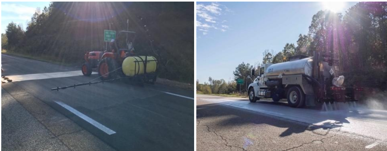
Figure 35. S3-A and S3-B Application of Spray-on Rejuvenators
