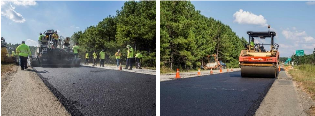
Figure 6. Construction of the Base Layer of Section S1
