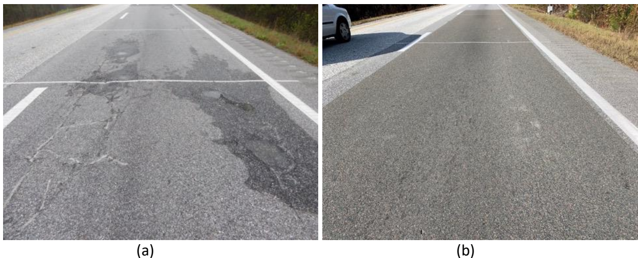
Figure 1. Overview of a) Control and b) Micro Surfacing Test Sections
