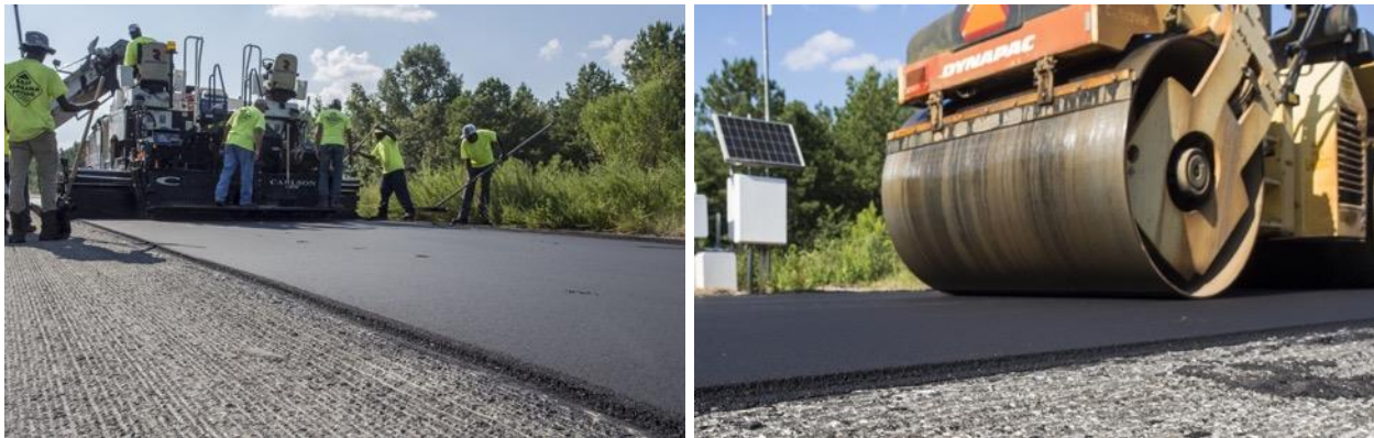
Figure 6. N11 Mix Placement and Compaction
