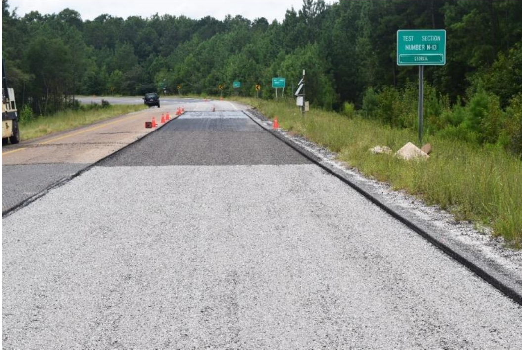
Figure 4. Chip Seal with No. 7 Stone (12C) and Reclaimed Asphalt Pavement (13A)
