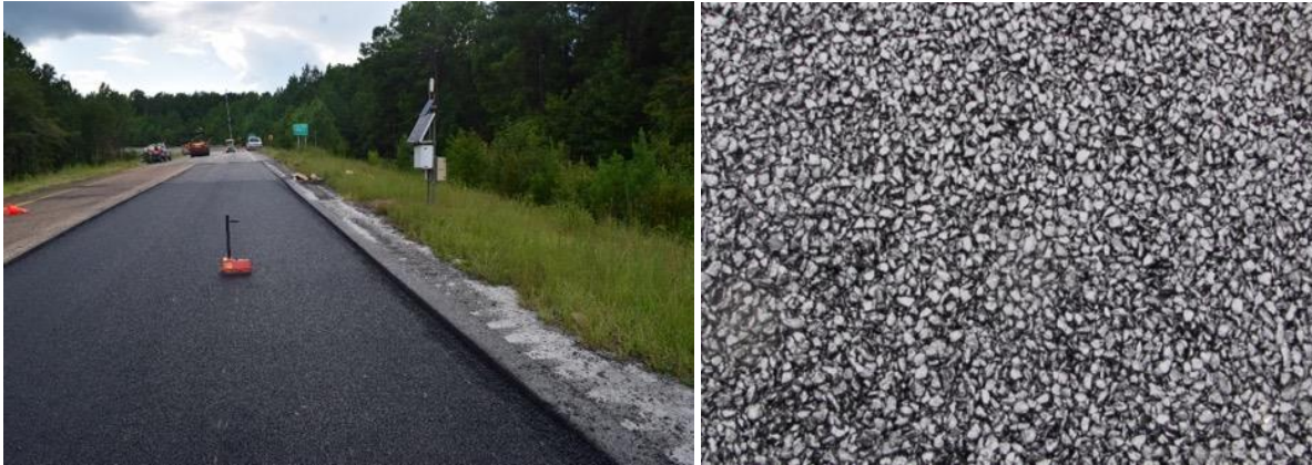
a. Rubber Modified Asphalt Interlayer
