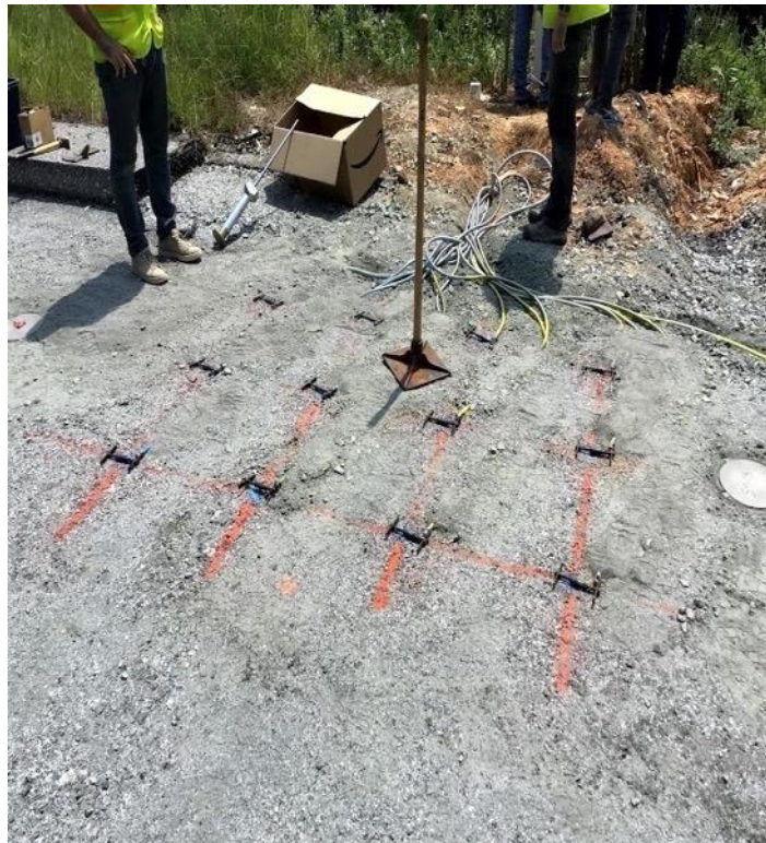
a) Pre-Placement of Instrumentation
