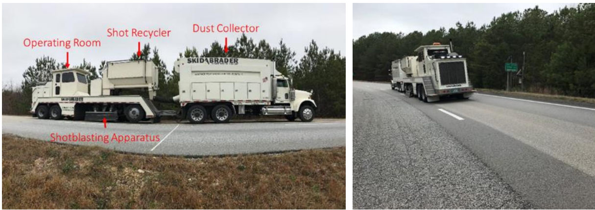
(a) Shotblasting System
