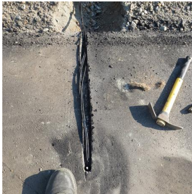
Figure 10. Installed Thermocouple Bundle Prior to Covering with Roofing Asphalt
