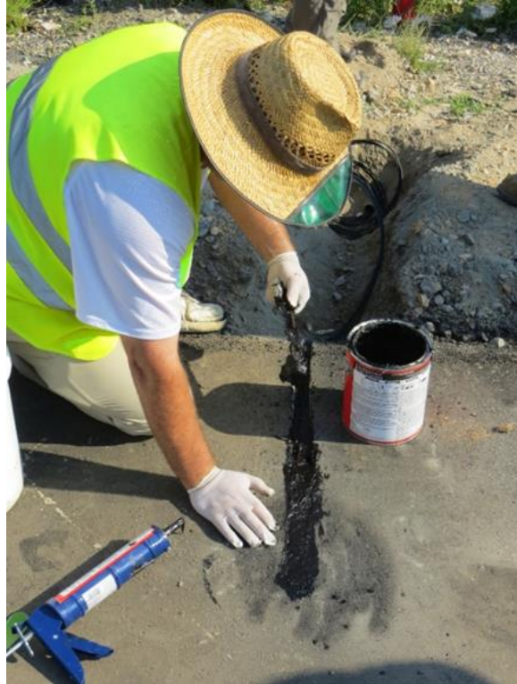
Figure 8. Covering Thermocouple Bundle with Roofing Asphalt
