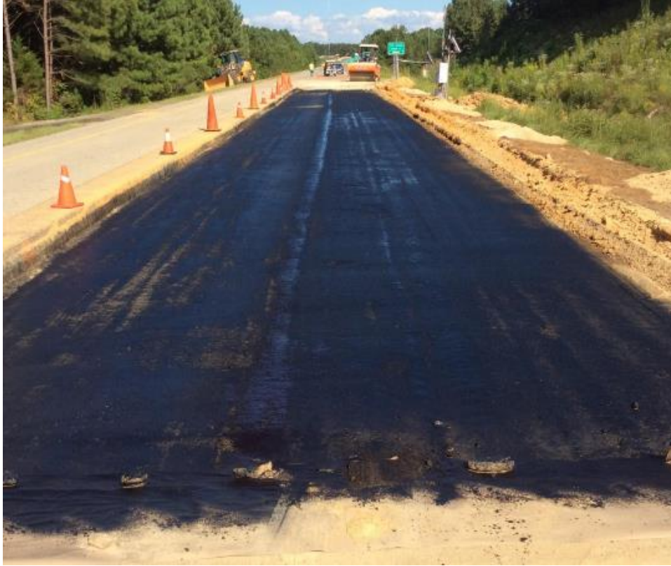
Figure 7. Completed CTB in Section S2 Shortly After Tack Coat Application
