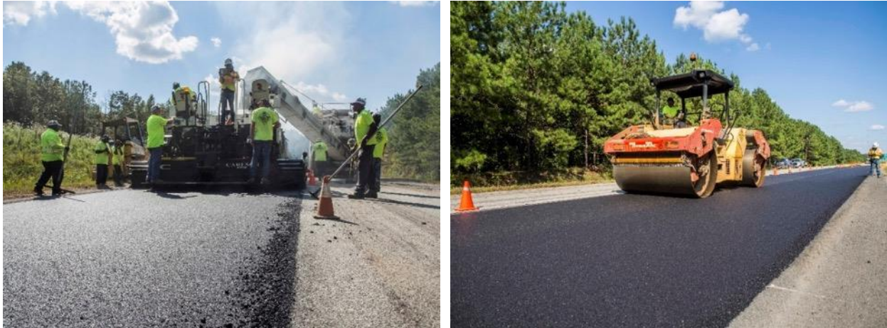
Figure 7. Construction of the Surface Layer of Section S1
