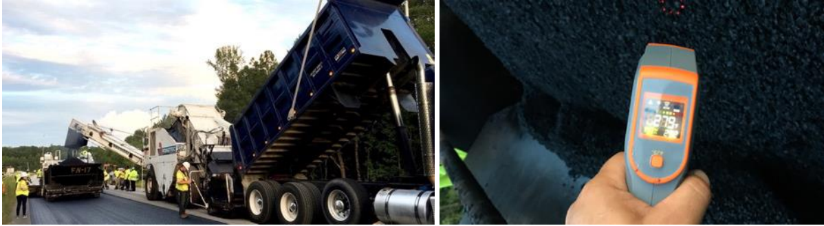
Figure 10. Paving of Section N3A and N3B
