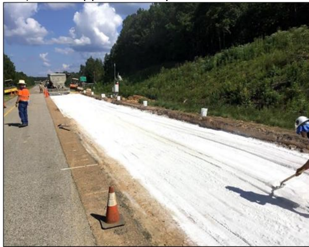
b) Lime Applied by Drop Spreader
