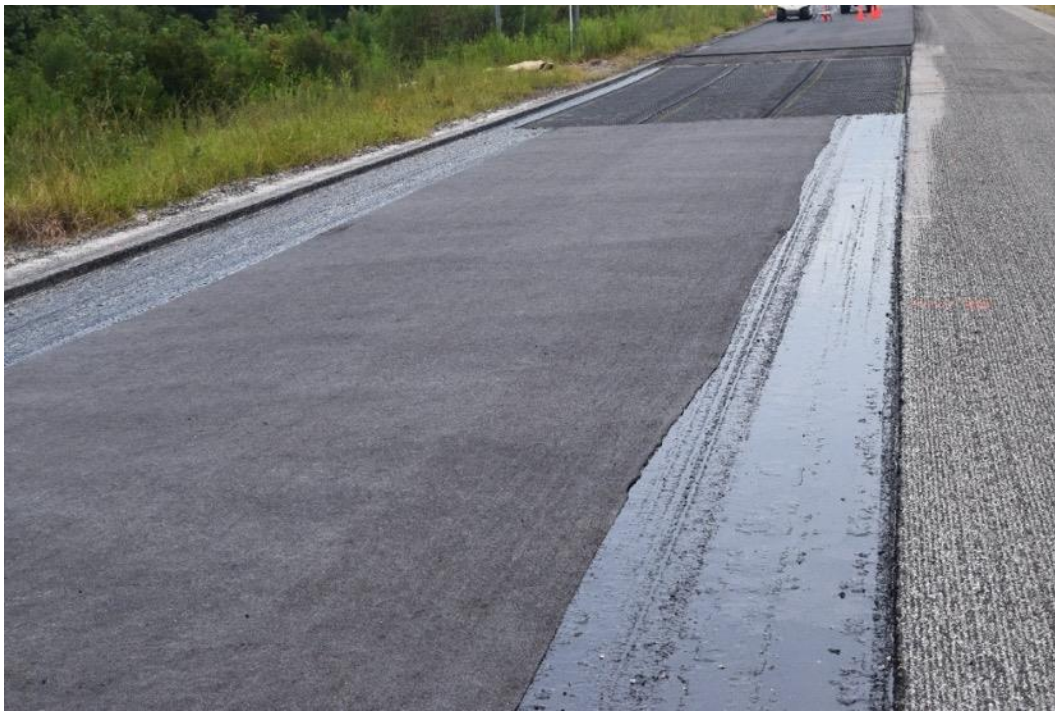
Figure 3. Geosynthetic Interlayers
