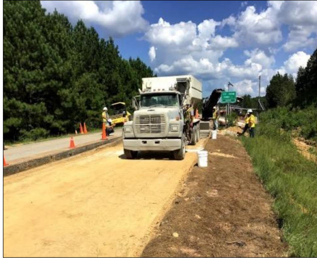
a) Mississippi Soil Ready for Lime Treatment
