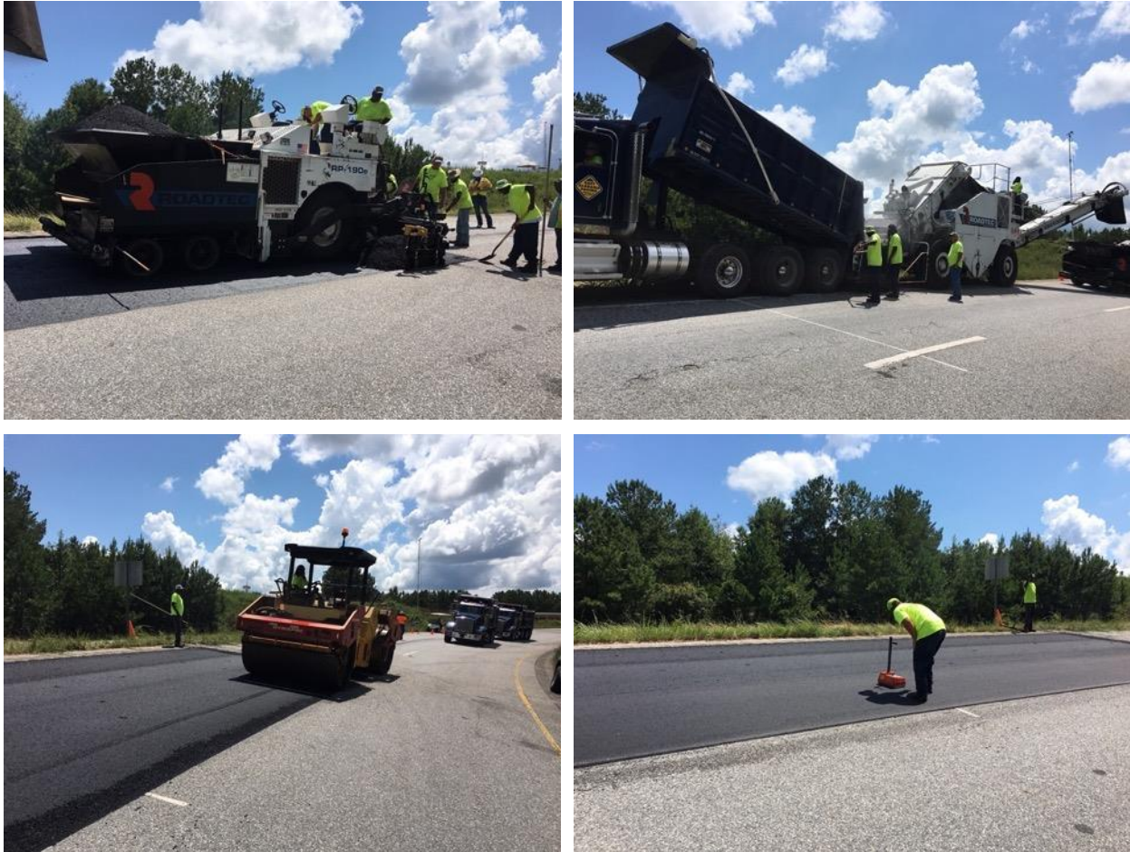
Figure 5. Equipment Utilized During Construction
