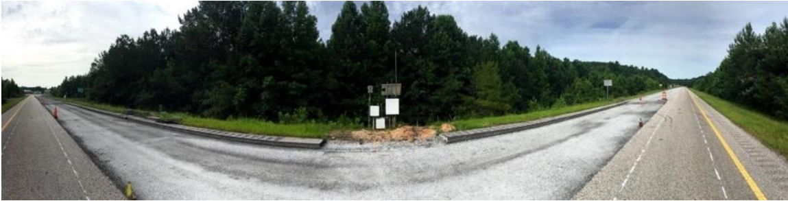
Figure 1. Section S9 Prior to Paving
