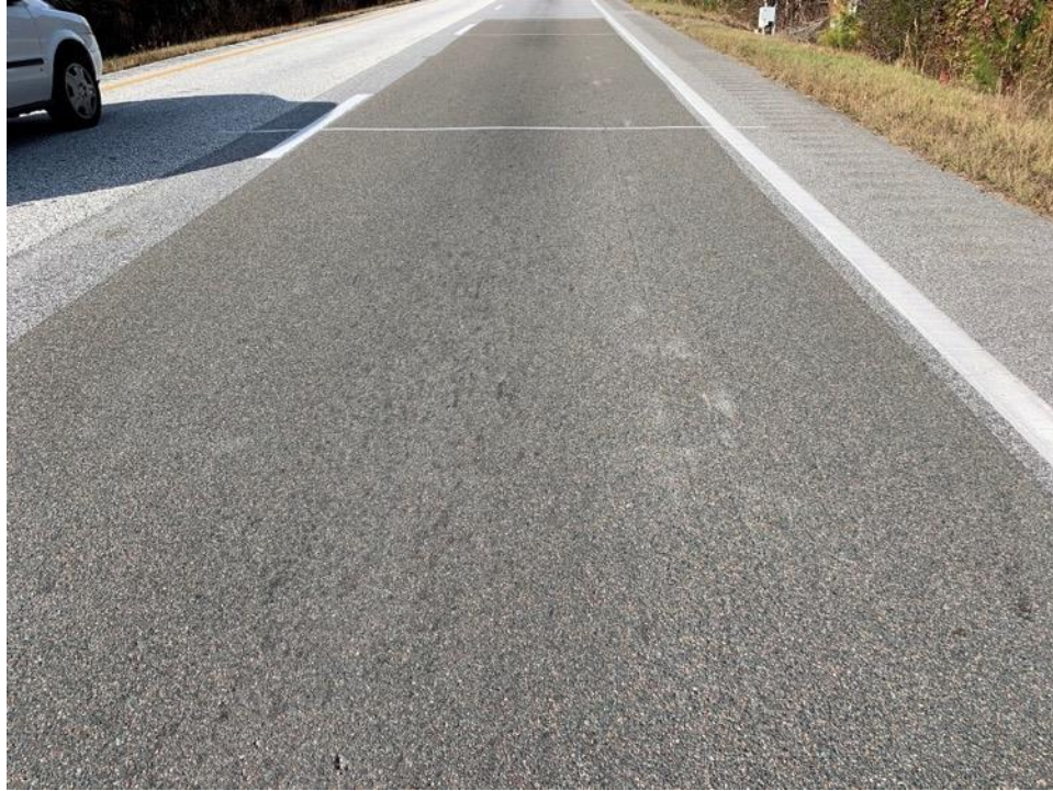
Figure 11. Overview of Micro Surfacing Test Section
