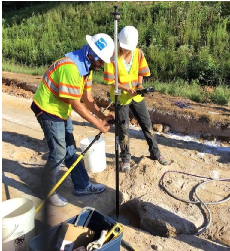
Figure 5. Installation of First EPC Below Lime Treated Soil in Section S2
