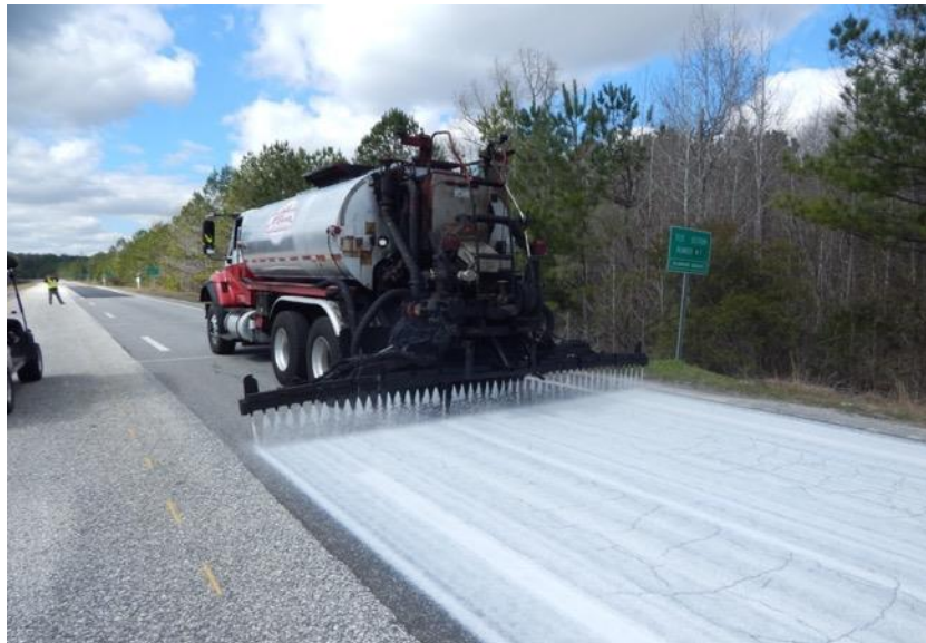
Figure 6. Delta Mist Application on Section N7 in February 2020
