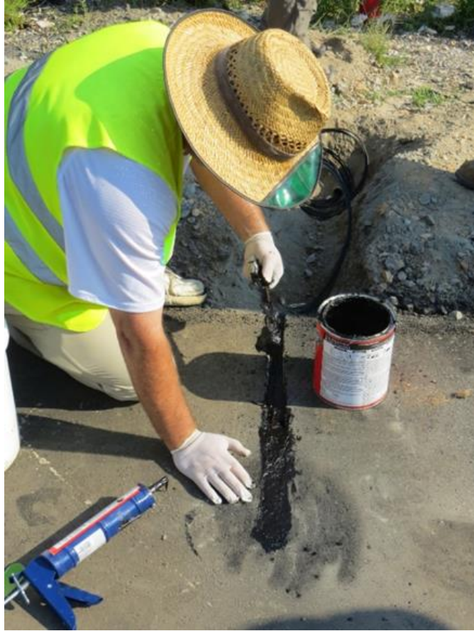
Figure 11. Covering Thermocouple Bundle with Roofing Asphalt
