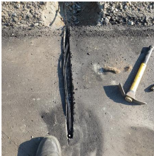
Figure 7. Installed Thermocouple Bundle Prior to Covering with Roofing Asphalt
