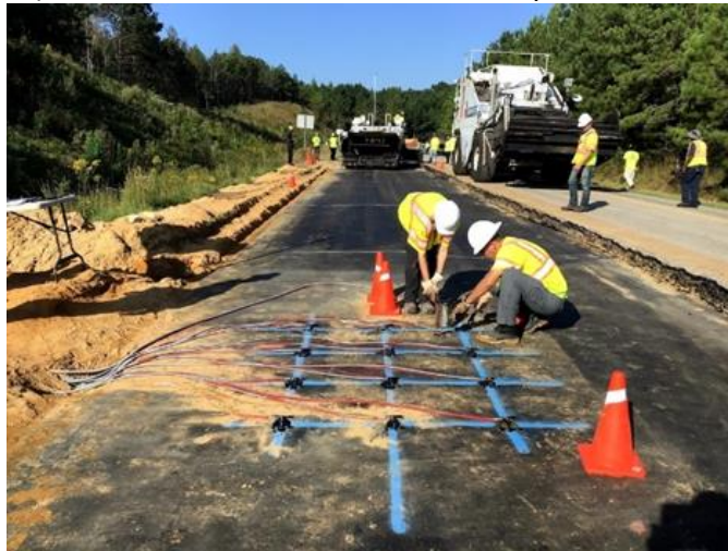
b) ASGs Positioned for Paving
