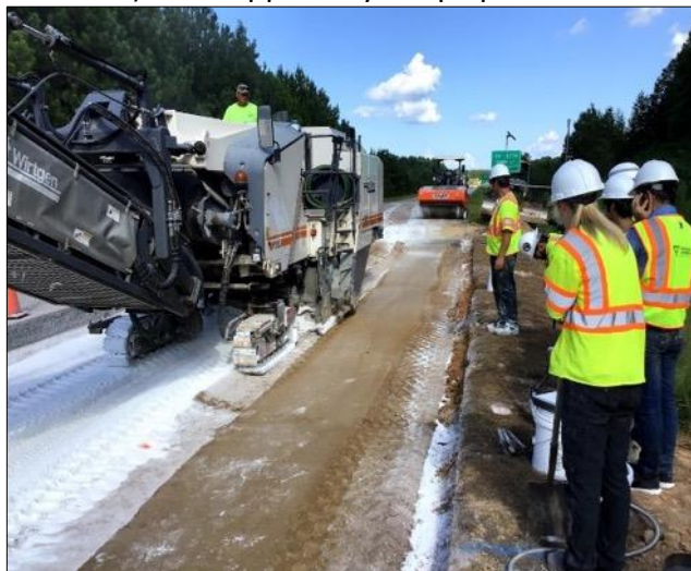
c) Lime Mixing with Milling Machine
