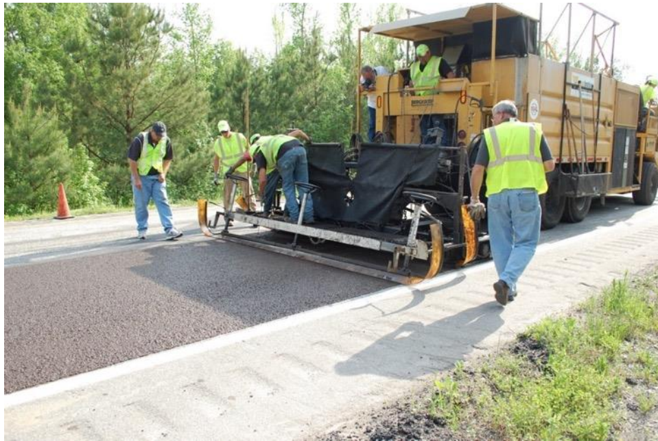
Figure 1. Micro Surfacing Application on Section N6A
