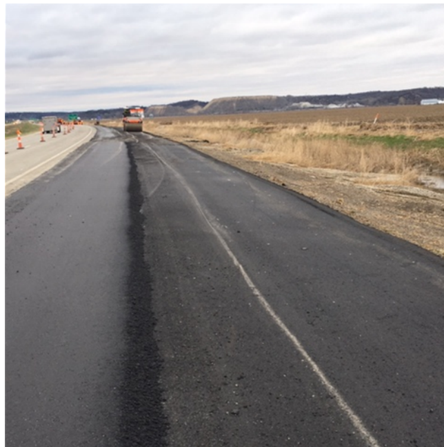
Figure 6. Extended (Additional) Shoulder as Temporary Flood Mitigation Technique in Case Additional Flooding Occurred Before Geogrid Mats Were Installed
