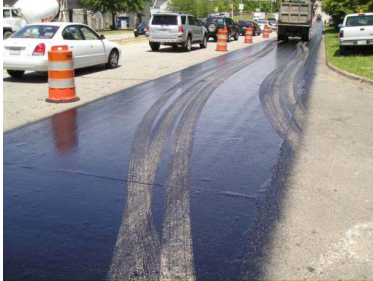
Figure 15. Tracking Problem with Typical Distributor (West et al., 2005)
