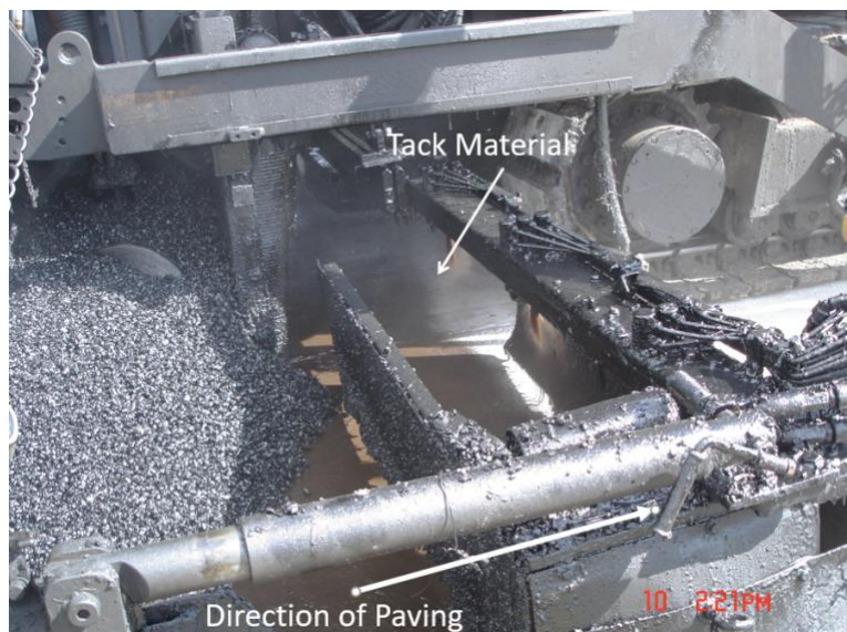
Figure 16. Tack Coat Application Using Spray Paver (Mohammad et al., 2012)
