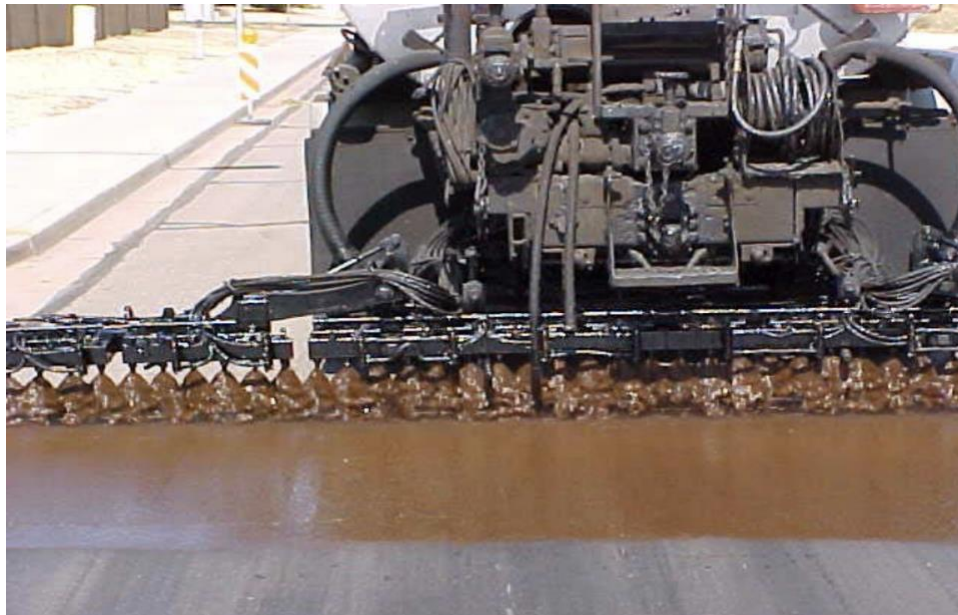
Figure 11. Tack Coat Application (Simpson, 2006)
