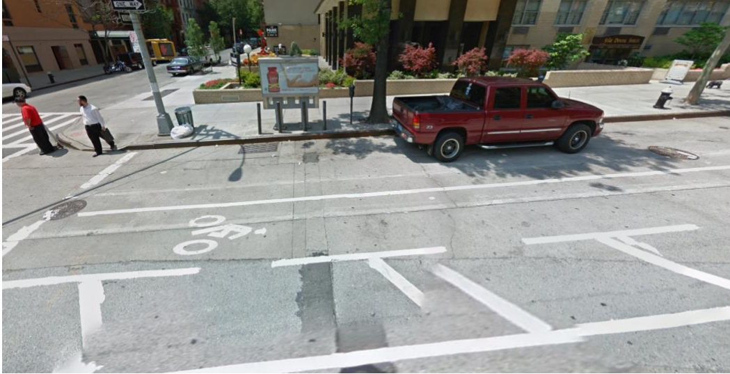
Figure 10. Tie-ins to Curb and Gutter and Drainage Inlets, 1 st Avenue, New York City
