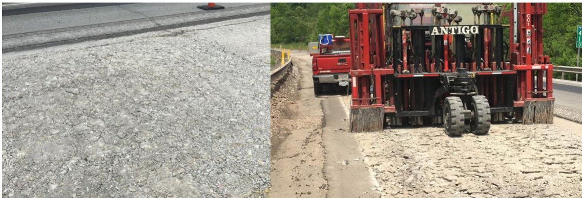
Figure 6. Rubblized PCC Pavement Surface, I-79 West Virginia
