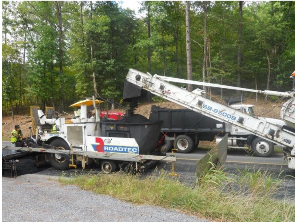
Figure 46 MTV Transferring Mix to Paver on AL 35
