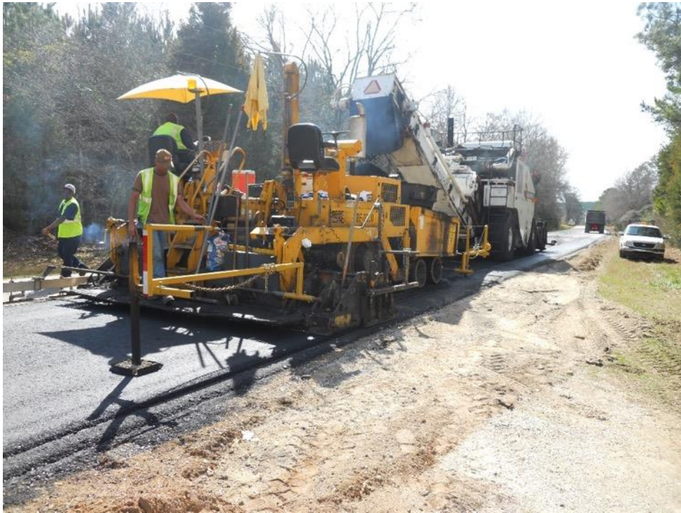
Figure 25 MTV Transferring Mix to Paver on AL 50
