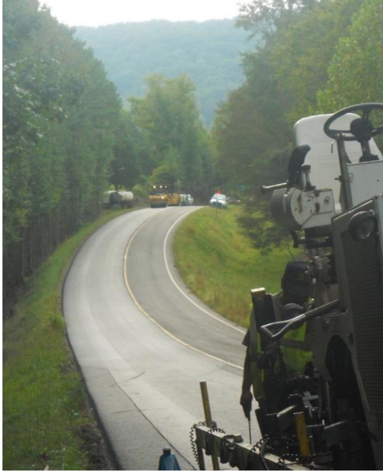
Figure 47 Roller Compacting on AL 35
