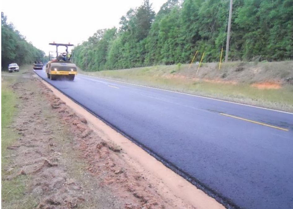
Figure 38 Breakdown and Finishing Rollers Operating on AL 137
