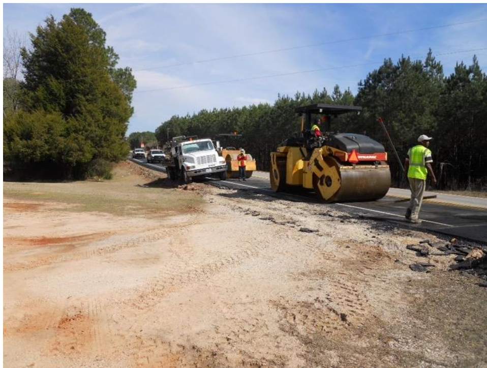
Figure 26 Breakdown and Finishing Rollers Used on AL 50
