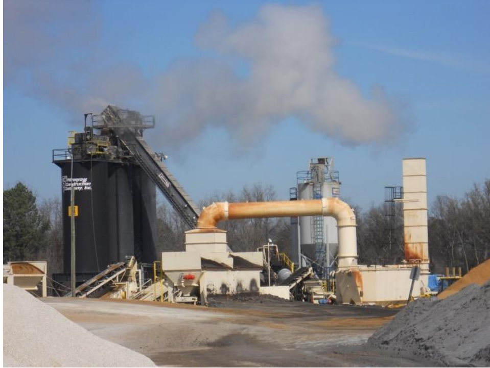
Figure 50 Wiregrass Construction's CMI Plant in Montgomery, Alabama
