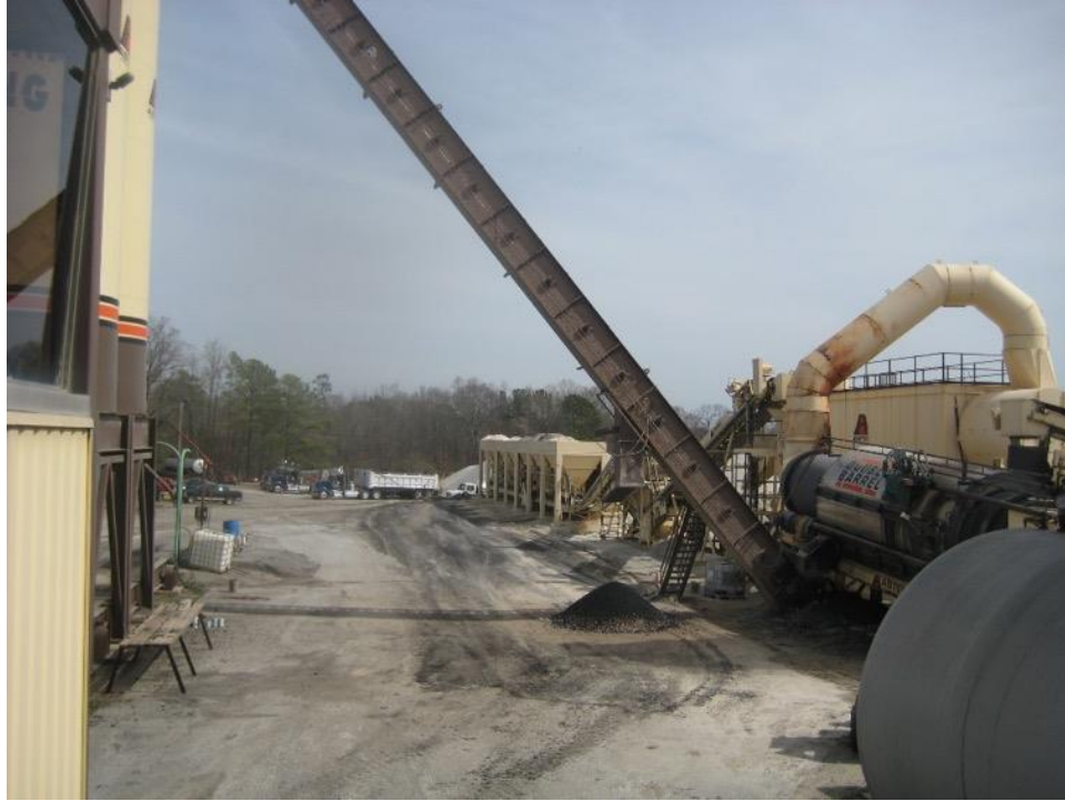
Figure 23 East Alabama Paving's Astec Double Barrel Green Plant
