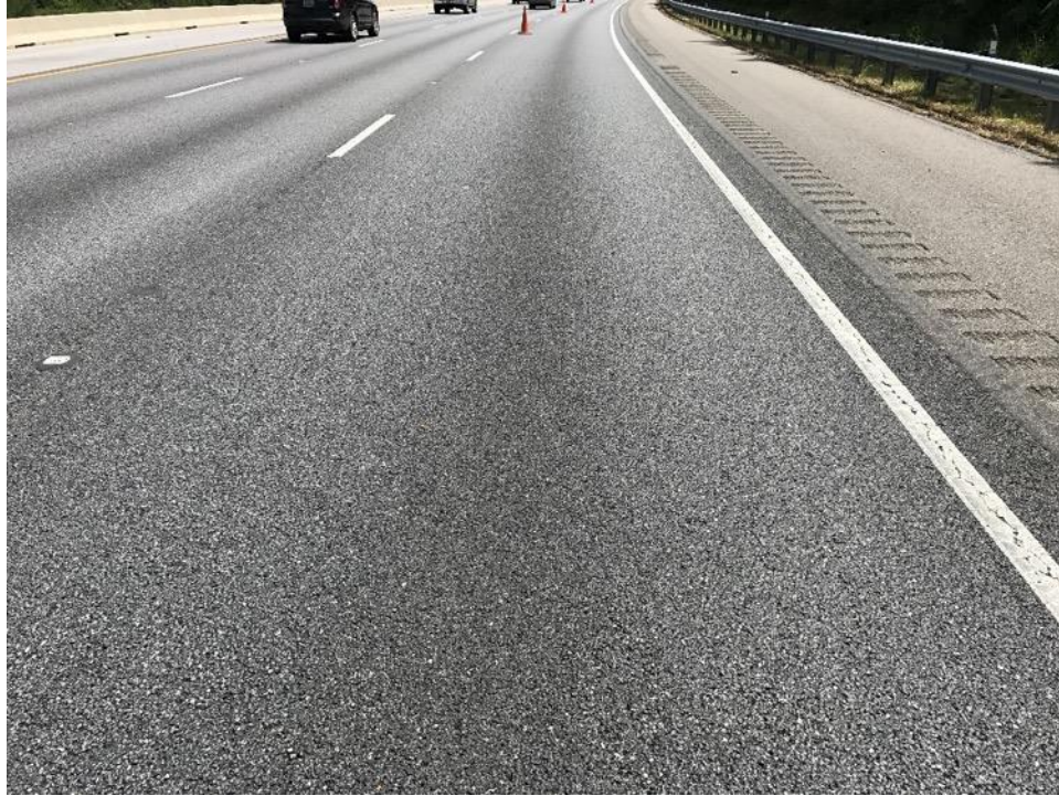
Figure 33 Example of Test Section on I-65
