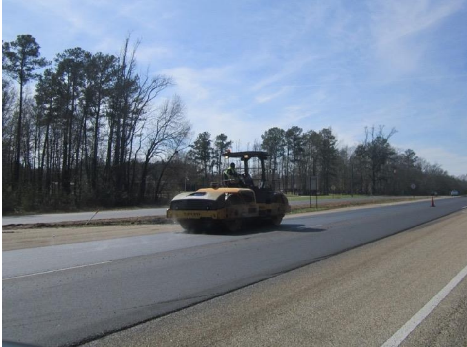
Figure 53 Breakdown Roller Operating on US 80
