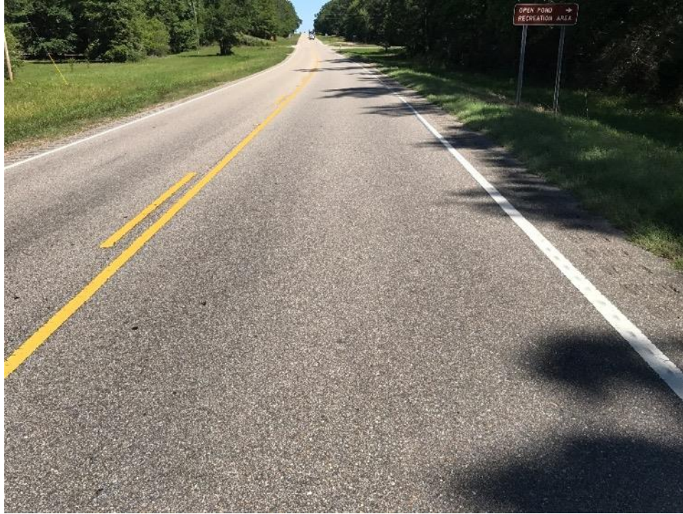
Figure 39 Example of Test Section on AL 137
