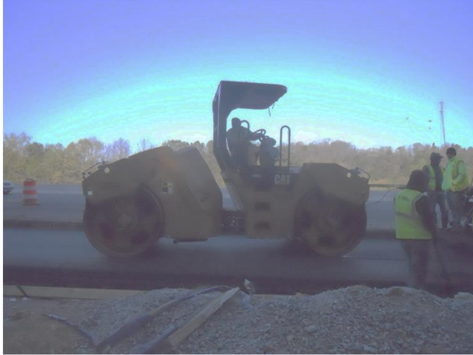
Figure 32 Breakdown Roller Used on I-65
