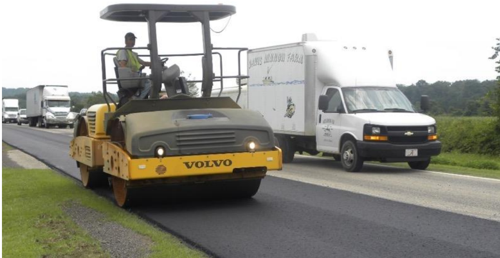
Figure 42 Breakdown Roller Operating on US 29
