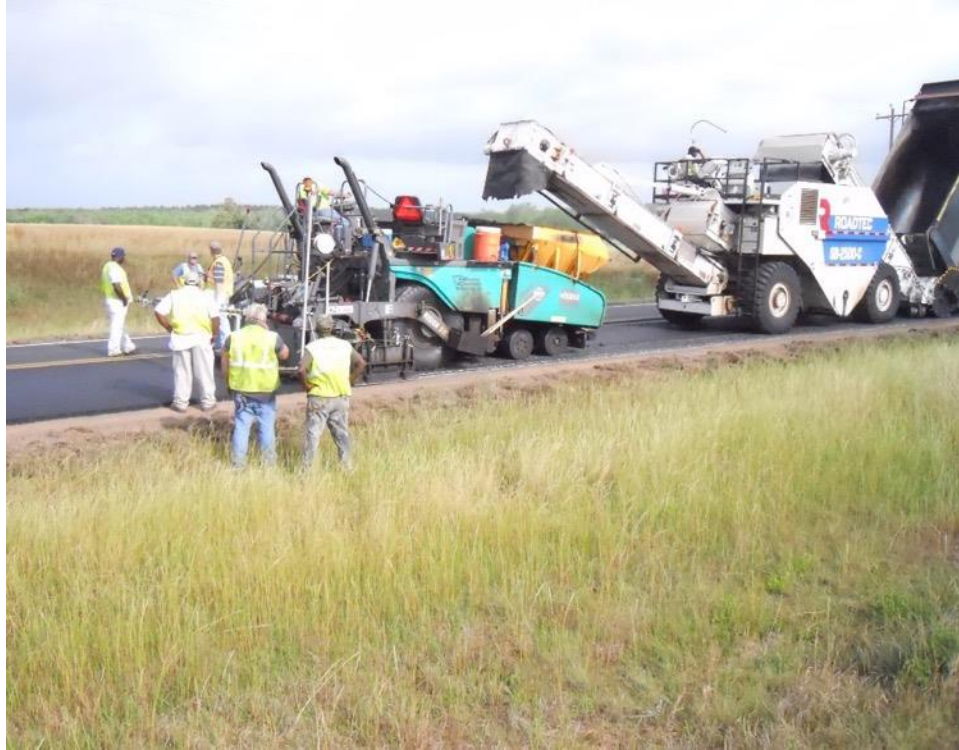
Figure 37 MTV Transferring Mix to Paver on AL 137
