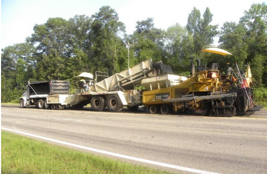
Figure 41 MTV Transferring Mix to Paver on US 29
