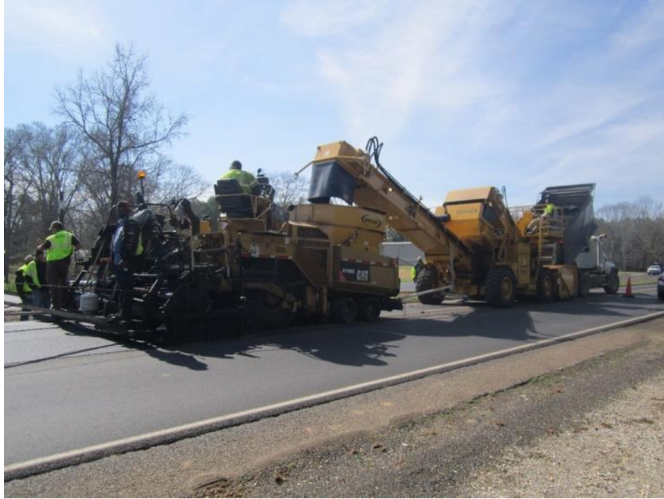
Figure 52 MTV Transferring Mix to Paver on US 80
