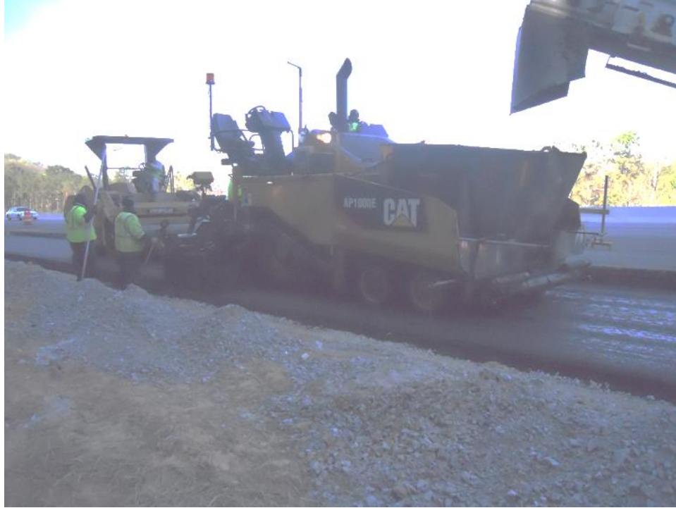
Figure 31 MTV Transferring Mix to Paver on I-65
