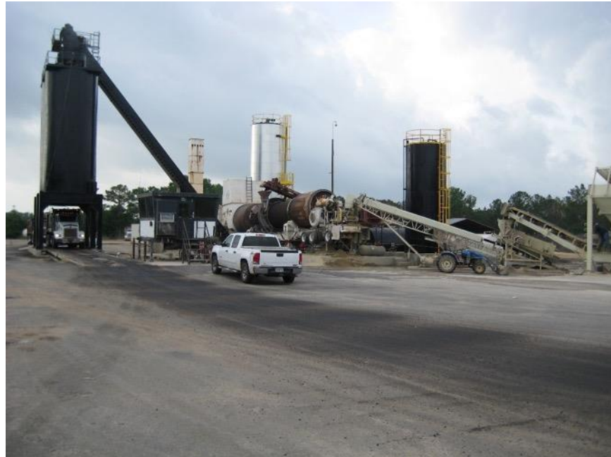
Figure 34 Wiregrass Construction’s CMI Plant in Brantley, Alabama
