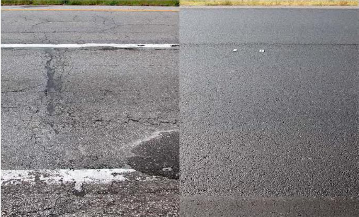
FIGURE 17 Close-up of pavements before and after resurfacing (29)
