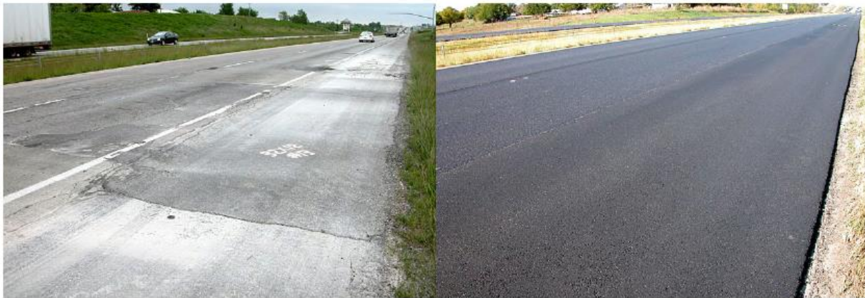
FIGURE 16 Interstate 70 pavements before and after pavement resurfacing (29)
