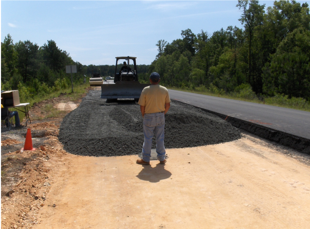
Figure 3.5 Subgrade and Aggregate Base
