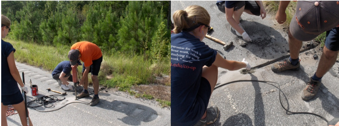
a) Drilling hole for temp probe
