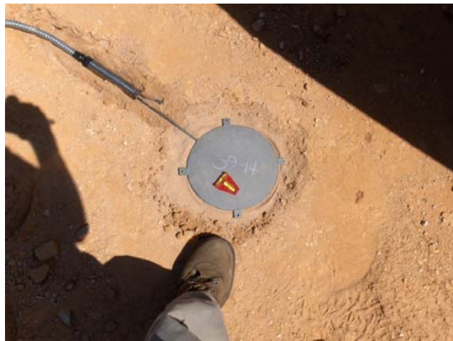
Figure 3.3 Subgrade Earth Pressure Cell Installation Prior to Final Covering
