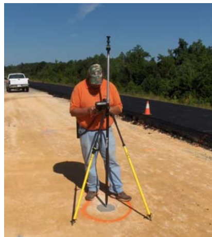
Figure 3.4 Final Survey of Subgrade Earth Pressure Cell
