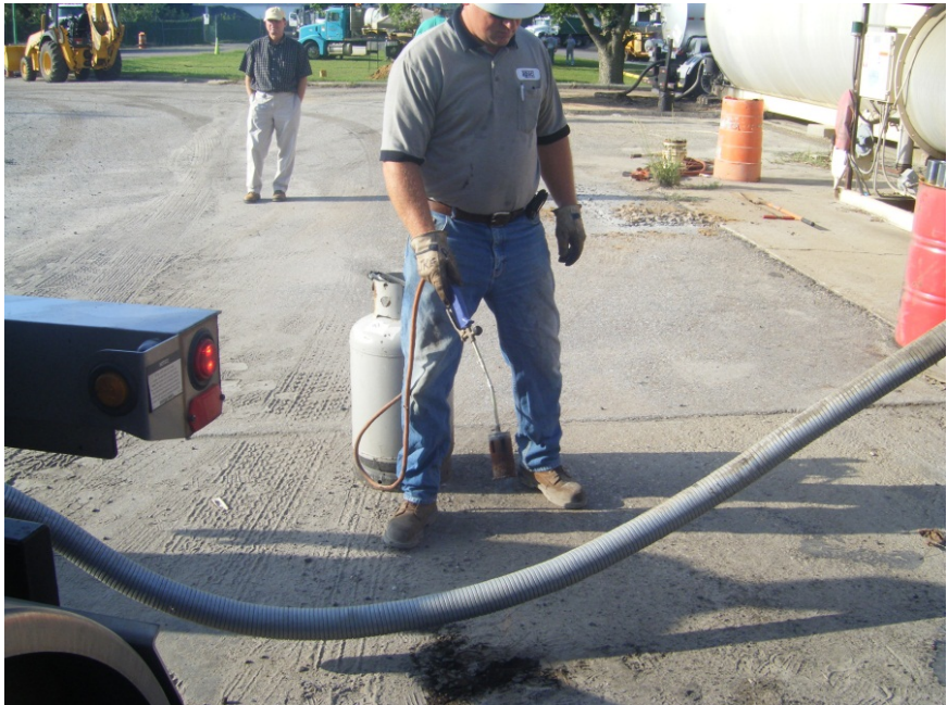
FIGURE 3.2 Rubber-modified binder pumped to plant
