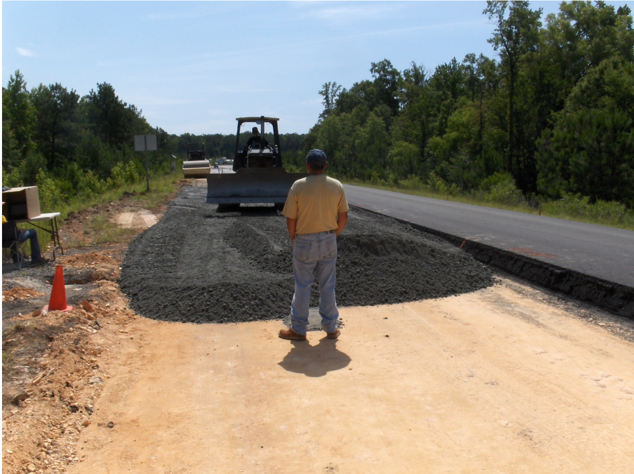
Figure 3.5 Subgrade and Aggregate Base
