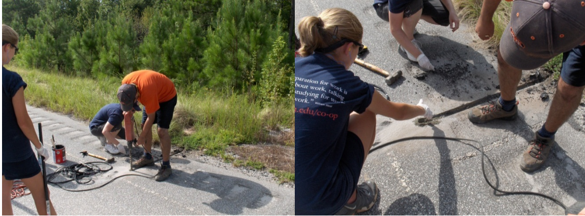
Figure 3.12 Temperature Probe Installation
