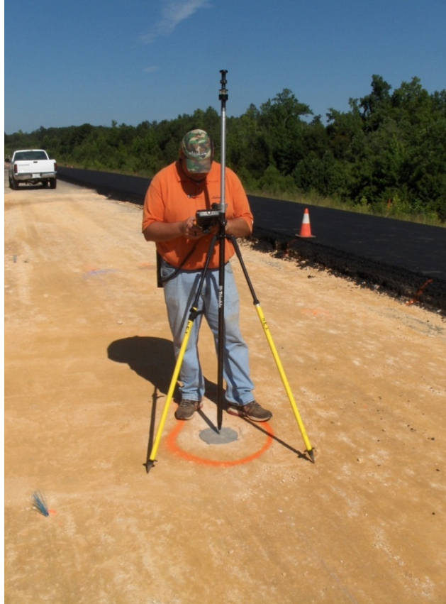
Figure 3.4 Final Survey of Subgrade Earth Pressure Cell
