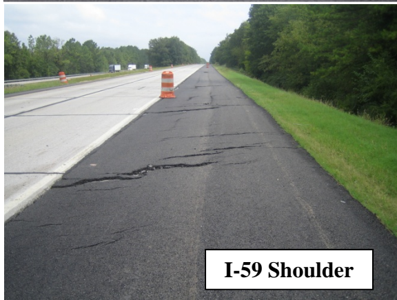
FIGURE 25 Some Pavement Sections Showing Slippage Failures Evaluated in this Study.
