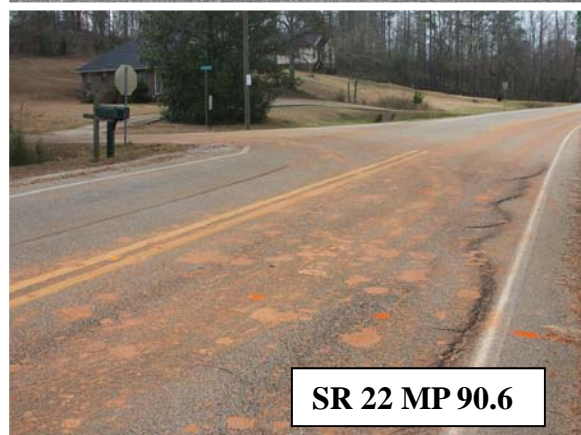
FIGURE 25 Some Pavement Sections Showing Slippage Failures Evaluated in this Study.
