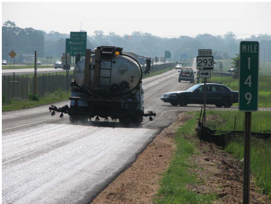
FIGURE 7 Tack Coat Application.
