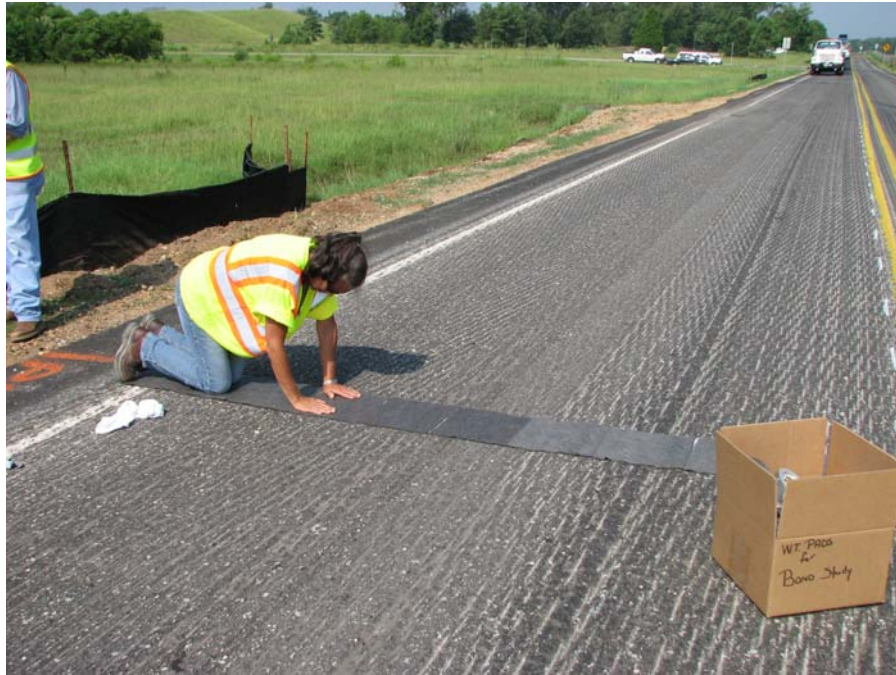
FIGURE 41 Installing Geotextile Pads for Measuring Application Rate.
