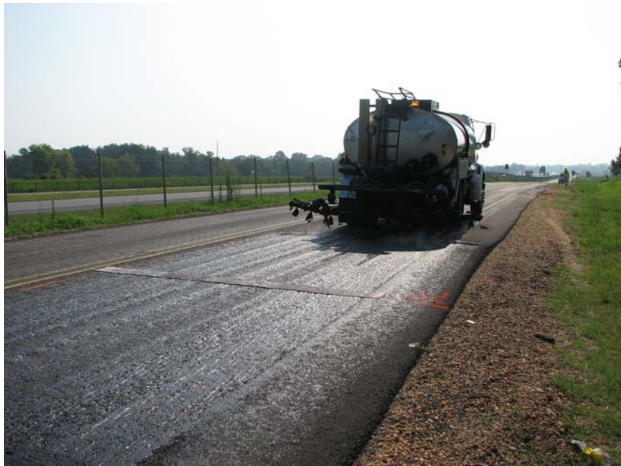
FIGURE 42 Installing Geotextile Pads for Measuring Application Rate.
