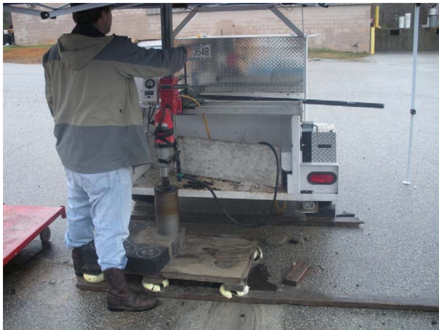
FIGURE 30 Cutting Cores from Slab.
