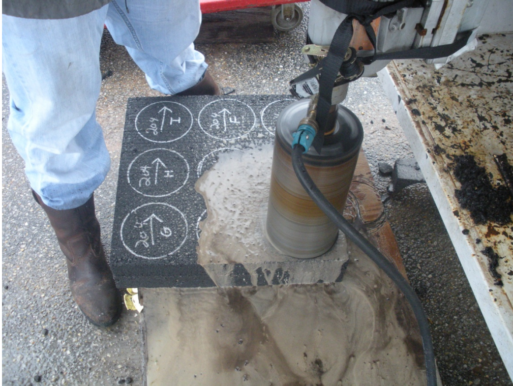
Figure 21 Coring of Slabs
