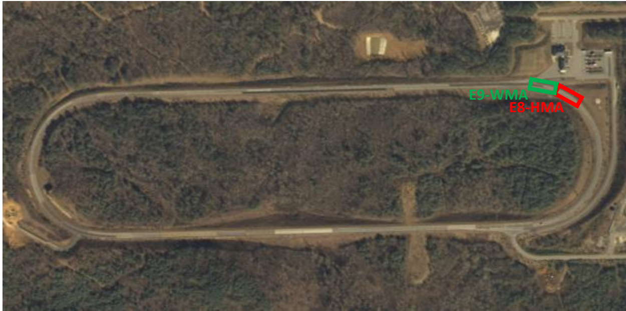
FIGURE 7 Location of Study Sections on the NCAT Pavement Test Track
