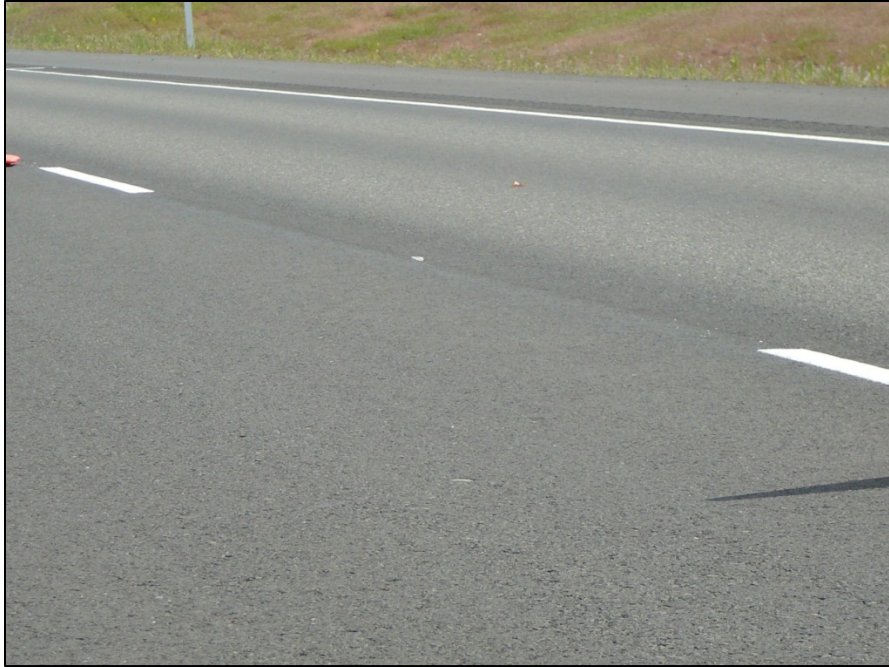
Figure 24 WMA (Foreground) and HMA (Background) Sections at 13-Month Revisit to Walla Walla, WA
