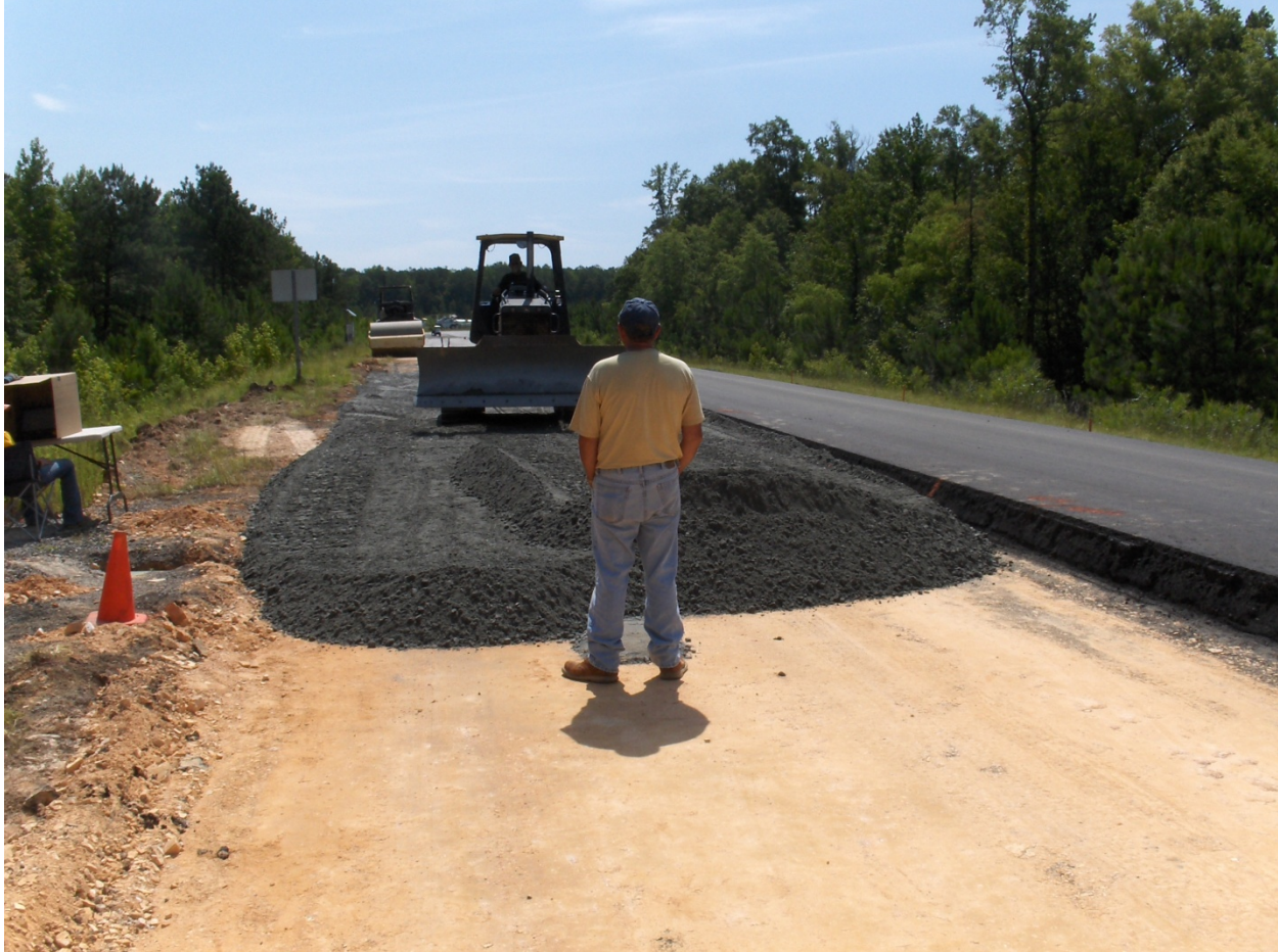
Figure 3.5 Subgrade and Aggregate Base
