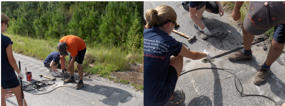
Figure 3.13 Temperature Probe Installation
