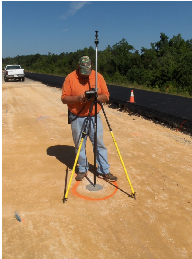
Figure 3.4 Final Survey of Subgrade Earth Pressure Cell
