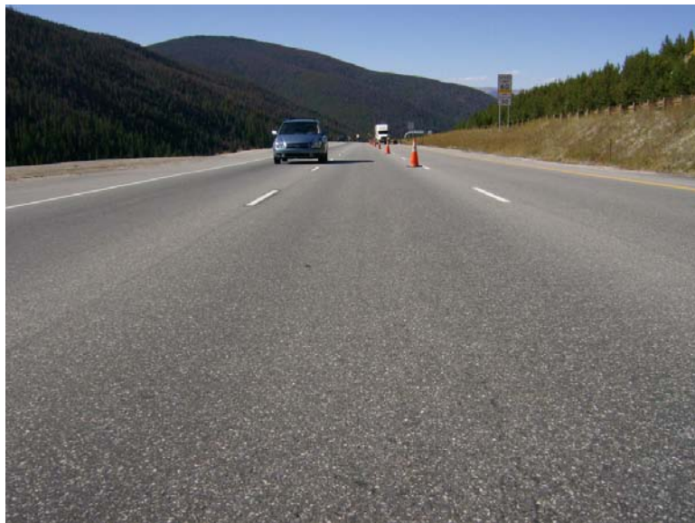
Figure 17 Overall Surface Texture of HMA Control and WMA Test Sections: Excellent Performance
