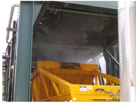
Figure 2 Visible Smoke and Fumes from HMA Production at the Plant
