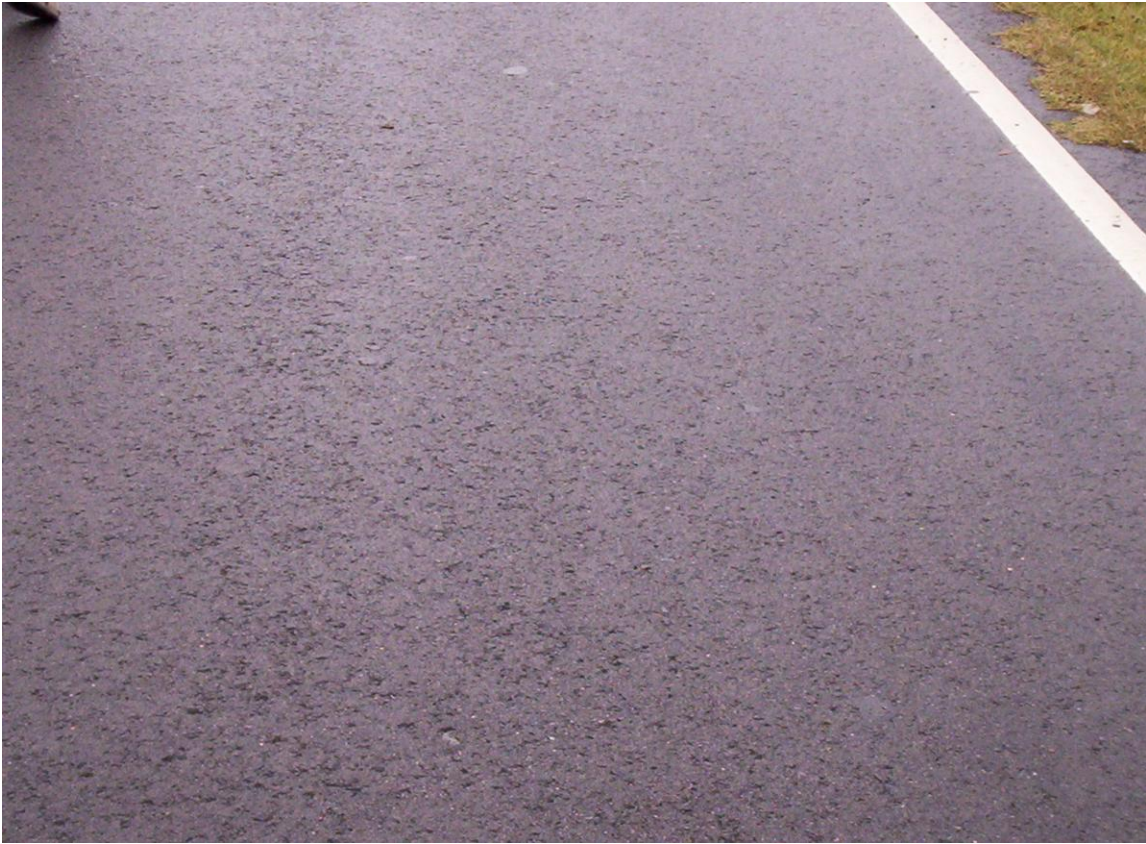
FIGURE 23 HMA 2 Pavement Condition
