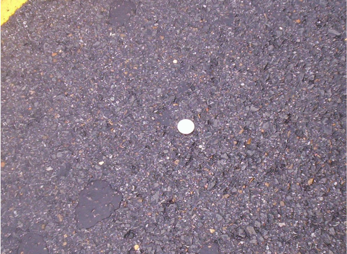
FIGURE 24 HMA 1 Pavement Condition
