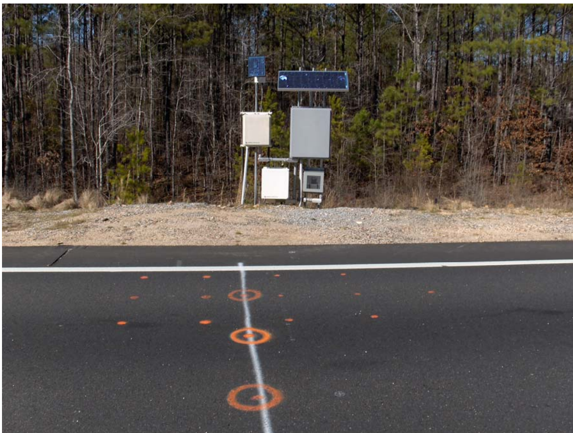
FIGURE 62 Remote roadside boxes.
