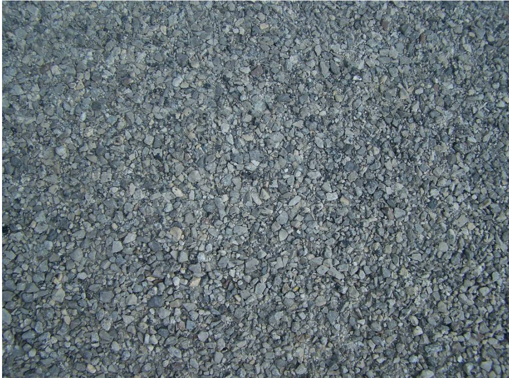
Figure 17. Sasobit® WMA Test Section (20)
