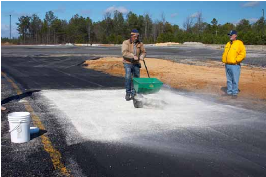
FIGURE 9 Spreading uncoated aggregate for surface gritting.
