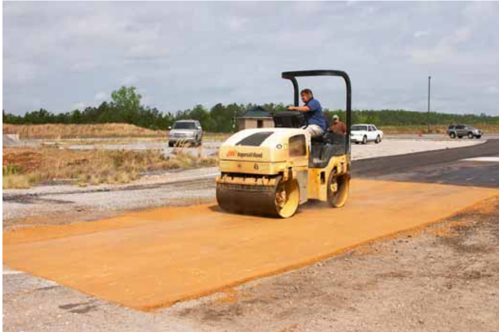
FIGURE 20 Rolling synthetic binder section.
