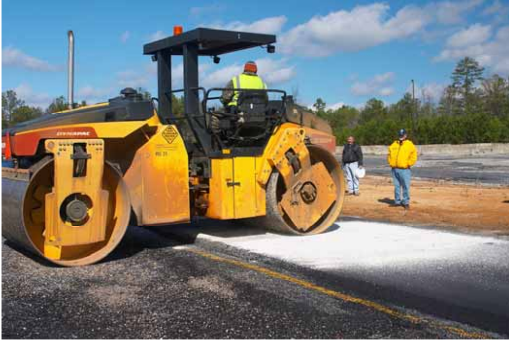
FIGURE 10 Construction of surface gritting section using uncoated aggregate.
