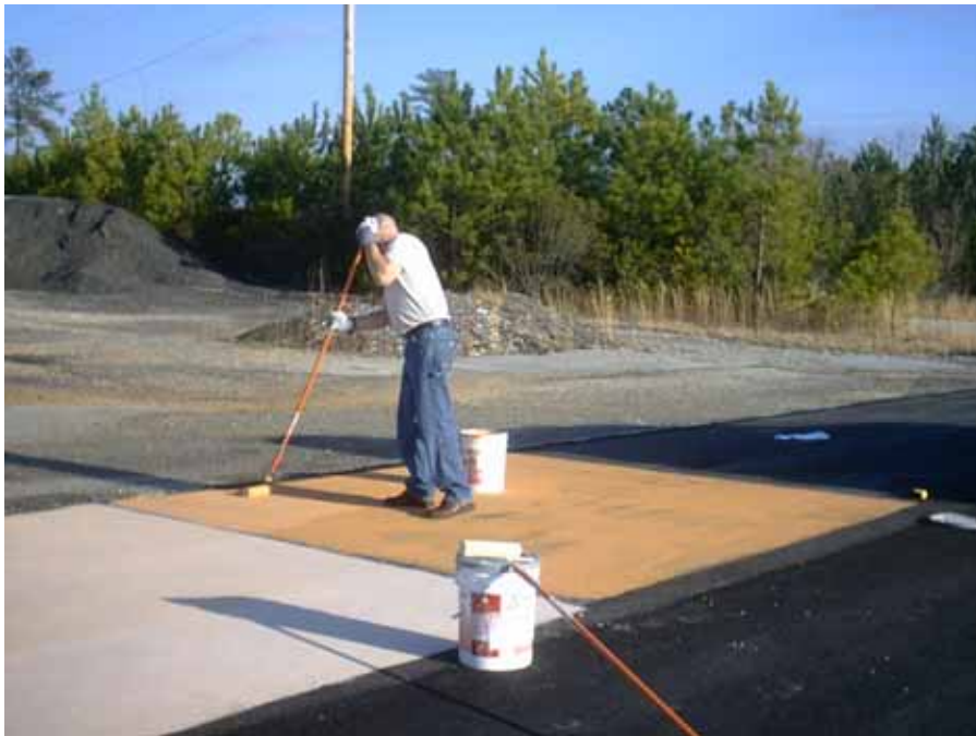
FIGURE 15 Construction of StreetPrint section (Sun-Baked Clay Color).
