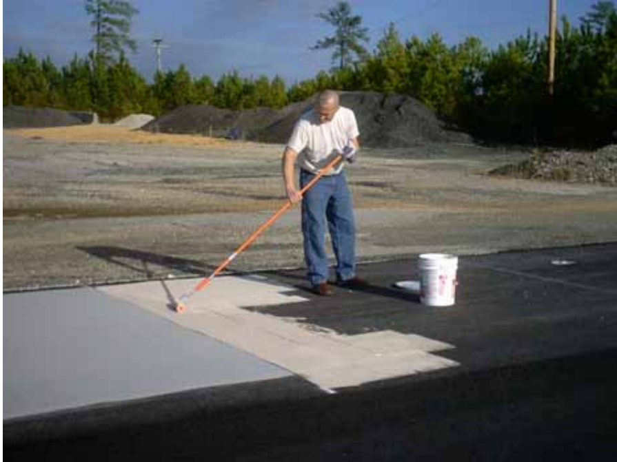
FIGURE 14 Construction of StreetPrint section (Irish Cream Color).
