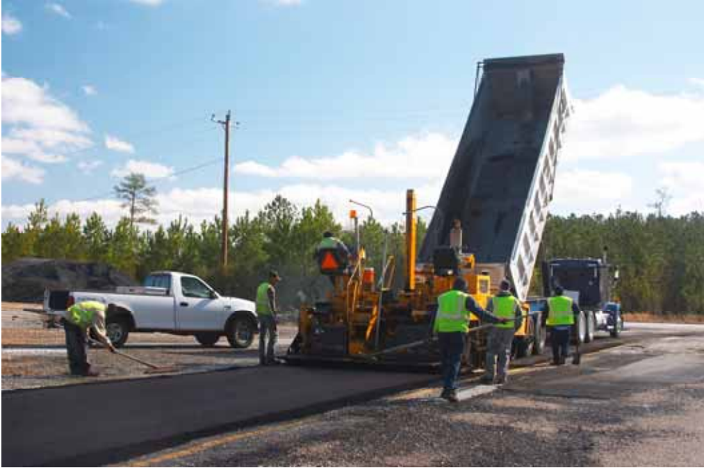
FIGURE 8 Construction of HMA test strip.
