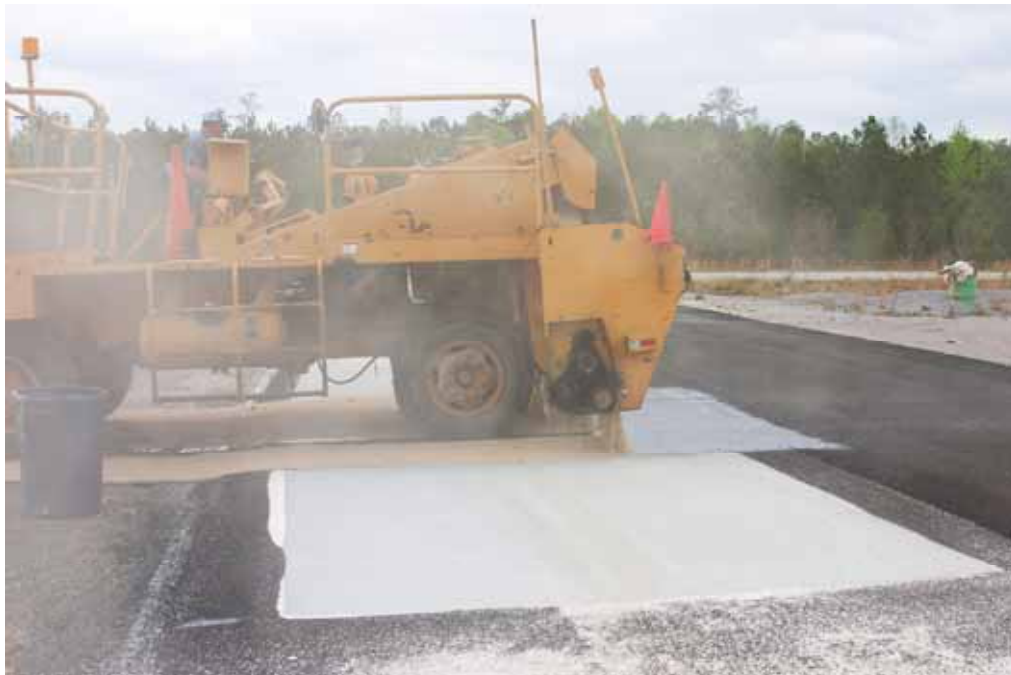
FIGURE 21 Installing chip and sand seals sections.
