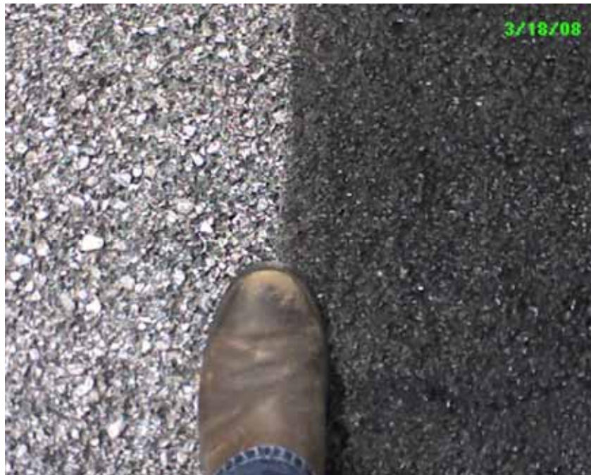
FIGURE 17 Before and after shot blasting.
