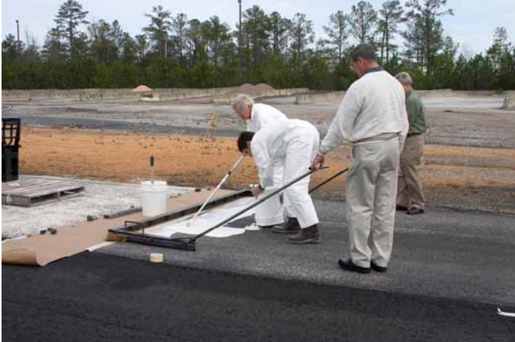
FIGURE 12 Construction of PolyCon section (without coarse sand).
