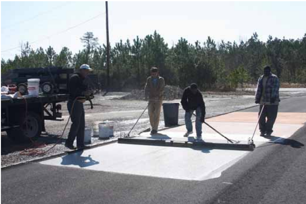
FIGURE 13 Construction of PolyCon section (with coarse sand on top).
