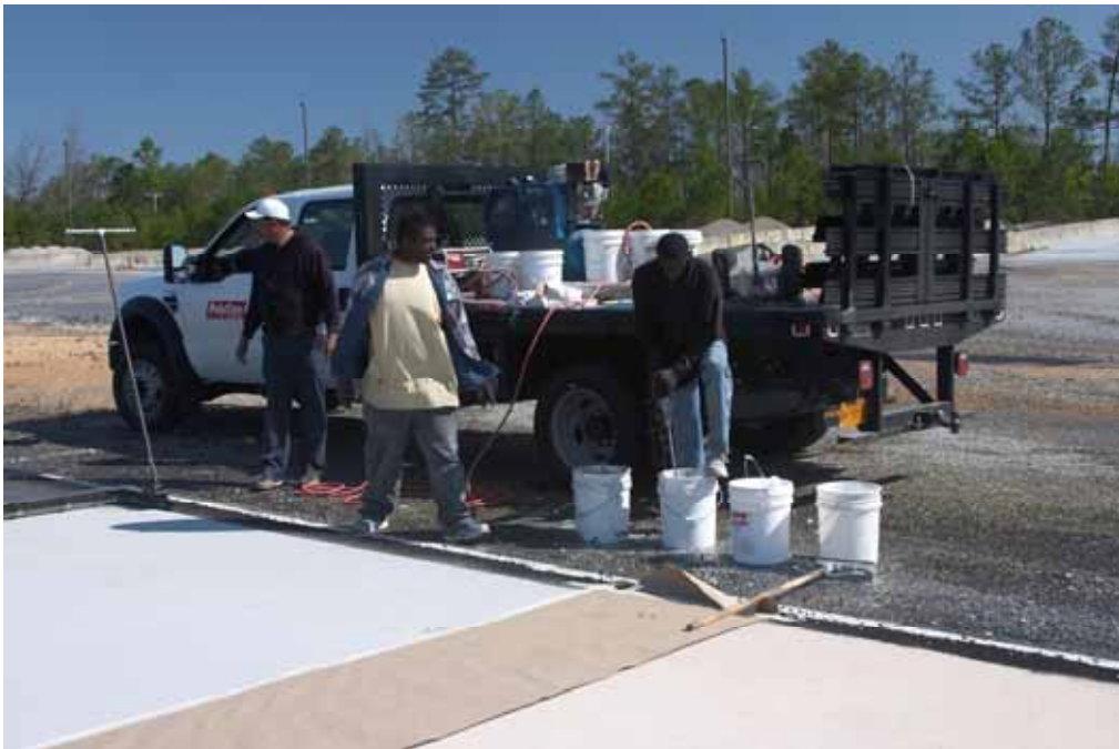
FIGURE 11 Mixing PolyCon materials.
