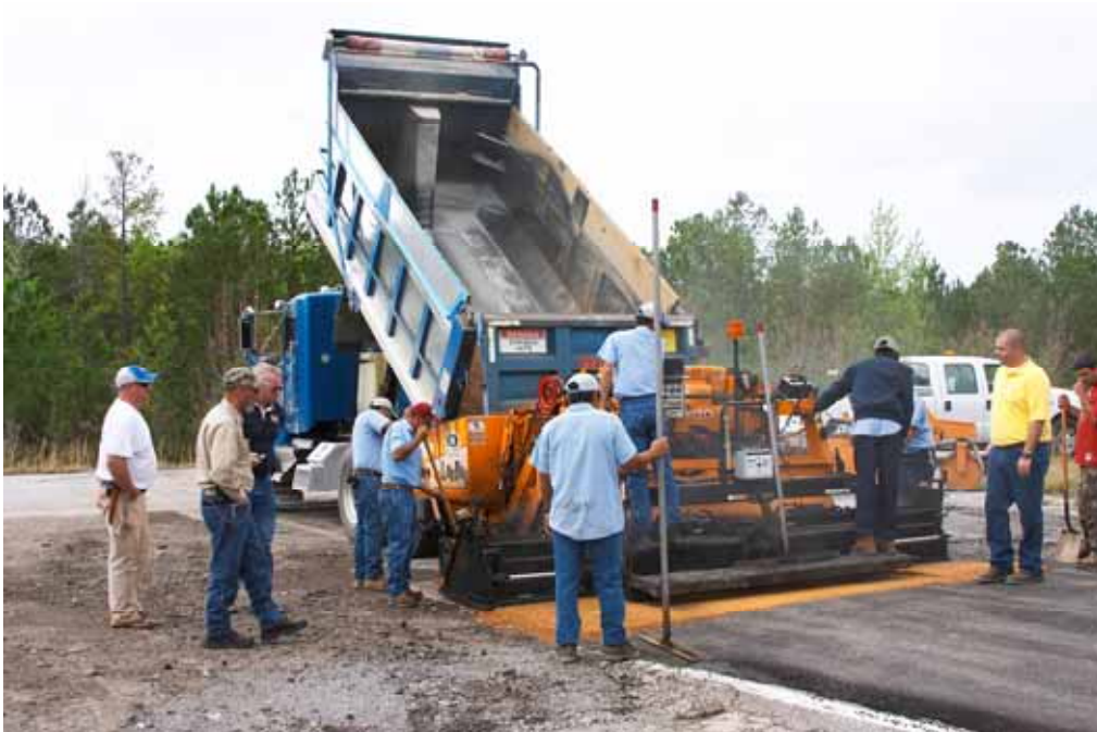
FIGURE 19 Placing synthetic binder section.
