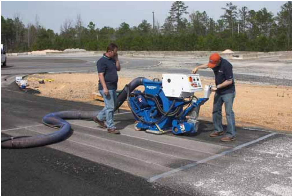
FIGURE 16 Shot blasting by Blastrac.
