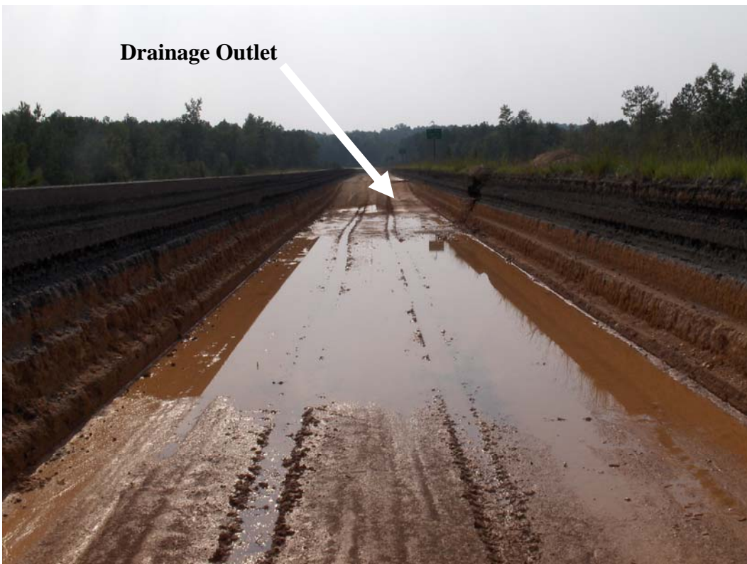
Figure 4.3. Section N9 After a Rain Event (8/24/2006)
