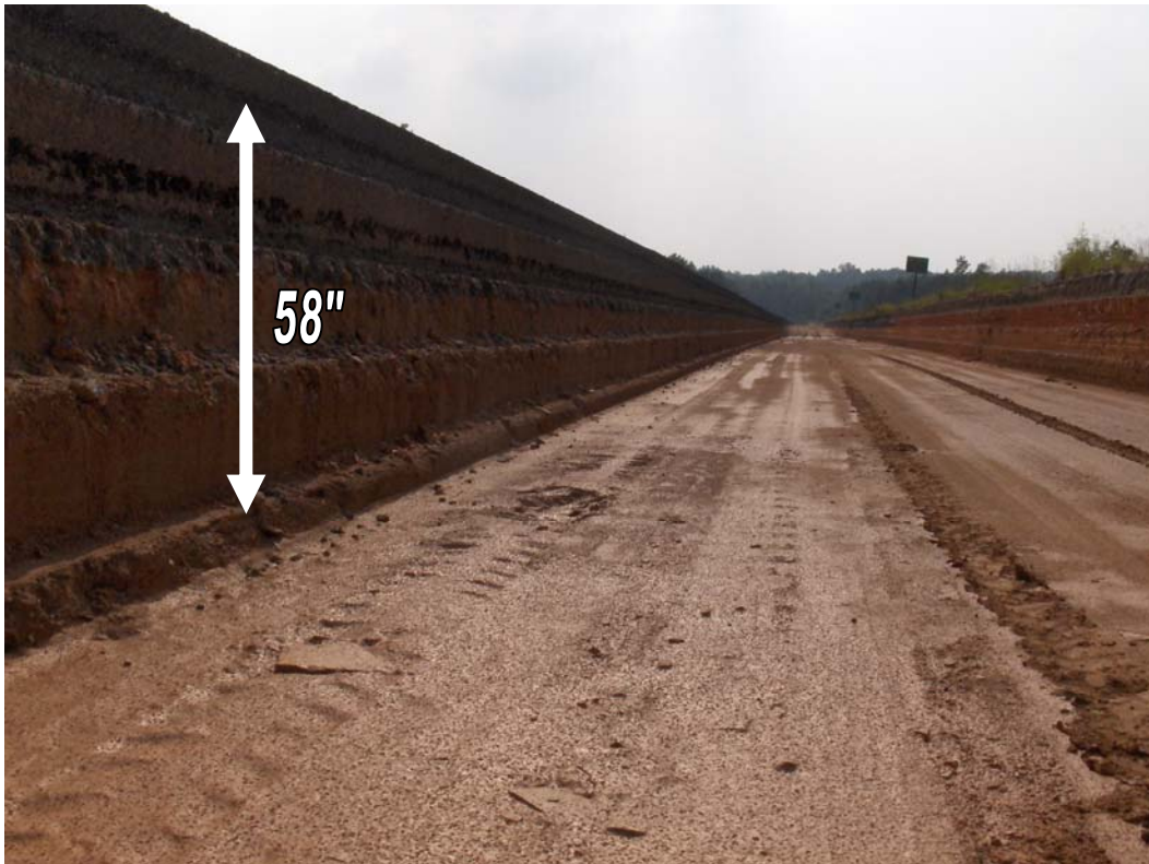
Figure 4.2. Section N8 at Conclusion of Pavement Removal (8/24/2006)
