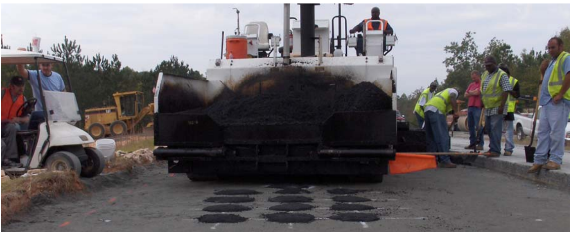
Figure 4.20. Paver Approaching Gauge Array (S11)
