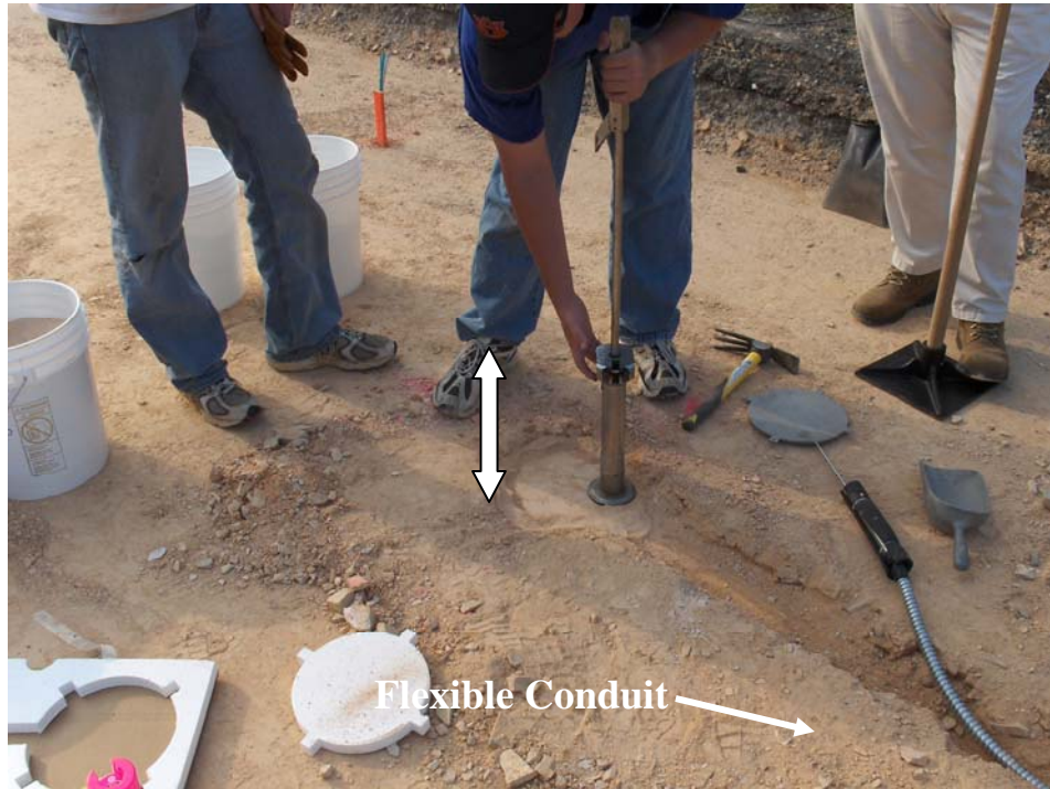
Figure 4.8. Preparation of Pressure Cell Cavity and Trench in N1
