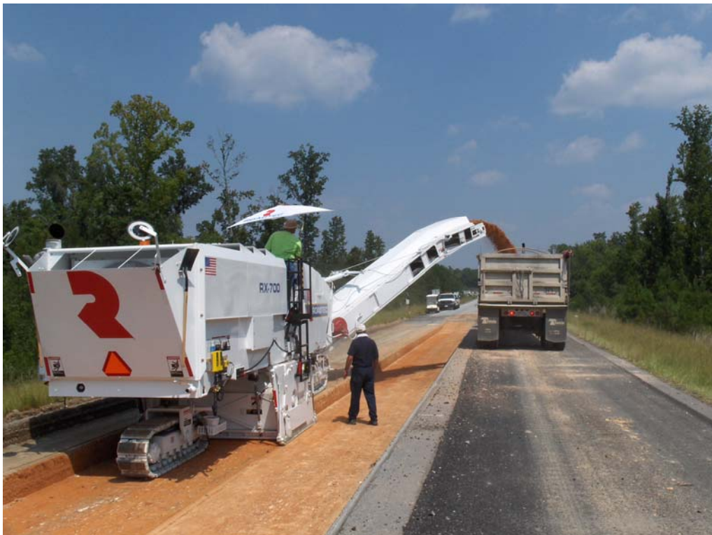
Figure 4.1. Milling Operation in Section N8 (8/18/2006)
