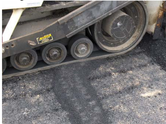
c. Paver Crossing Over Gauge Cables.
