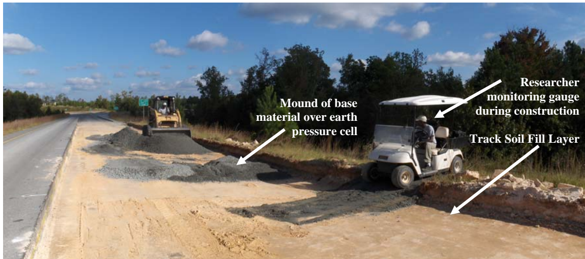
Figure 4.11 Placing Aggregate Base in Section S11.
