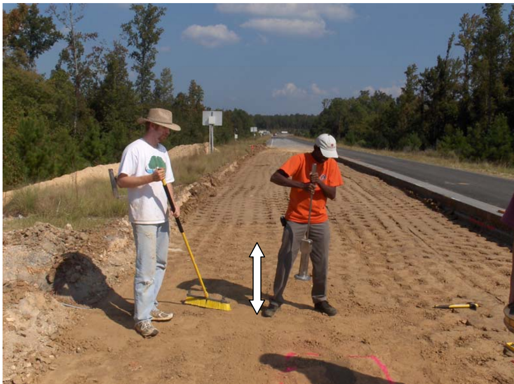
Figure 4.10. Compaction of Cable Trench for Fill Pressure Cell in Section N8
