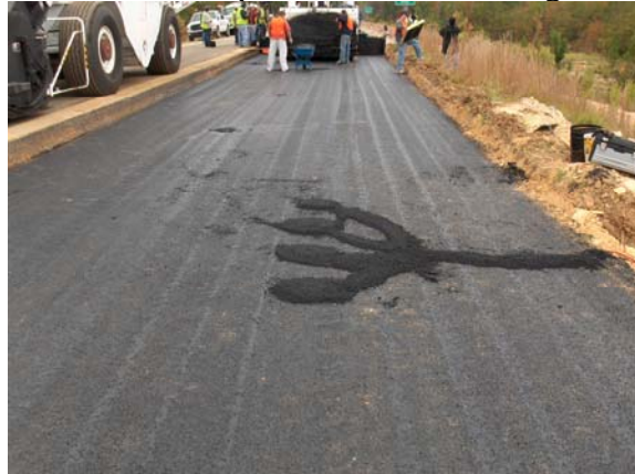
b. Gauges Covered with -#4 Mix Prior to Paving.
