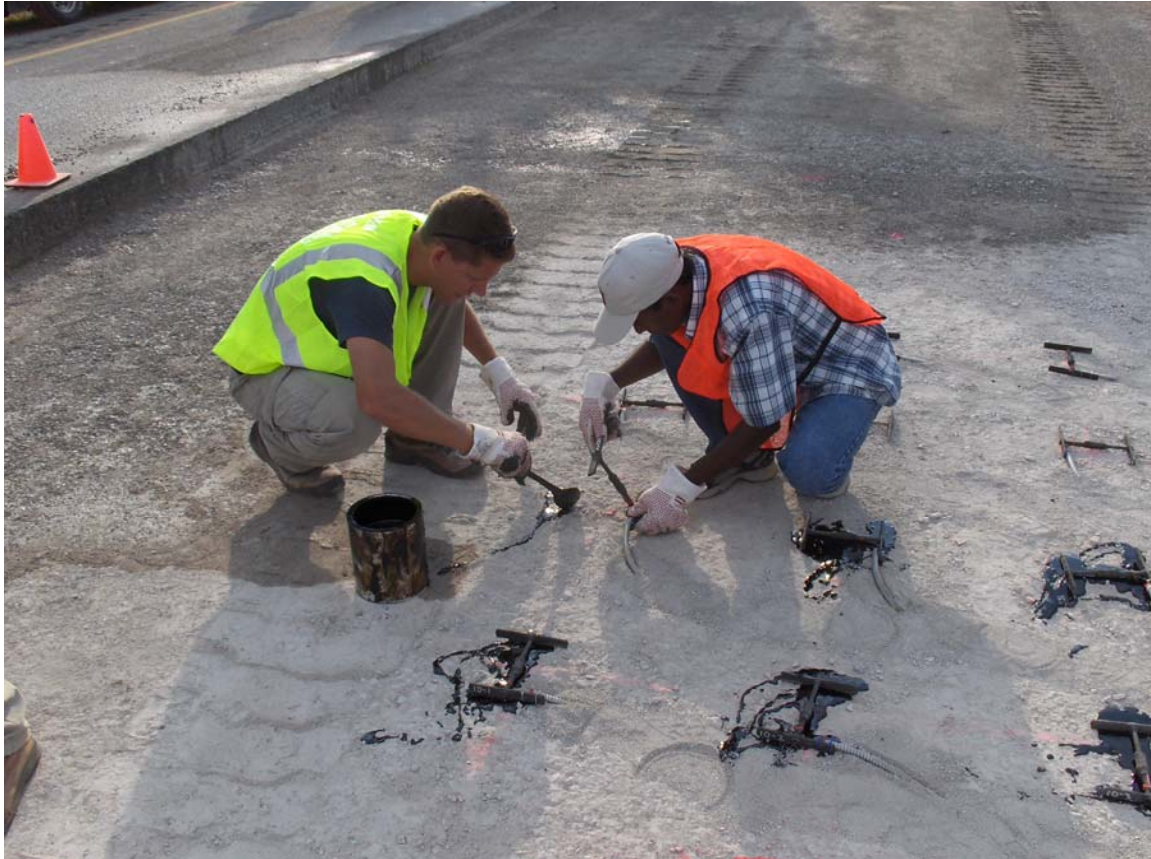
Figure 4.18. Tacking ASGs into Place (N10)
