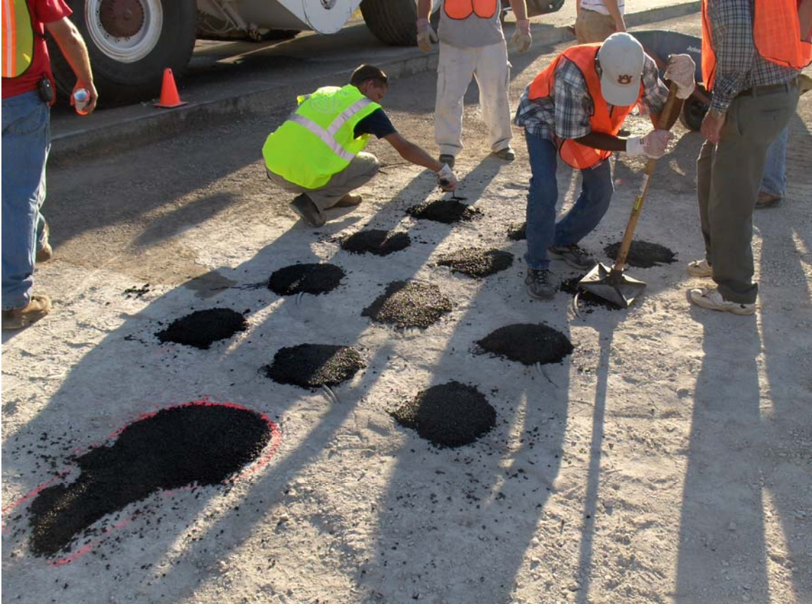
Figure 4.19. Placing Cover Mix (N10)
