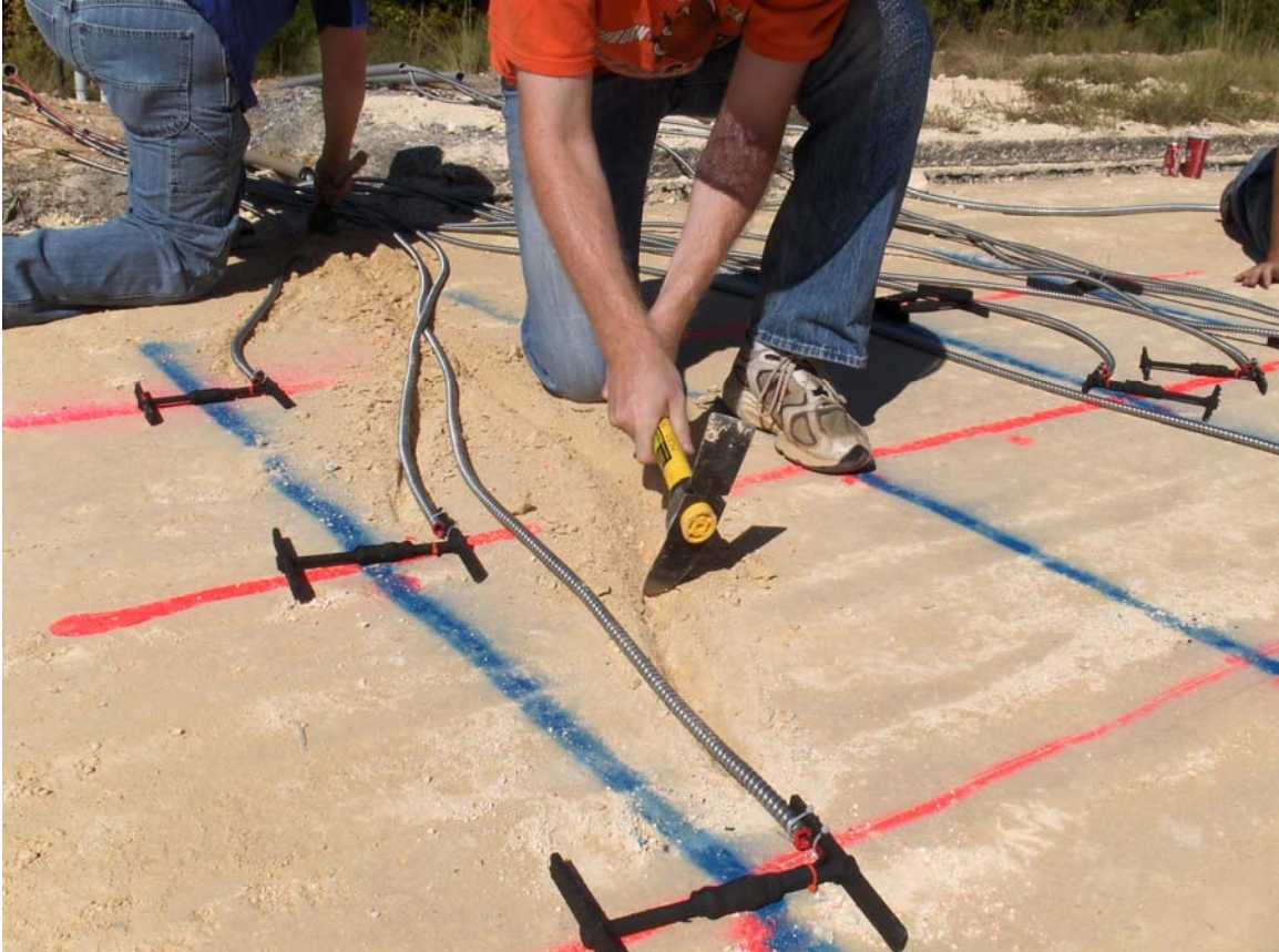
Figure 4.16. Preparing Trenches for Cables in Aggregate Base
