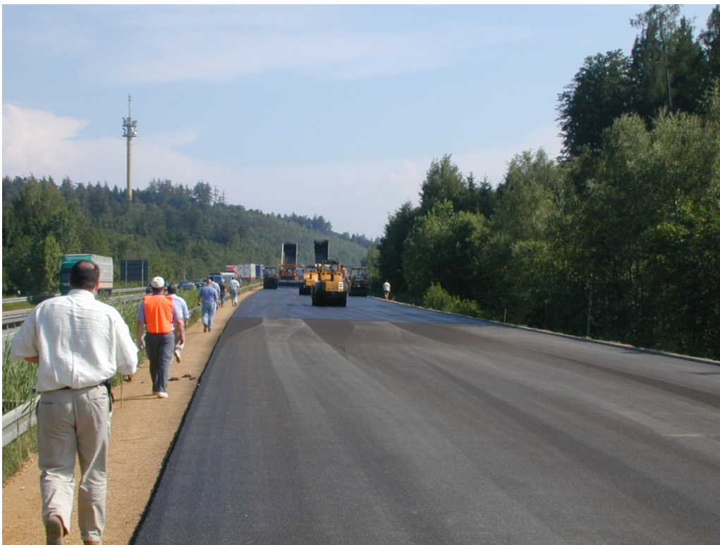
Figure 12. Gritted (Foreground) and Non-Gritted SMA Surface
