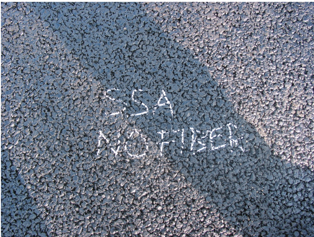
Figure 5. Typical Surface Texture, No Fibers
