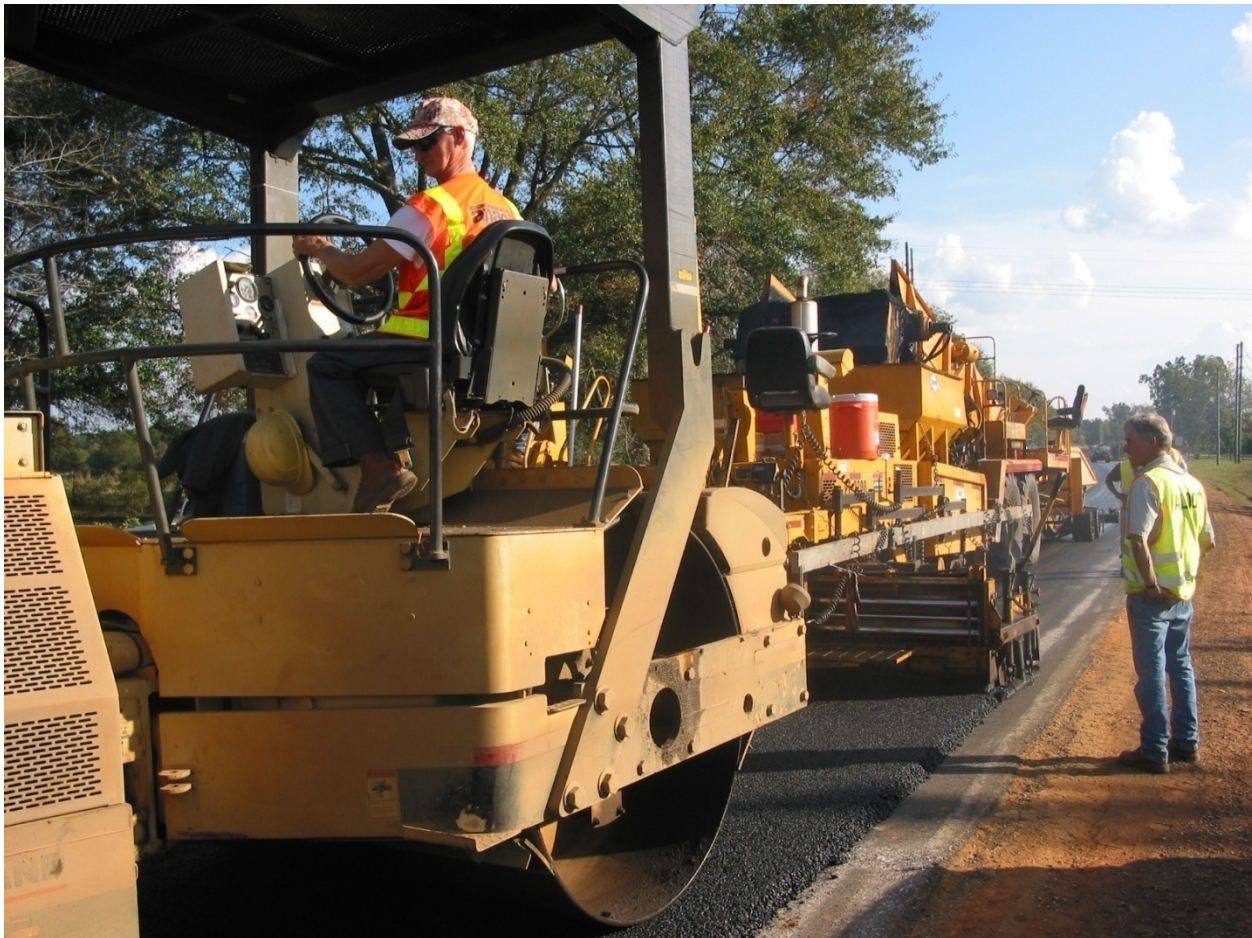
Figure 3. Paving Train with Breakdown Roller Close to Paver Screed
