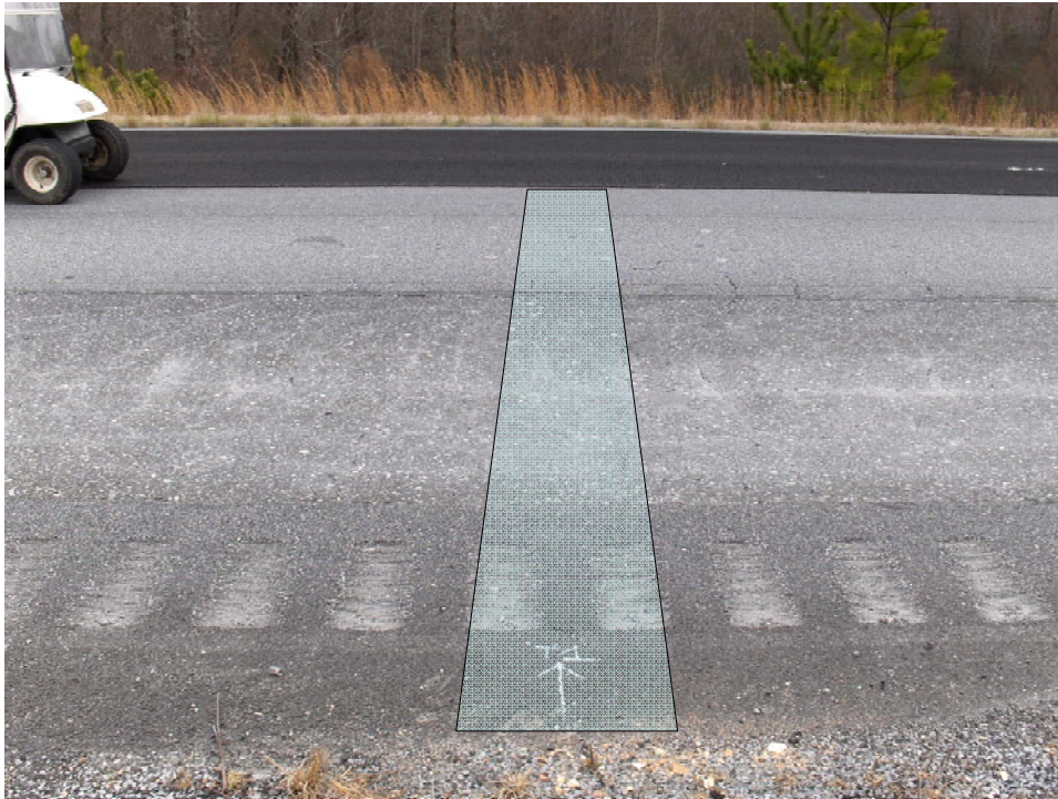
Figure 3.1 Location of Trench 1.
