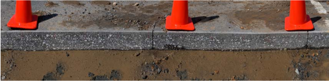
Figure 3.11 Trench 3 West Face.
