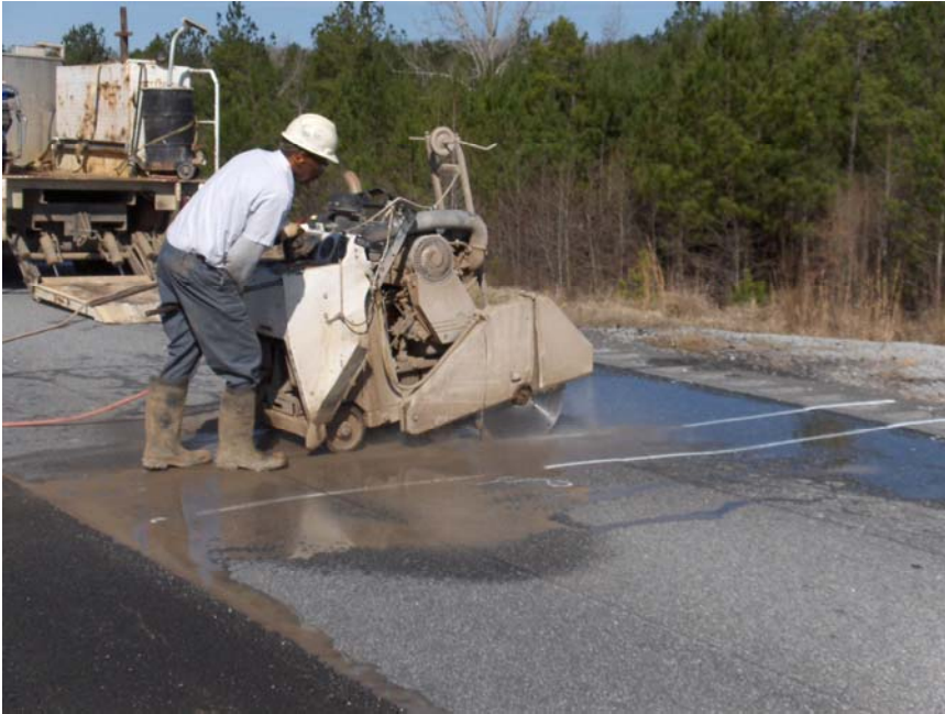
Figure 3.5 Cutting Trench 1.
