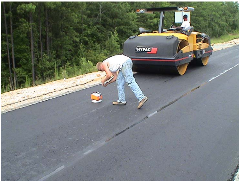
Figure 2.17 Steel-Wheel Compaction and Density Check.
