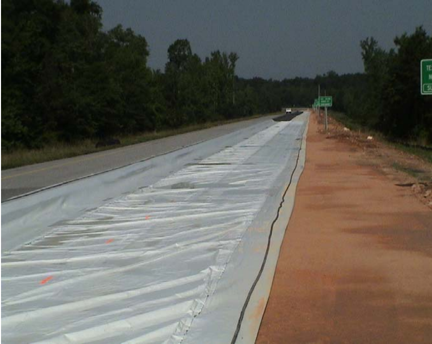
Figure 2.4 Tarp Covering Fill Material.
