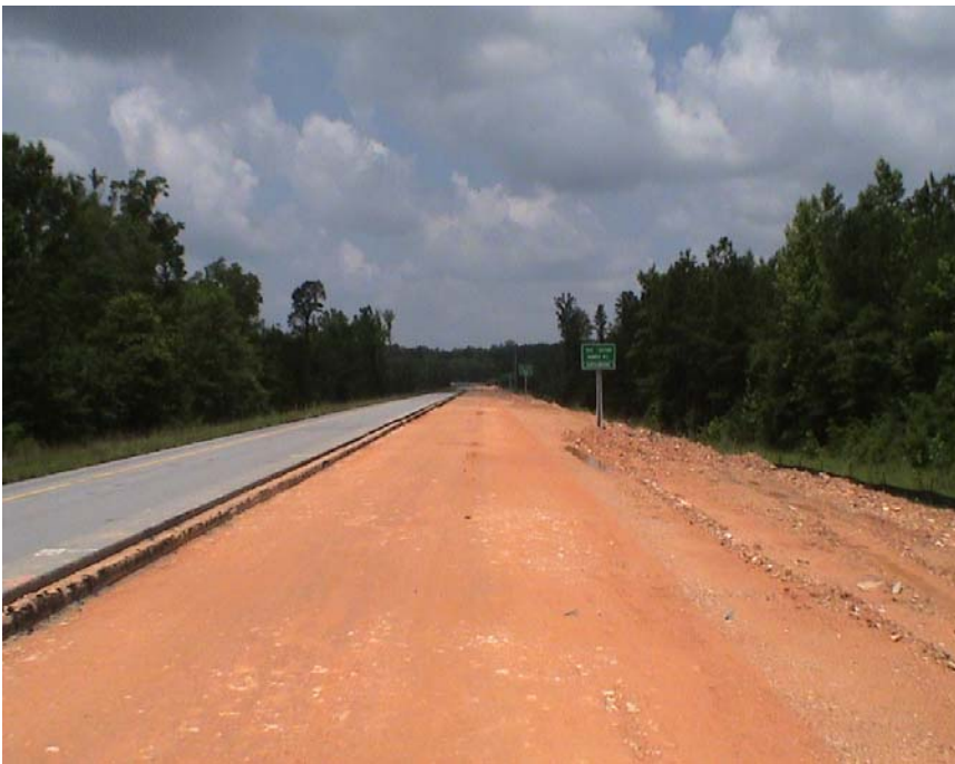
Figure 2.5 Completed Fill Layer.
