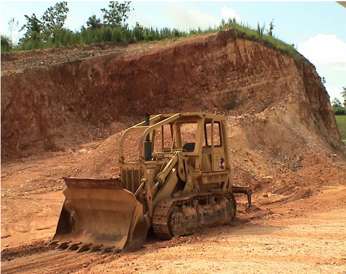
Figure 2.2 Excavation of Fill Material.
