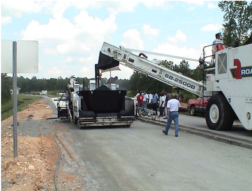
Figure 2.16 Use of Material Transfer Vehicle During Paving.
