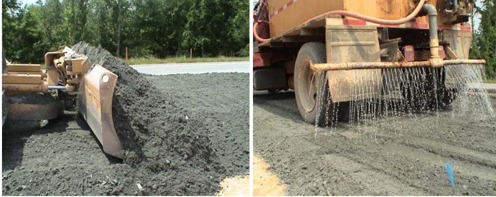
Figure 2.8 Granular Base Under Construction.
