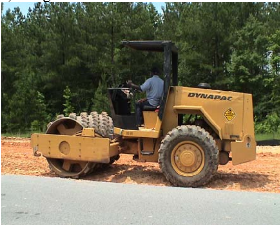
b) Rolling Compaction
