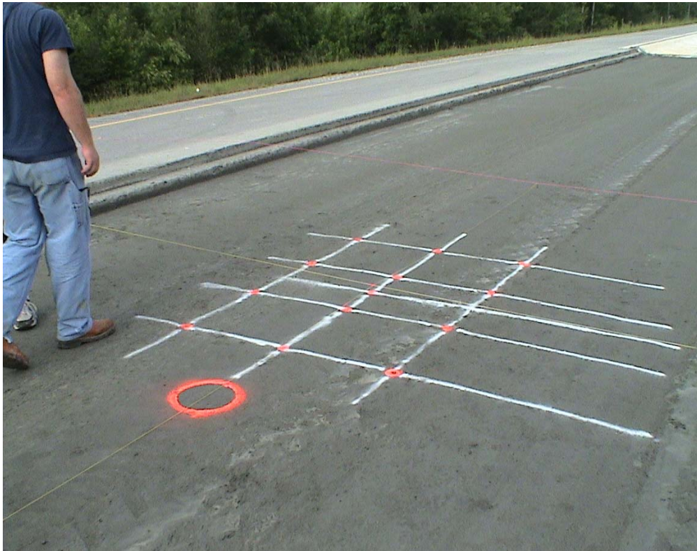
Figure 2.9 Granular Base Ready for Paving.
