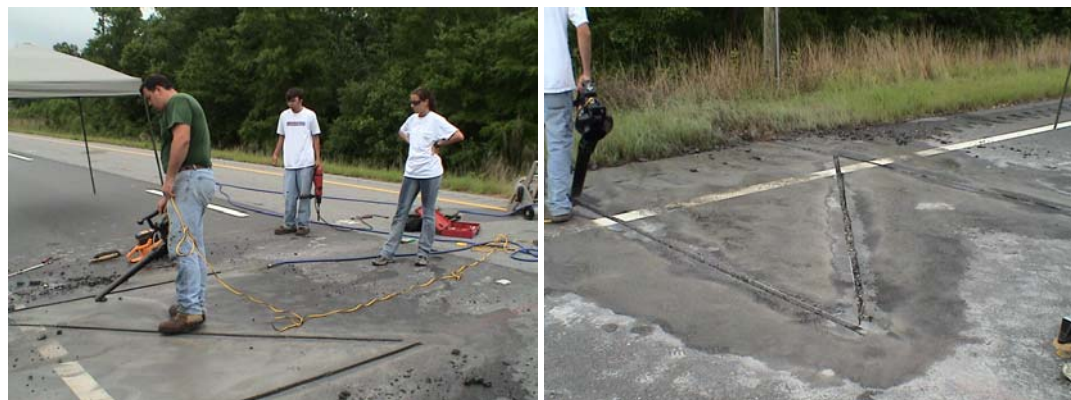
Figure 12. Cleaning Sensor Slots.
