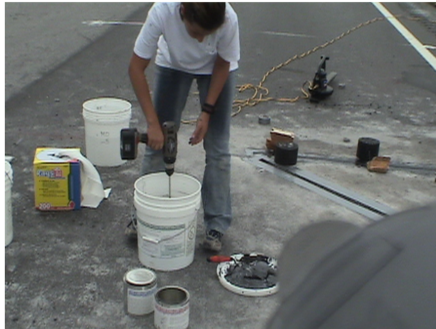
a) Mixing Epoxy
