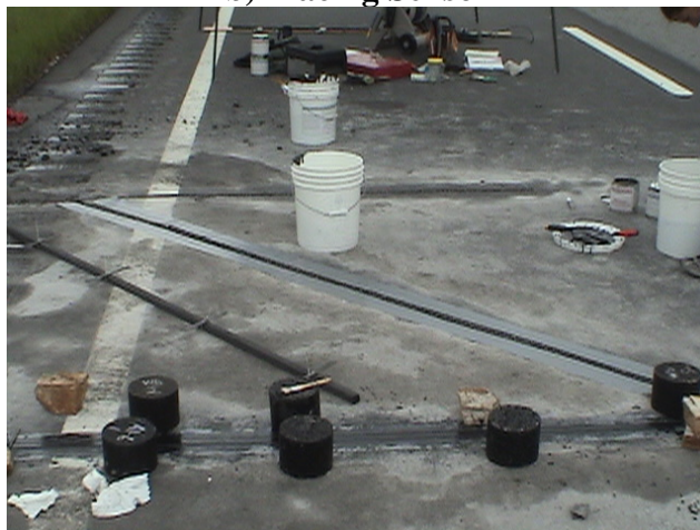
c) Sensor In-place, Waiting for Cure Time
