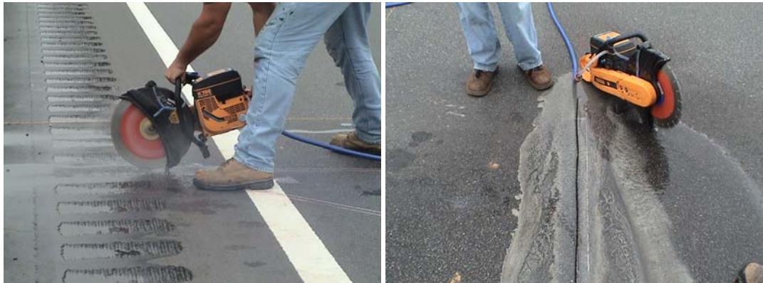
Figure 10. Cutting Sensor Slots.
