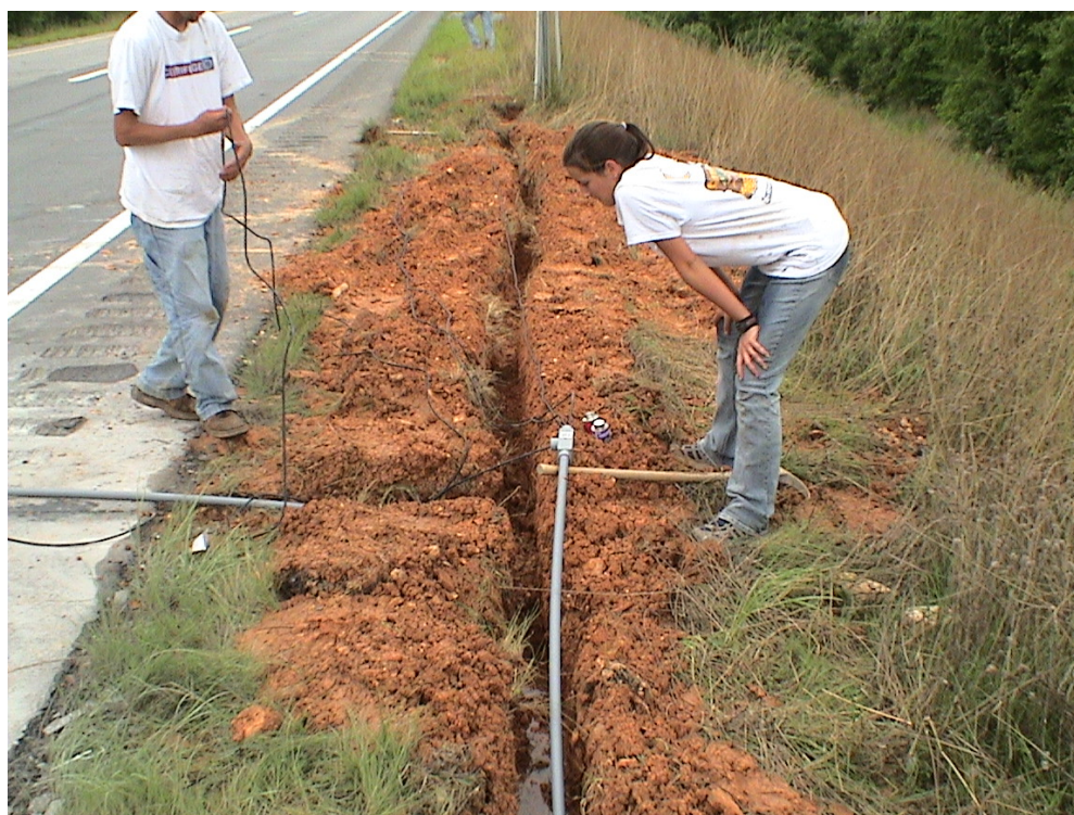
Figure 16. Burying Cable From Sensors to Data Acquisition Box.
