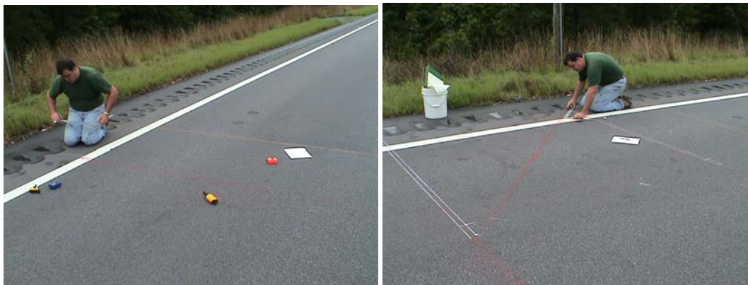
Figure 9. Laying Out Sensor Locations.
