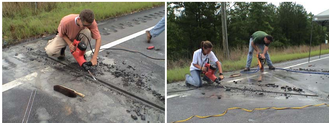
Figure 11. Chipping Out the Sensor Slots.
