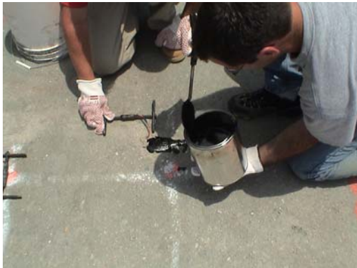
a) Placing Sand/Asphalt Mix
