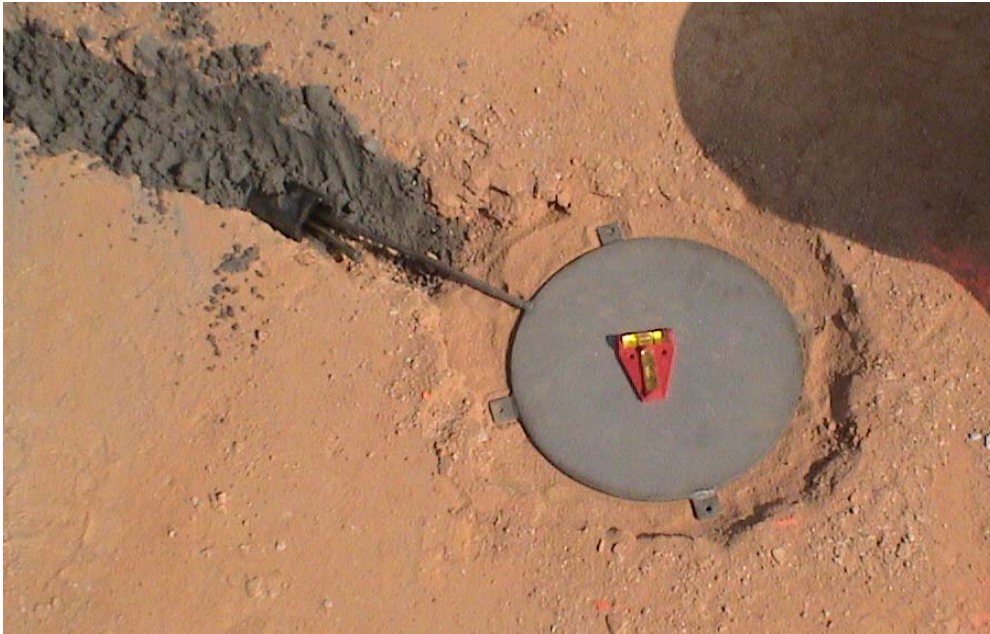
Figure 4.4 Leveling Subgrade Earth Pressure Cell.
