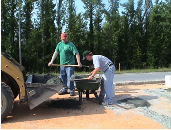
a) Sieving Granular Base for Cover
