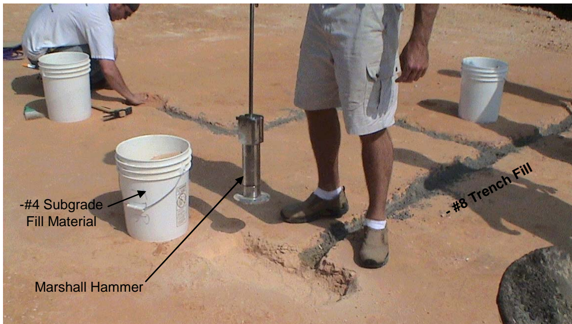
Figure 4.2. Compacting TDR Cavity and Backfilled Cable Trenches.
