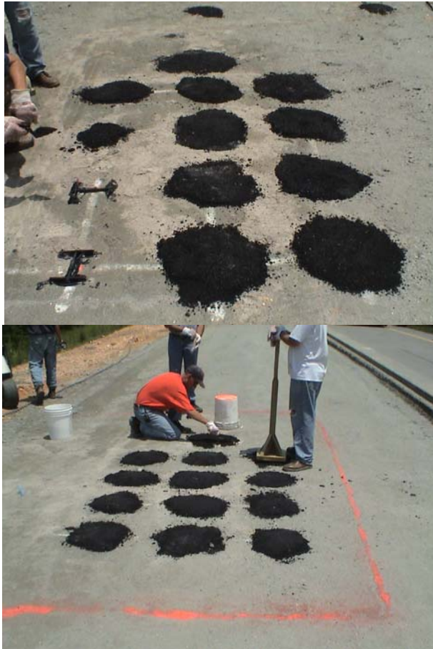
Figure 4.17 Placing Cover Material on ASGs.
