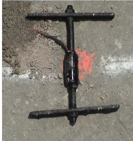
Figure 4.13 ASG with Cable Tie Missing from Axial Bar.
