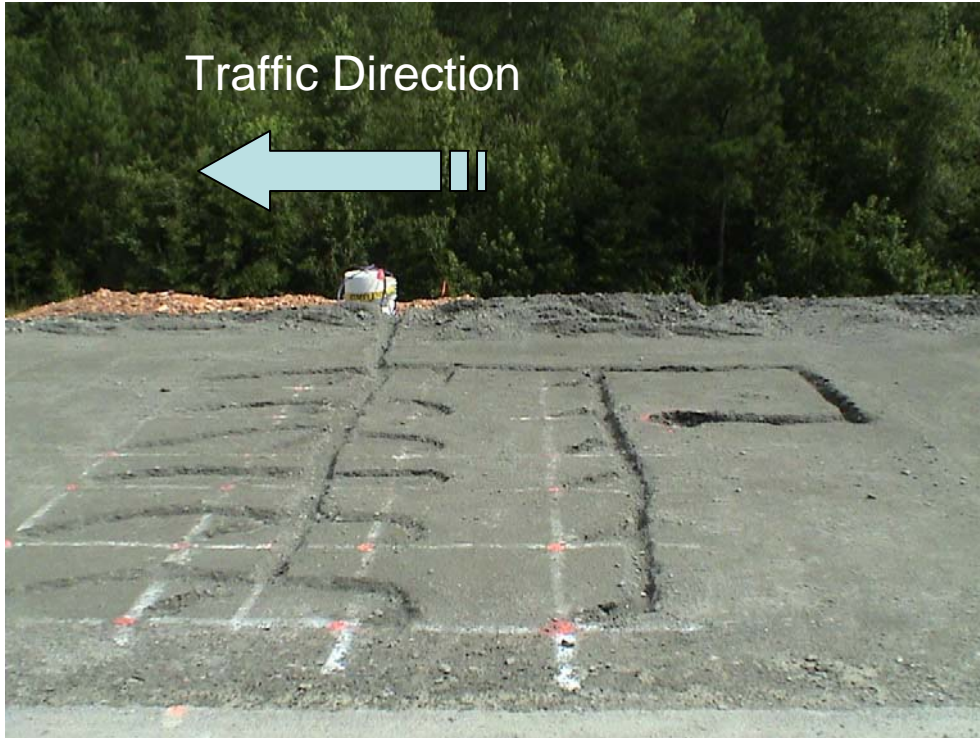
Figure 4.10 Cell N8 Excavation for ASG's and Earth Pressure Cells.
