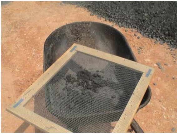
b) #4 Screen to Sieve Cover Material
