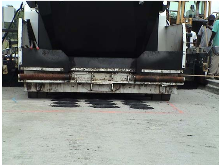
Figure 4.18 Paver Straddling Gauge Array.
