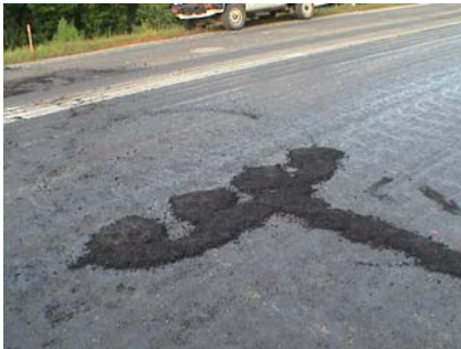
Figure 4.20 Installation of ASG's on Top of First Hot Mix Lift (Section N7).
