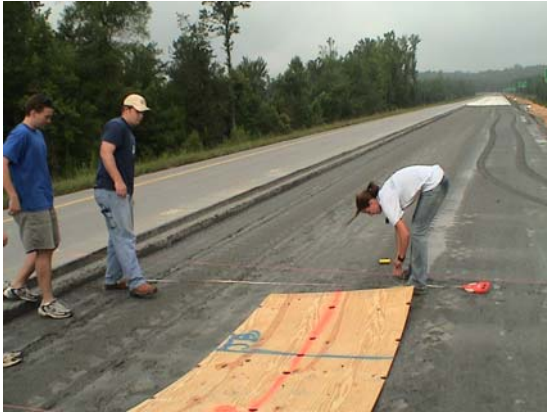
a) Setting String Lines
