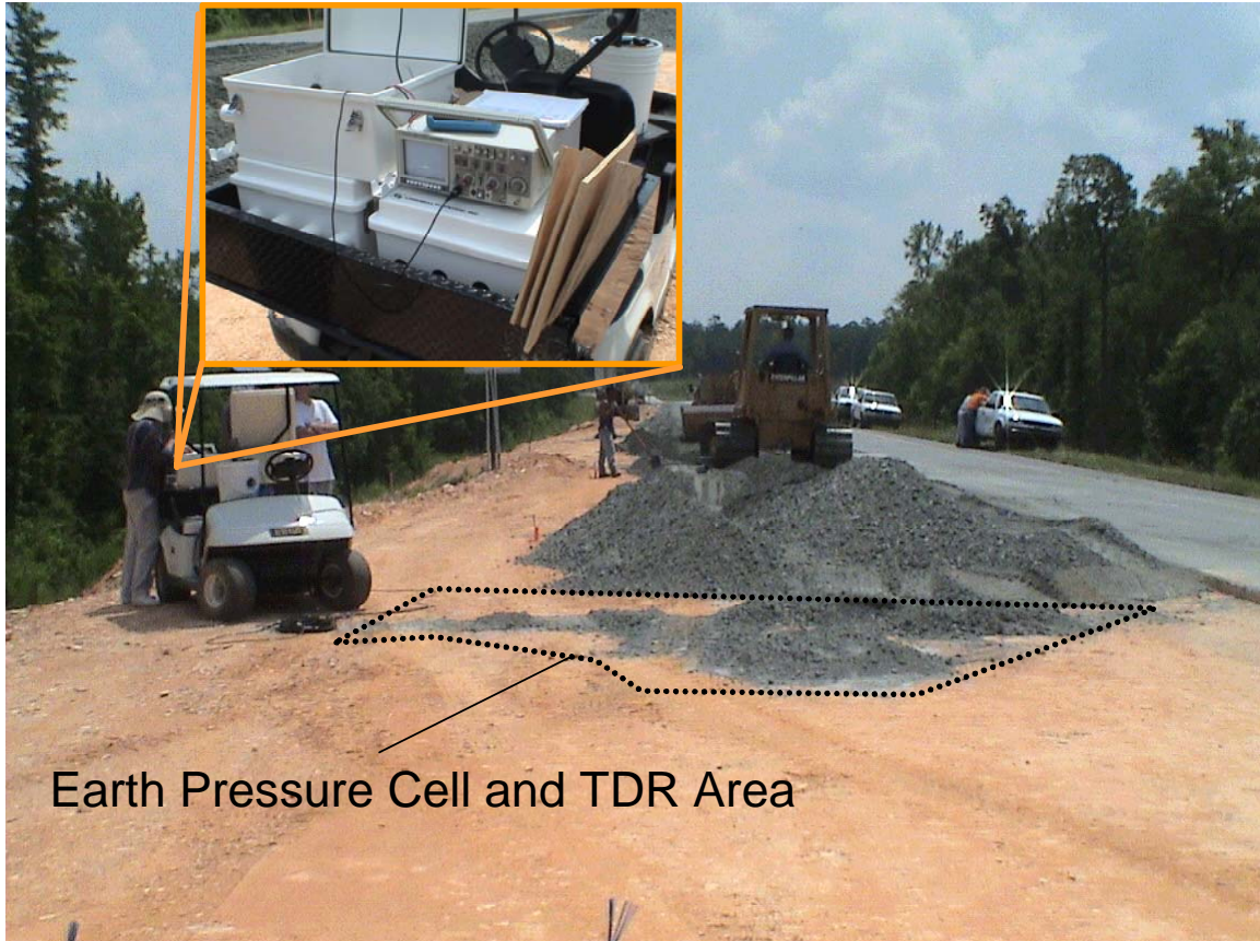
Figure 4.7 Base Construction and Gauge Monitoring.
