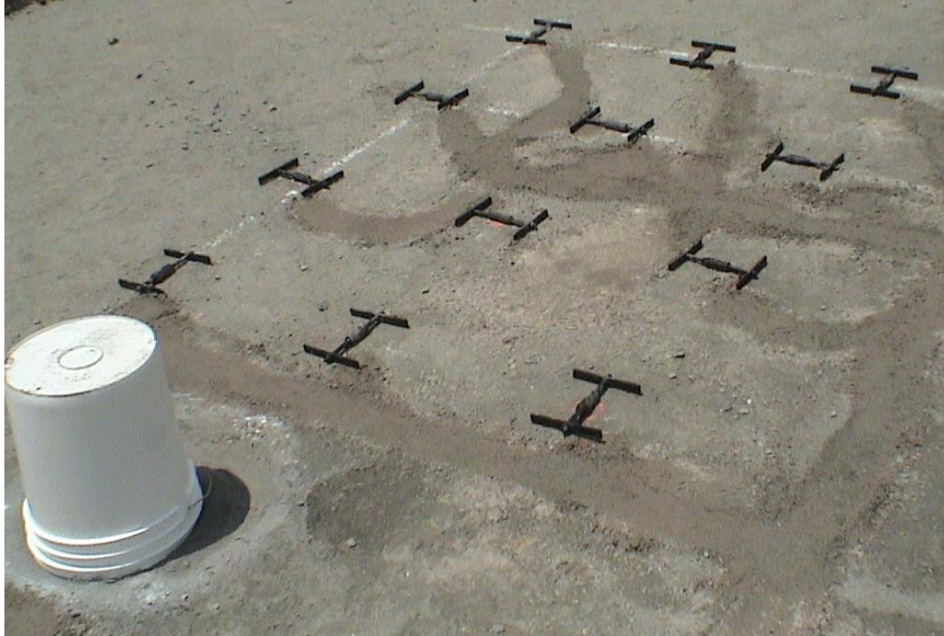
Figure 4.15 Gauge Layout Prior to Paving.
