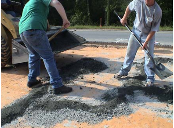
Figure 4.6 Hand Placement of Granular Base Material.
