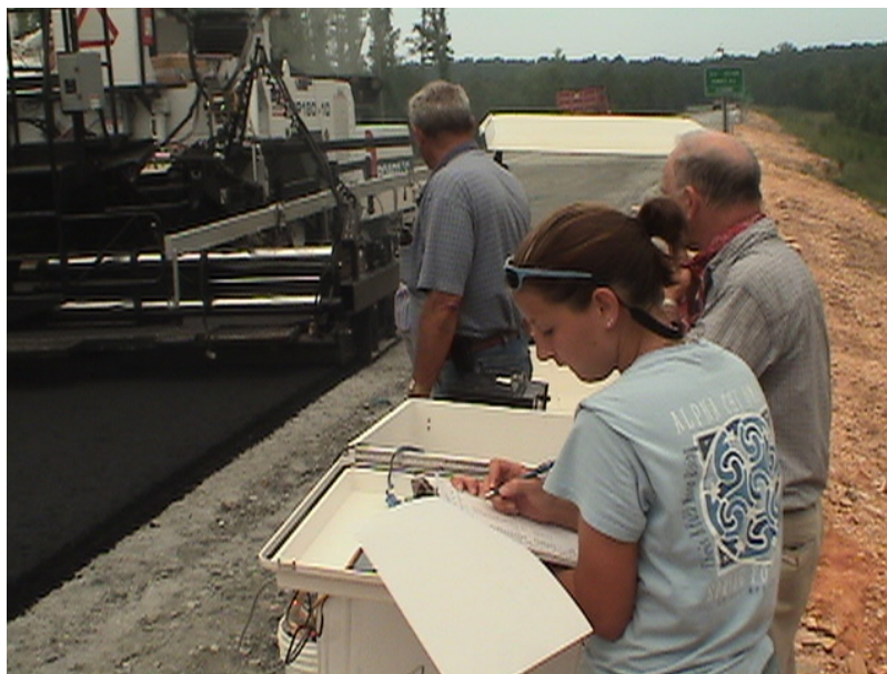
Figure 4.19 Monitoring Gauges During Construction.
