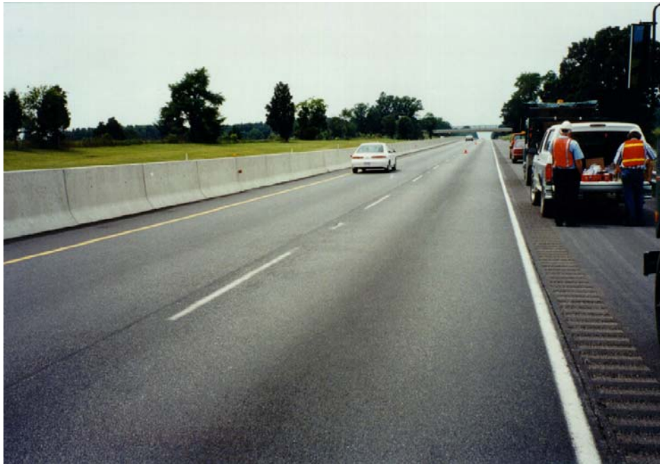
Figure 10. General View of the Relatively Good Area of the westbound Lanes Near MP 212.9
