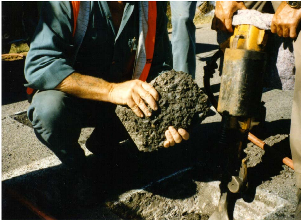
Figure 27. Excavation of Each Asphalt Layer With a Jack Hammer
