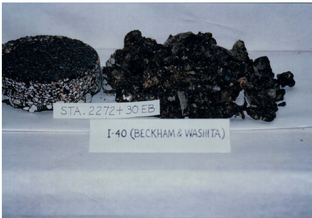
Figure 15. Stripped F Binder Mix (Right) Which Crumbled on Coring With an Intact OGFC Layer (I-40)
