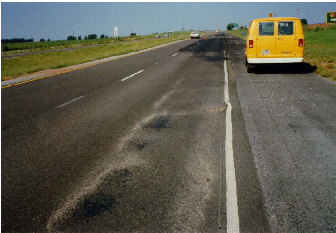
Figure 11. Development of Potholes Primarily in the Outside Wheel Track of I-40 in Oklahoma
