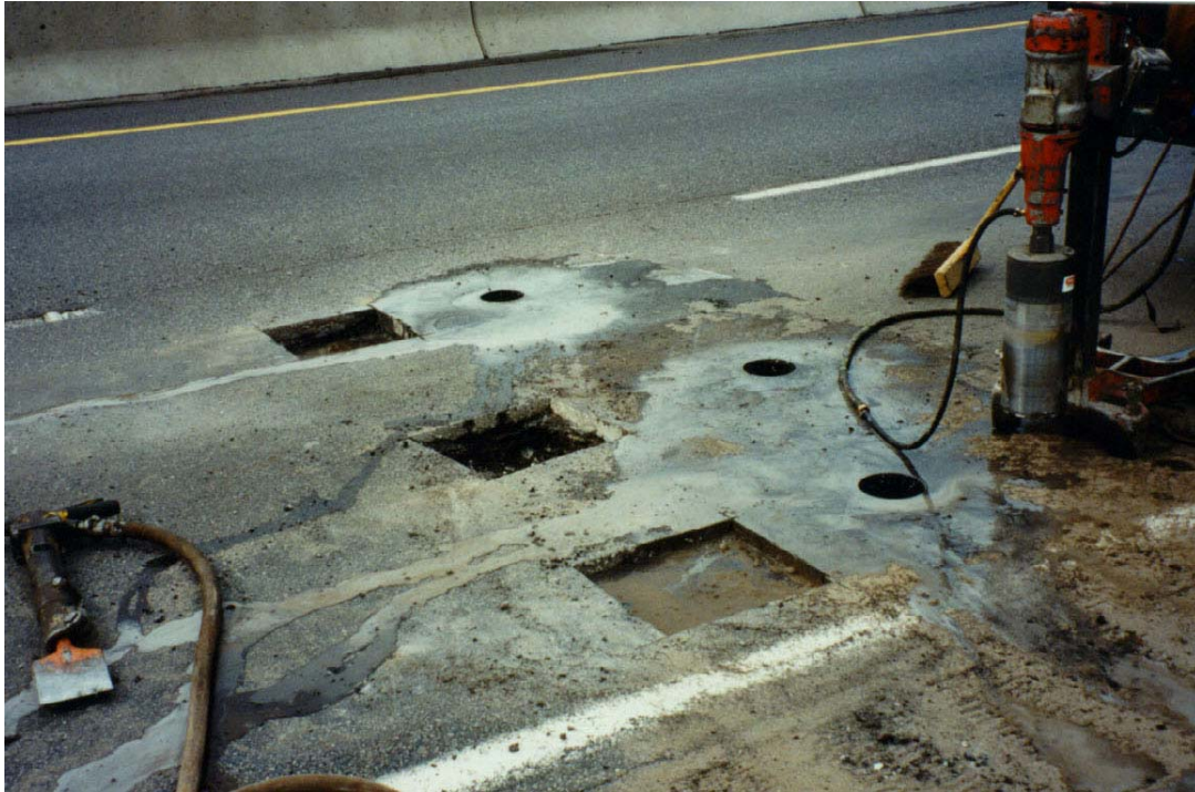
Figure 8. Cores Taken Adjacent to Square Holes at MP 217.65
