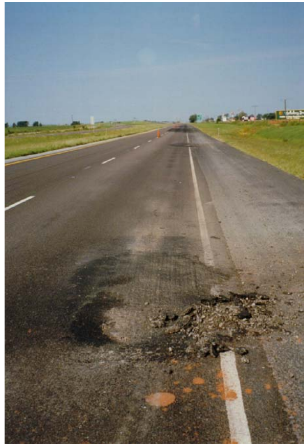
Figure 12. Potholing on I-40, Oklahoma
