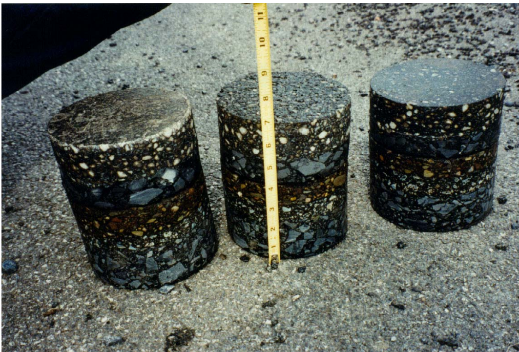
Figure 9. Cores Taken at MP 217.65 (From Left to Right): Inside Wheel Track, Between the Wheel Tracks, and Outside Wheel Track
