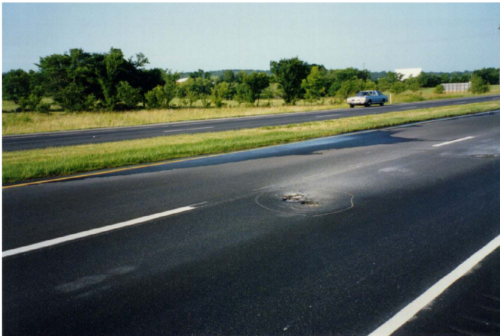
Figure 19. Water From the Raised Grassy Median
