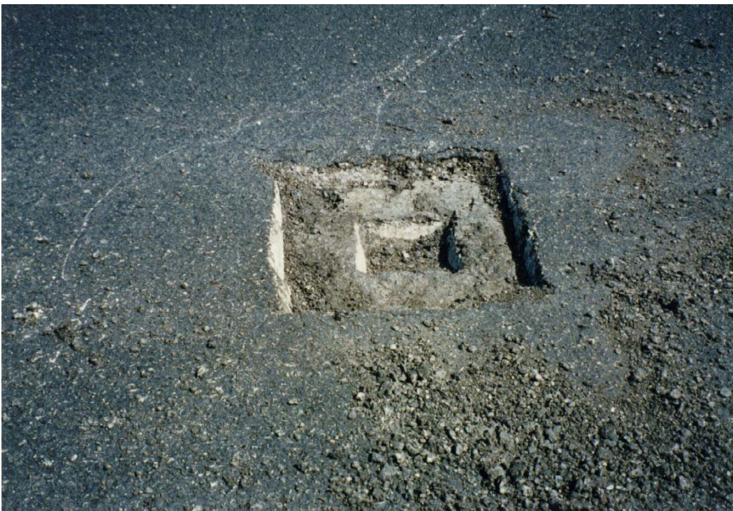
Figure 21. E Mix and B Mix Layers Removed by Jack Hammer
