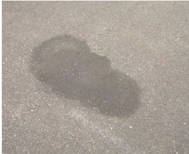
Figure 17. Oil Spillage
