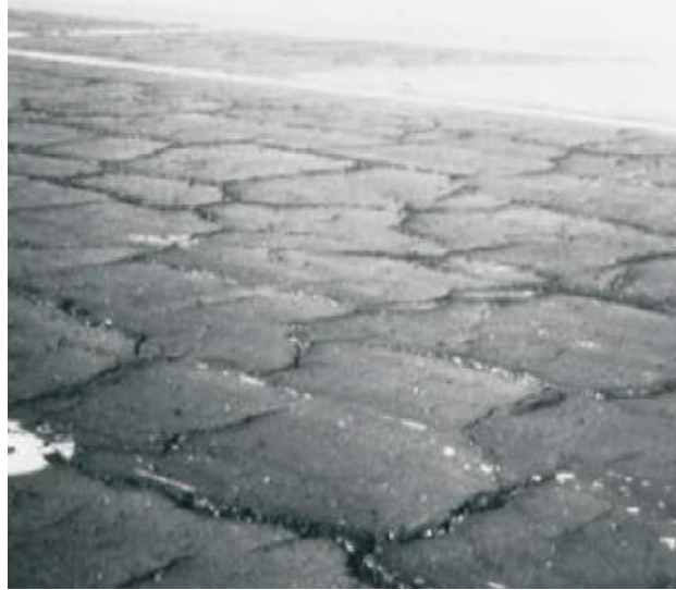
Figure 11. Block Cracking
