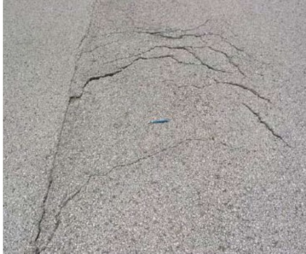
Figure 23. Slippage Cracking
