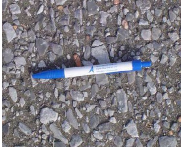
Figure 19. Polished Aggregate
