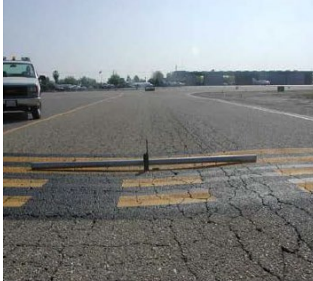
Figure 21. Rutting
