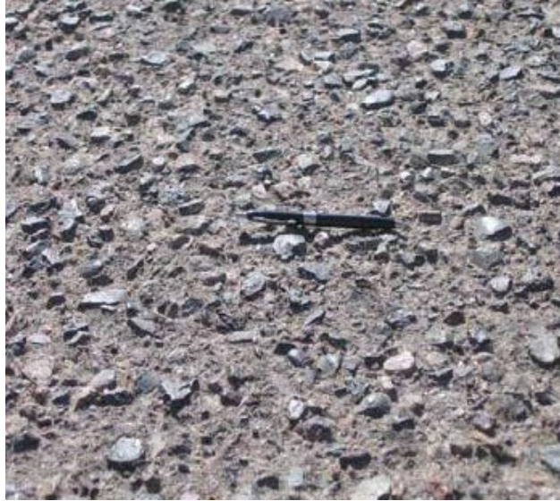
Figure 25. Weathering (Surface Wear)
