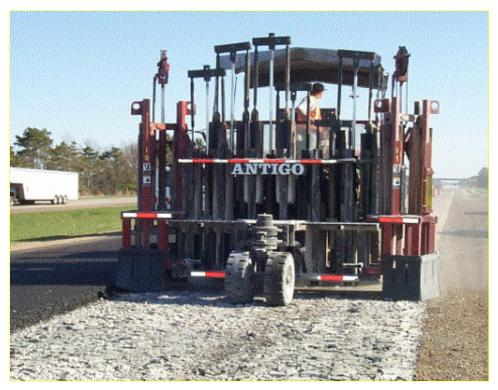
Figure 9. Multiple-Drop Hammer for Rubblizing PCC Slabs
