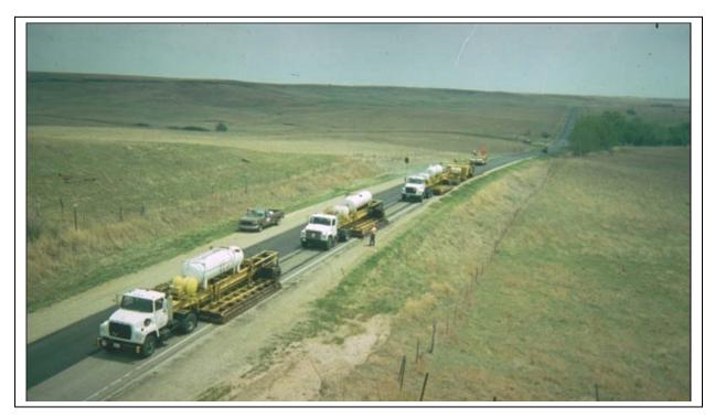
Figure 11. Heater Scarification of HMA Surfaced Pavements
