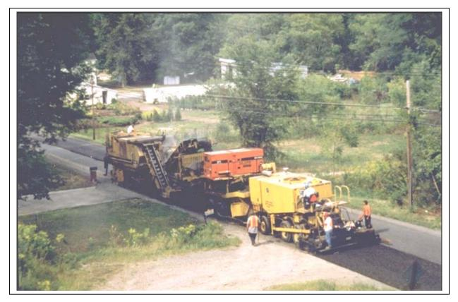
Figure 12. Cold In Placed Recycling Method of Flexible Pavements
