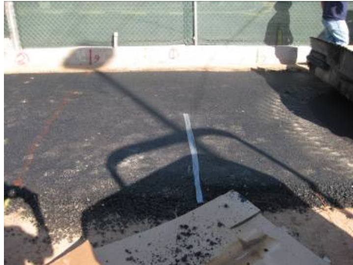
Figure C.7 – Installation of Thermocouple on Asphalt Base
