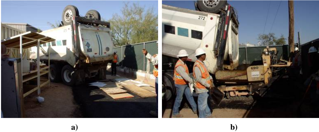
Figure C.8 – HMA Delivery to the Site
