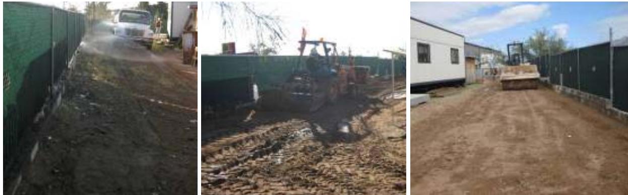
Figure C.4 – Preparation of Subgrade
