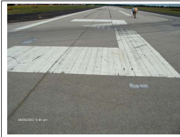
Rantoul Airport – Control Section
