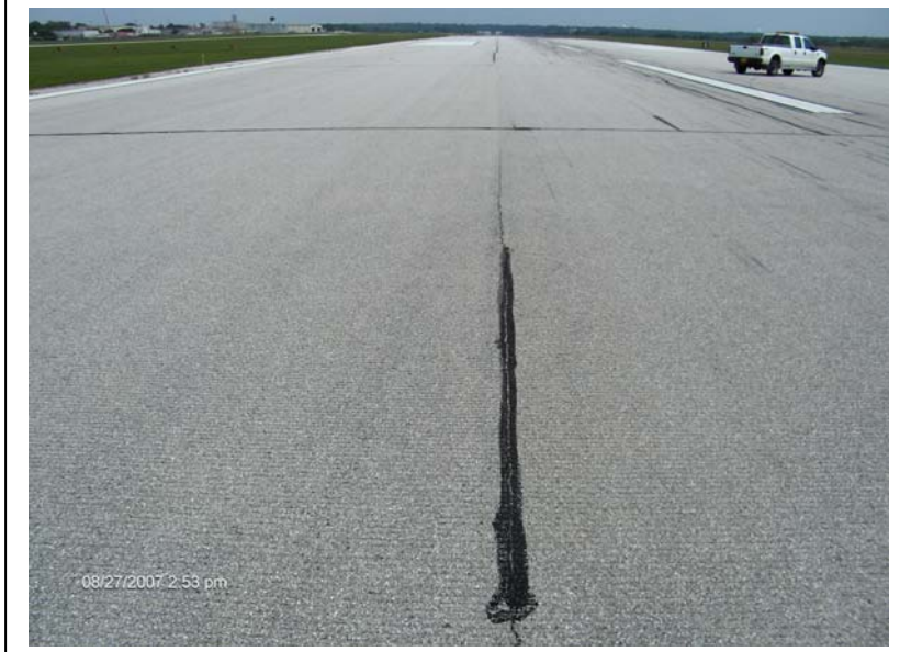
Purdue University Airport – Full-Depth Reclamation for Runway Rehabilitation.
