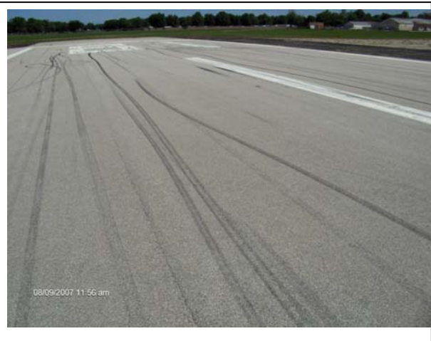
Rantoul Airport – Rubblized Section
