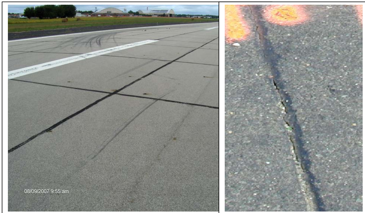
Figure 23 Saw and Seal Method for Crack Control
