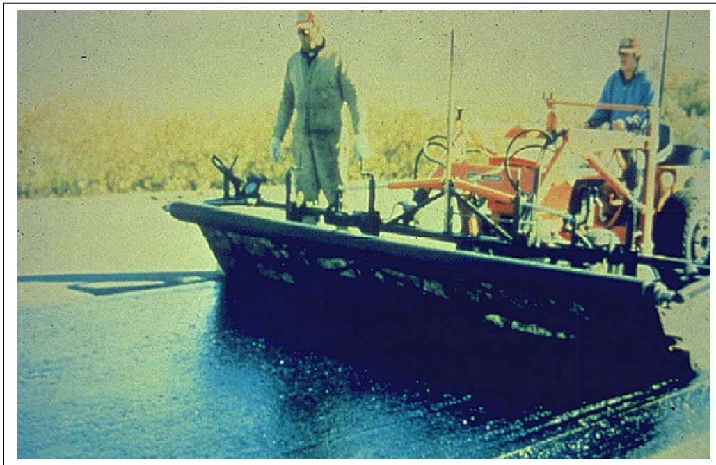
Figure 21 Geosynthetics Interlayer Used in a Stress/Strain Interlayer
