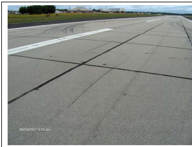
Rantoul Airport – Saw and Seal Section
