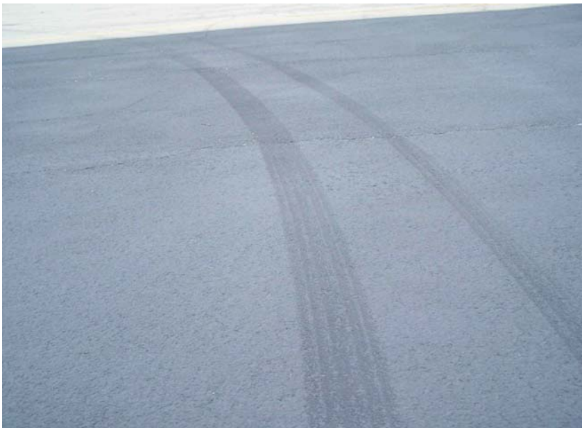
Figure 2-6 – Rubber Tire Tracks from USAF C-17 High Performance Turn.
