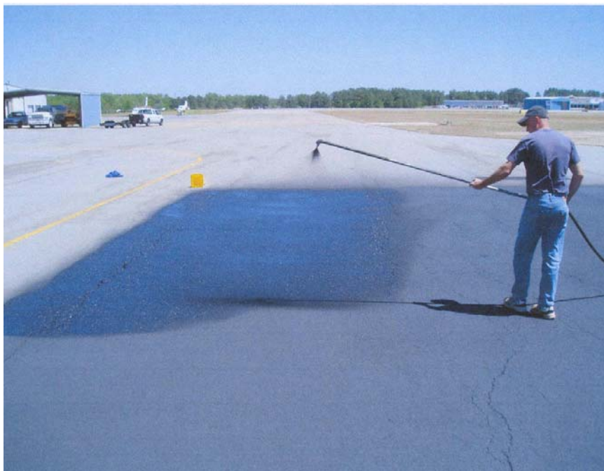
Figure 2-3 – CarbonPlex Application, Apron, Columbia Airport, SC, 2007.
