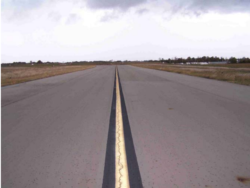
Figure 2-13 – E-Krete on East End of Main Taxiway, Tupelo Regional.
