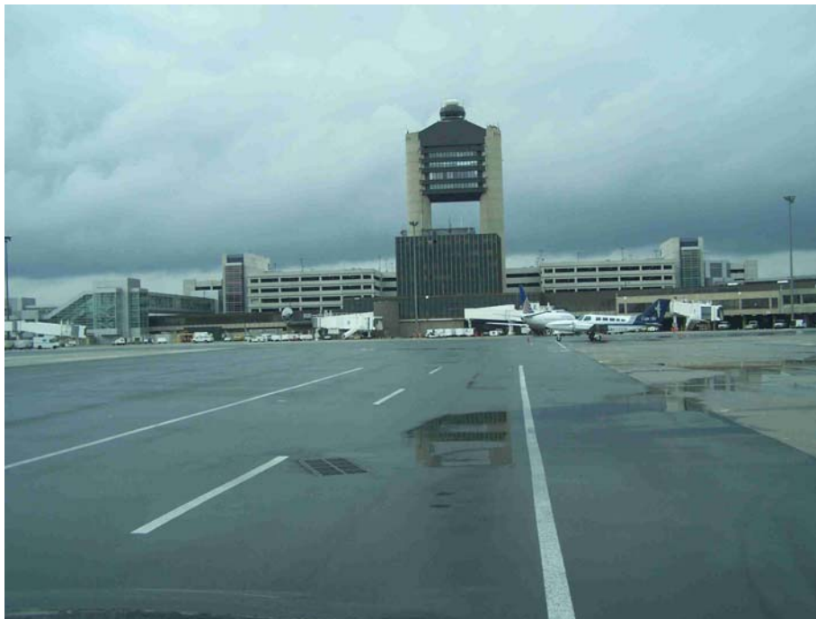
Figure 2-24 – View of Alley B-C Pavement, BLIAP, November 2006
