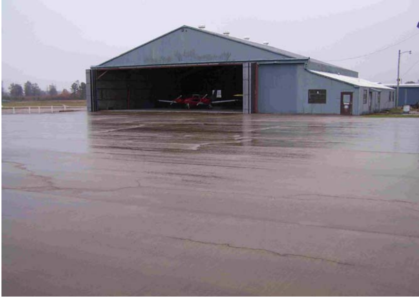
Figure 2-17 – Corinth-Alcorn County Airport, Apron and Hangar
