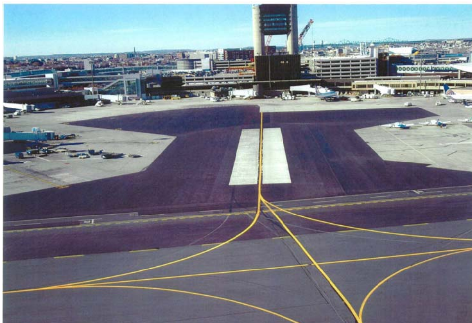
Figure 2-23 – Completed Alleyway B-C Project, Boston Logan IAP, November, 2006.
