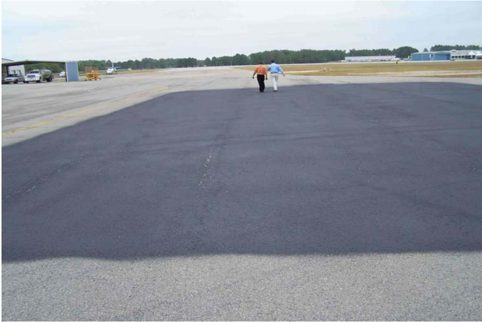
Figure 2-4 – CarbonPlex Sealer Demonstration Section, October 2007
