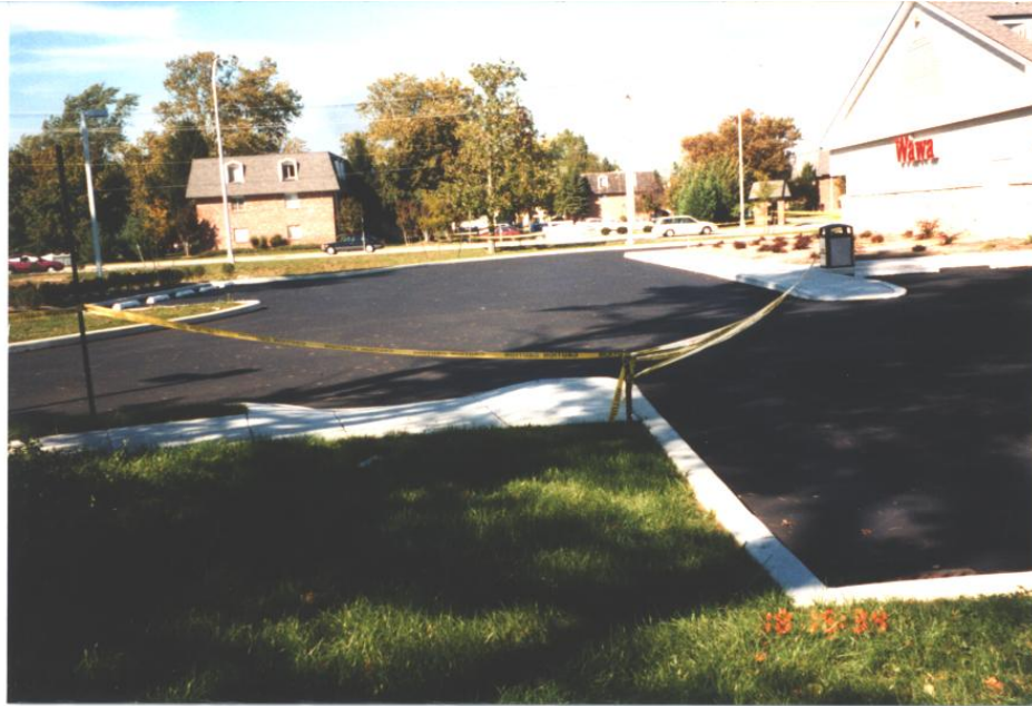
Figure 2-2 Typical Parking Lot Application, LAS-320 Sealer, New York
