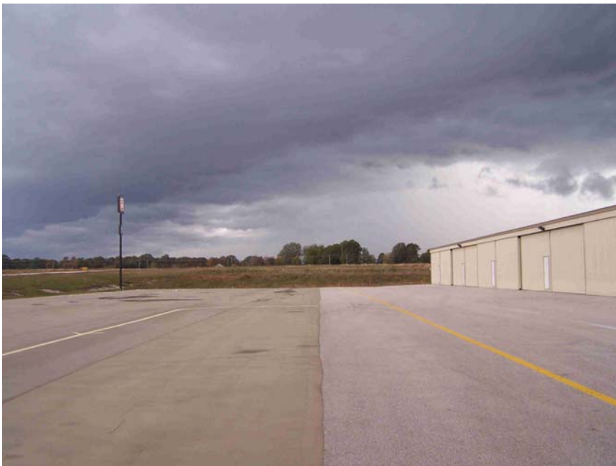
Figure 2-14 – E-Krete on General Aviation Storage and Refueling Area, Tupelo Regional
