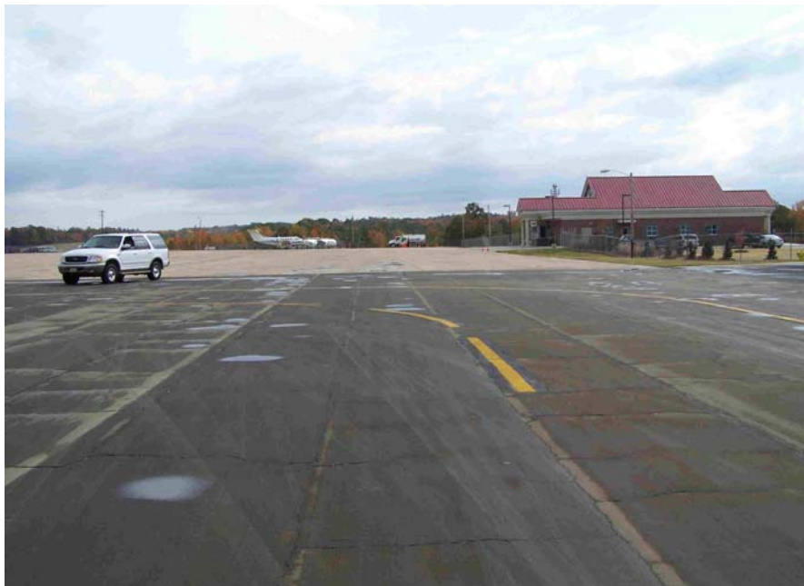
Figure 2-9 – University Oxford GA Apron, Westward Look.
