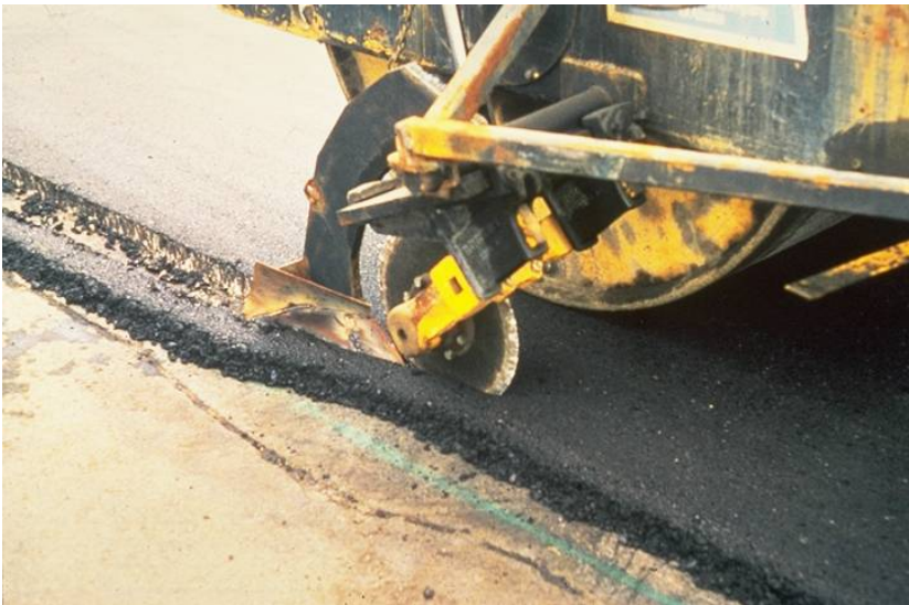
Figure 15.6 – Cutting back free edge prior to placing adjacent lane
