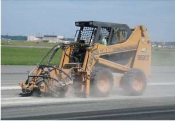
Figure 17.8 – Grinder attached to a skid steer loader (photo credit: D. Spiedel)
