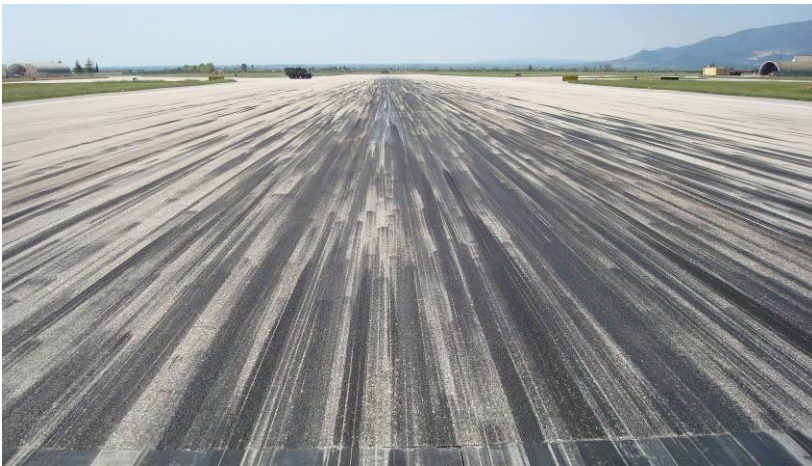
Figure 11.5 – Rubber buildup on runway end
