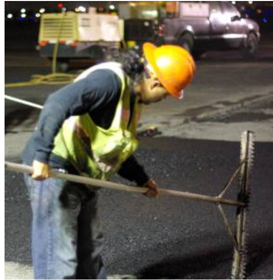
Figure 12.4 – Lute with a smooth edge (left side) and a rake edge (right side)
