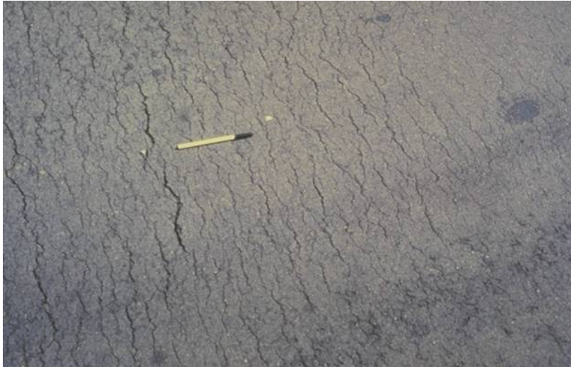
Figure 14.5 – Roller checking
