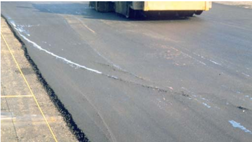
Figure 14.4 – Roller marks
