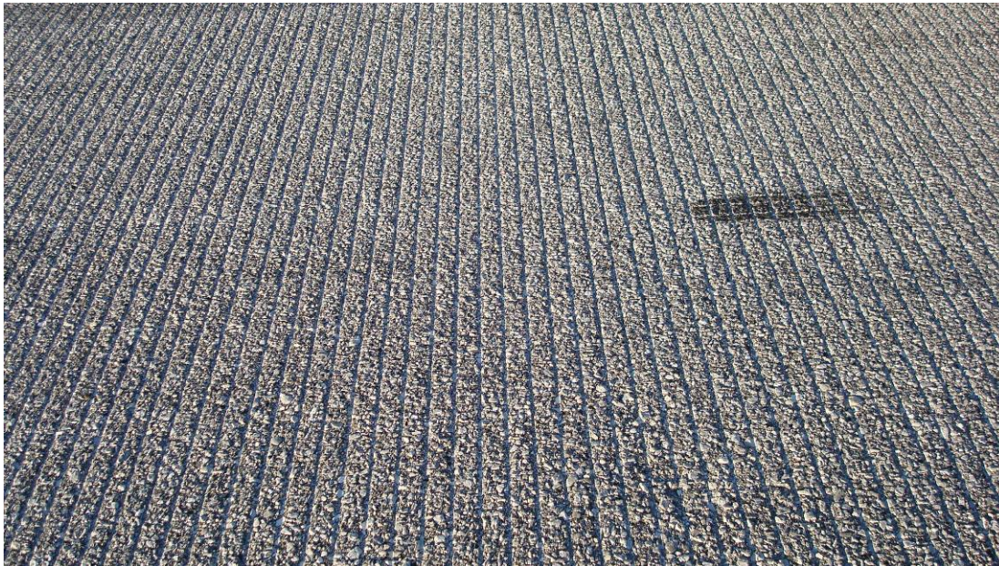
Figure 16.1 – Appearance of typical grooves after traffic
