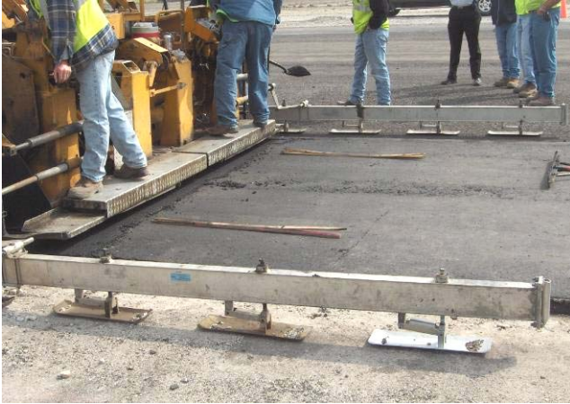
Figure 13.5 – Strips underneath paver to provide sufficient thickness for rolldown
