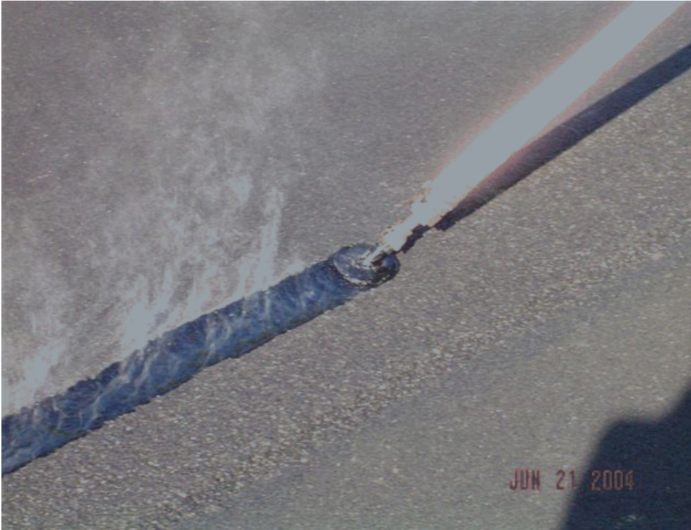
Figure 15.9 – Application of rubberized tack coat at notch
