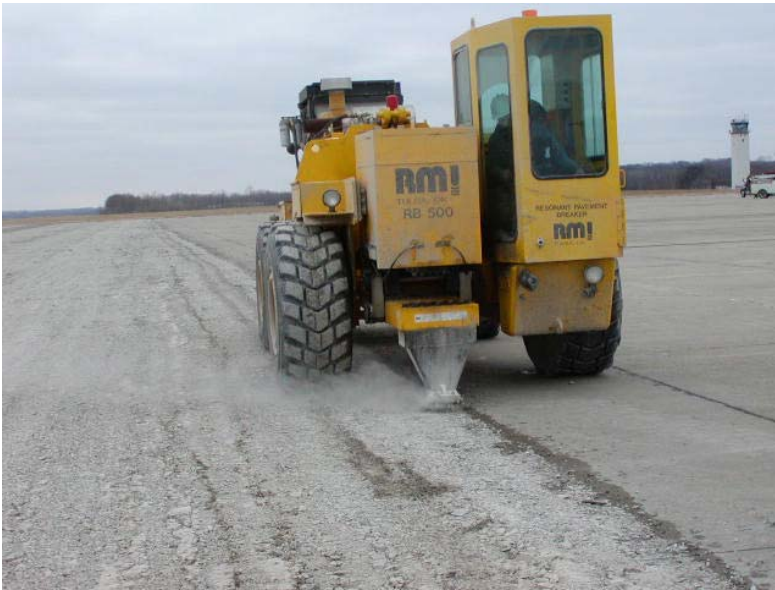
Figure 5.1 – Resonant pavement breaker (courtesy of Asphalt Institute)
