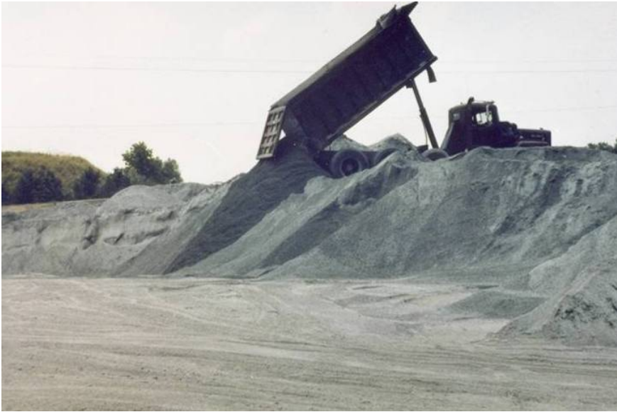
Figure 9.1 – Improper procedure for adding material to a stockpile
