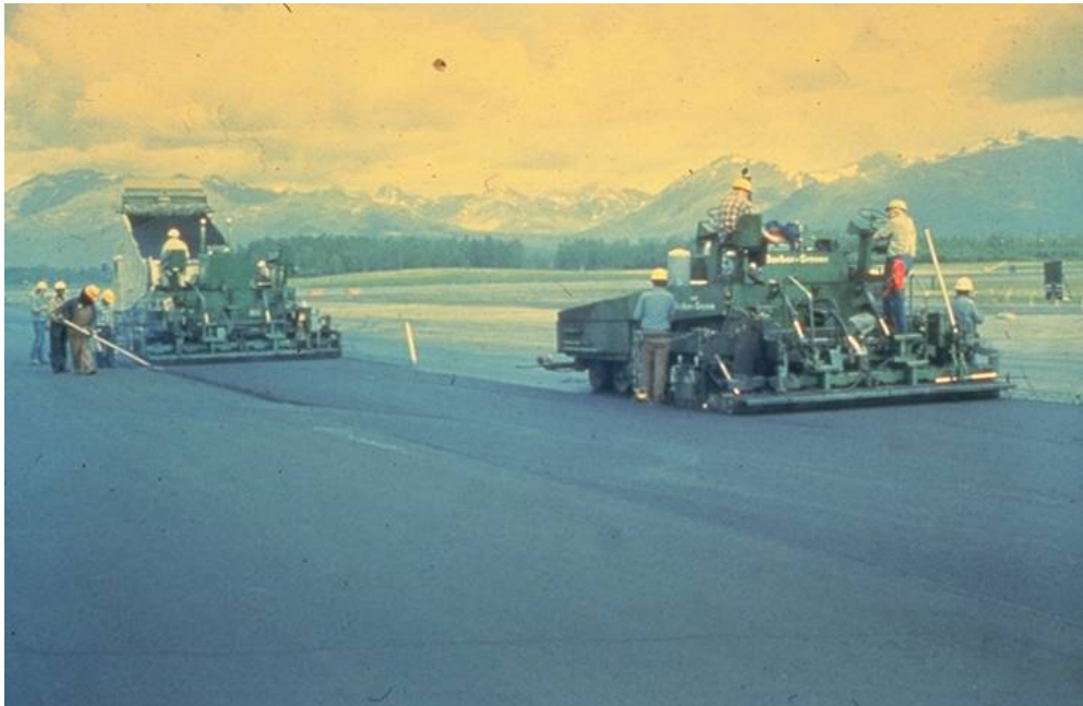
Figure 15.5 – Paving in echelon
