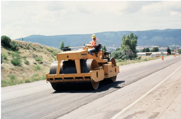
Figure 3.3 – Example of a static steel-wheel roller
