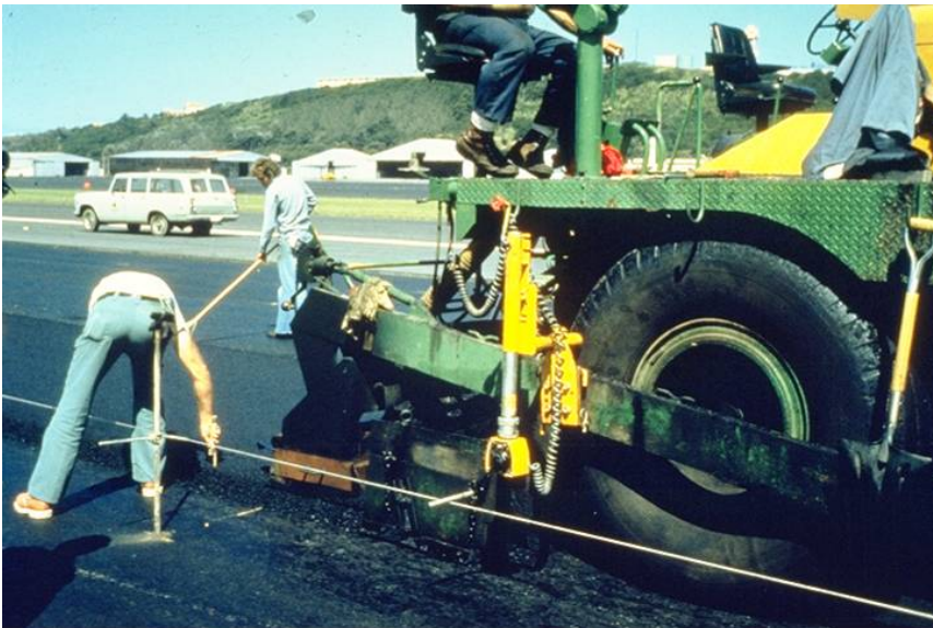
Figure 13.7 – Use of stringline to control grade
