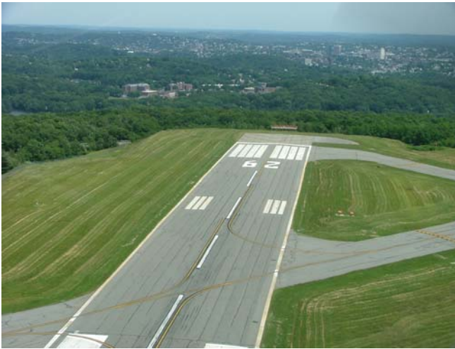
Figure 15.1 – Aerial view of runway with many longitudinal joints
