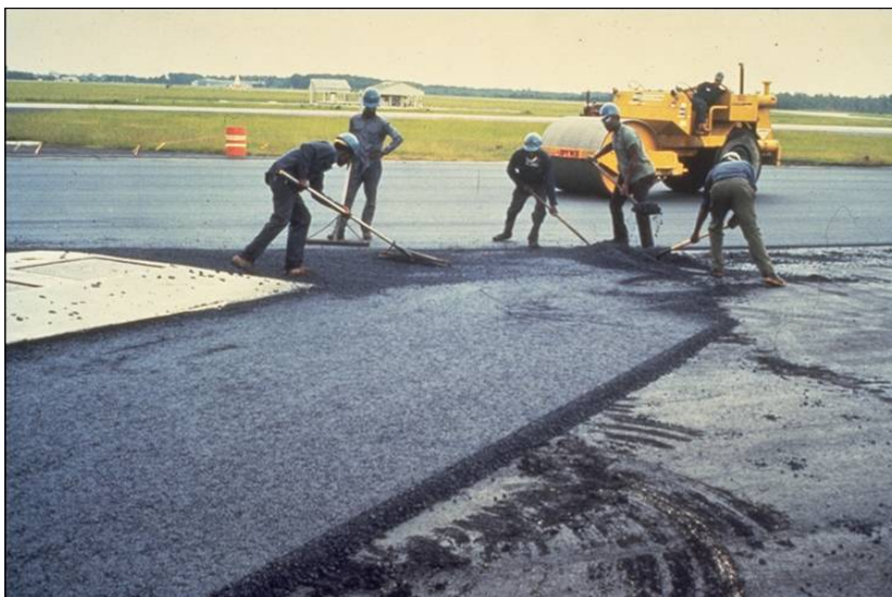
Figure 12.1 – Handwork around concrete structure
