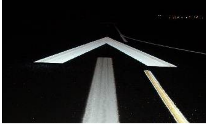
Figure 17.5 – Type III glass beads in the arrowhead with a higher index of reflection (1.9) provide better visibility than Type I glass beads in the tail with a lower index of reflection (1.5) (photo credit: D. Spiedel)
