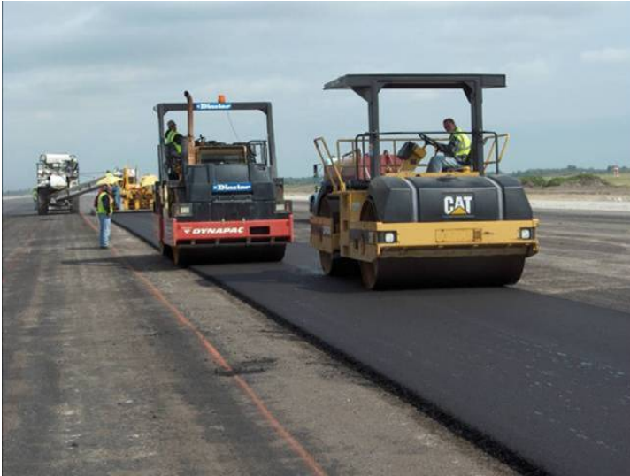
Figure 15.4 – Paving a straight line
