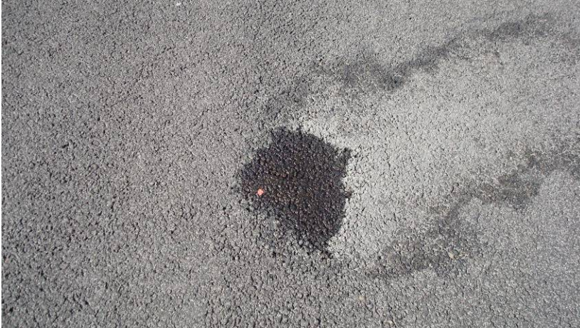
Figure 20.8 – Water from vapor pressure seeping up through pavement surface
