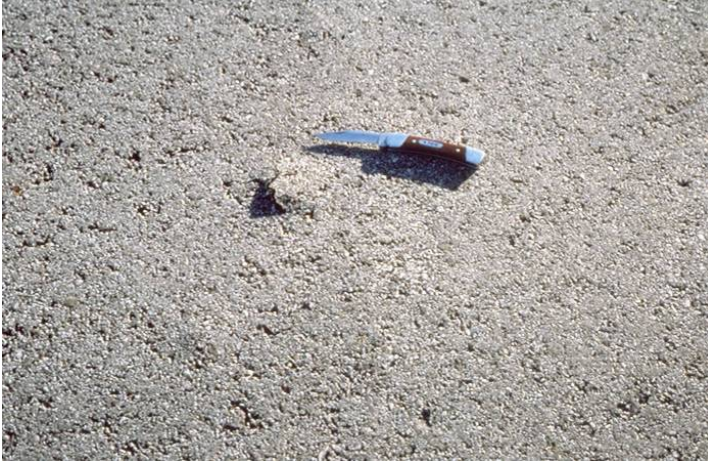
Figure 20.11 – Potential popout due to clayball
