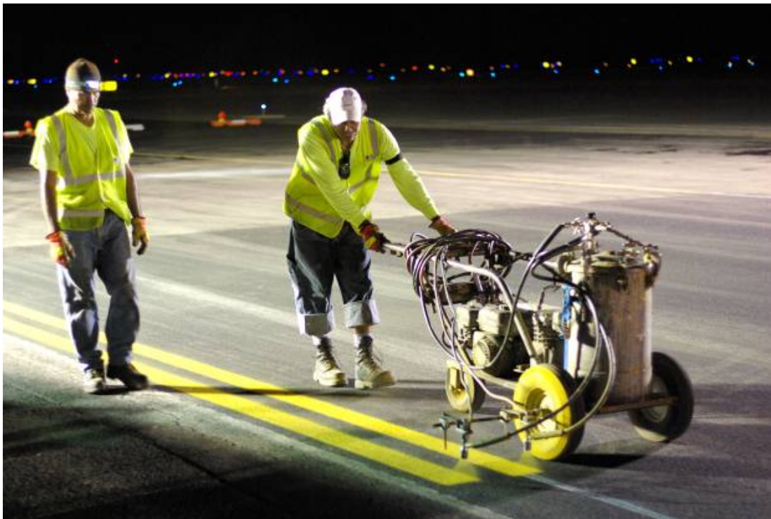
Figure 17.3 – Hand-operated sprayer for temporary markings
