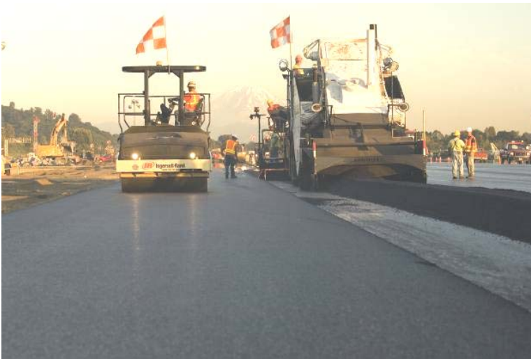
Figure 13.3 – Placement of HMA using windrowing process
