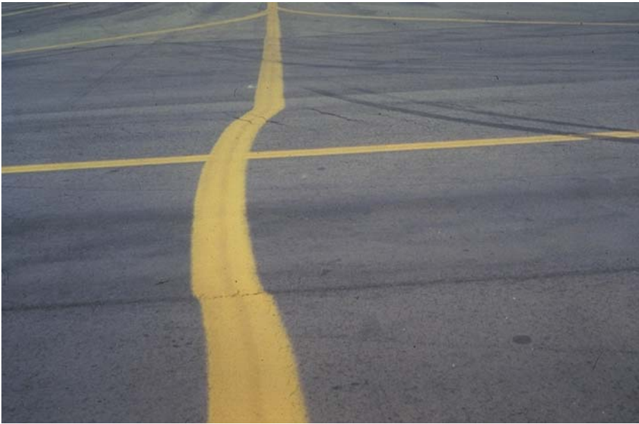
Figure 20.4 – Slippage of HMA surface showing distorted line
