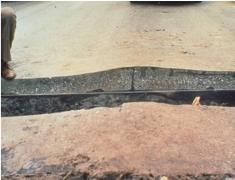
Figure 20.1 – Trench cut across a rutted pavement
