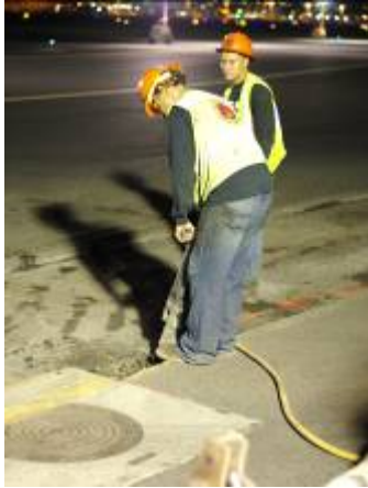
Figure 12.8 – Jackhammering HMA around a manhole
