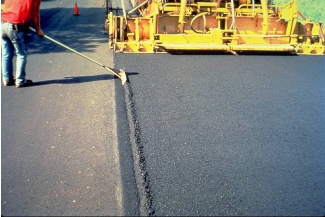
Figure 12.5 – Bumping the longitudinal joint
