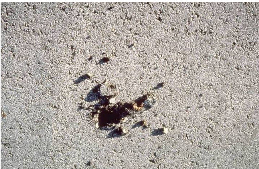
Figure 9.3 – Contamination with clayballs
