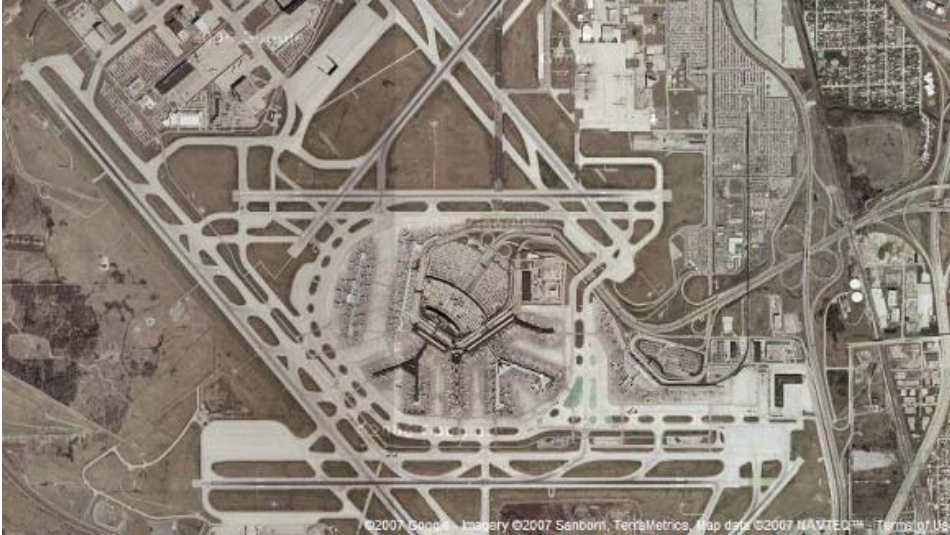
Figure 12.6 – Chicago’s O’Hare International Airport showing runways and taxiways and fillets at connection points (image from Google Maps, 2007)
