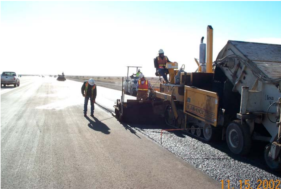
Figure 15.3 – Hot lane being placed next to adjacent cold lane
