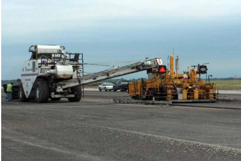
Figure 13.4 – Use of material transfer vehicle (MTV) in placing HMA
