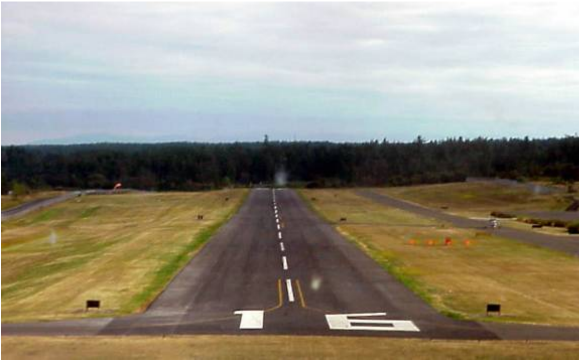
Figure 17.1 – New striping at the Port of Friday Harbor airport in WA
