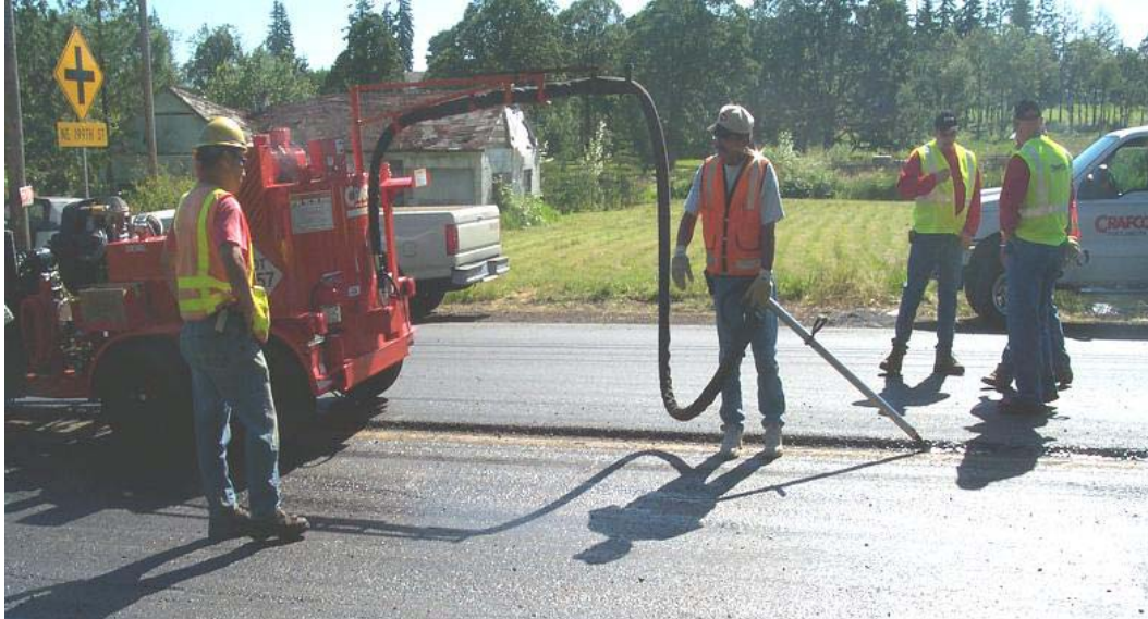
Figure 15. Application equipment for rubberized asphalt tack coat
