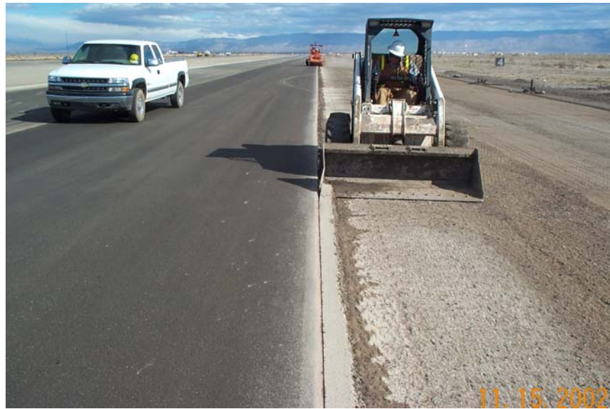
Figure 35. Removing approximately 200 mm of unconfined edge
