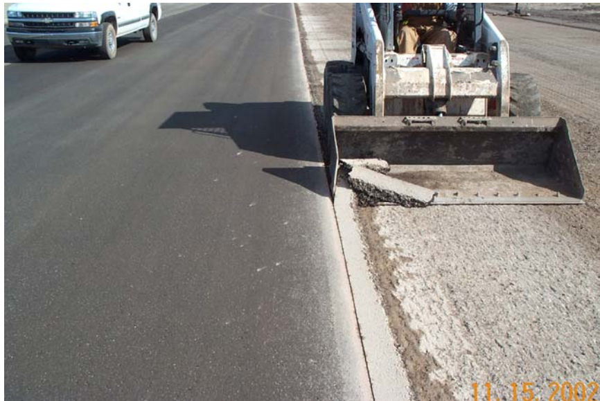
Figure 4. Removing cut edge
