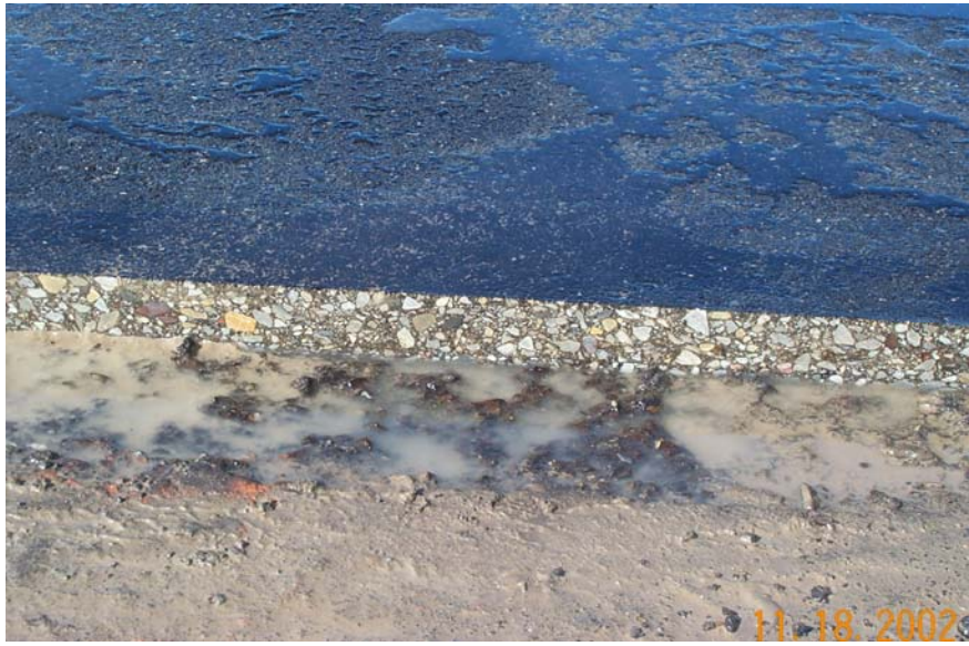
Figure 38. Clean washed cut edge
