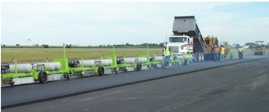
Figure 15. Use of Joint-Heating System
