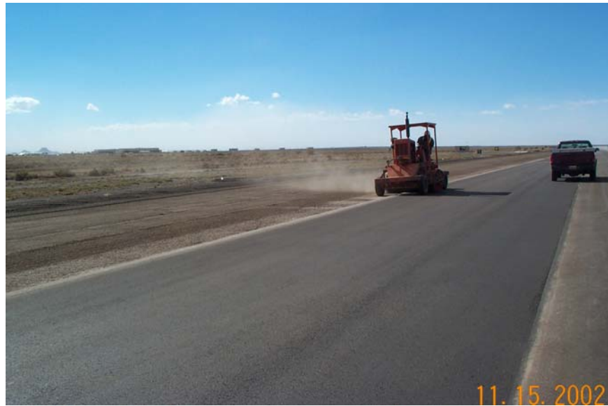
Figure 39. Cleaning joint prior to tack application
