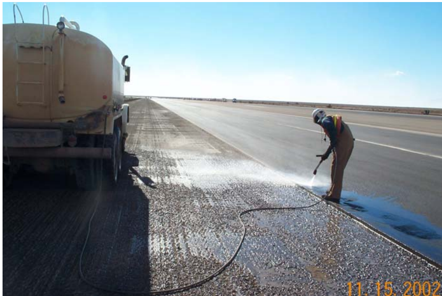
Figure 37. Power washing cut edge joint
