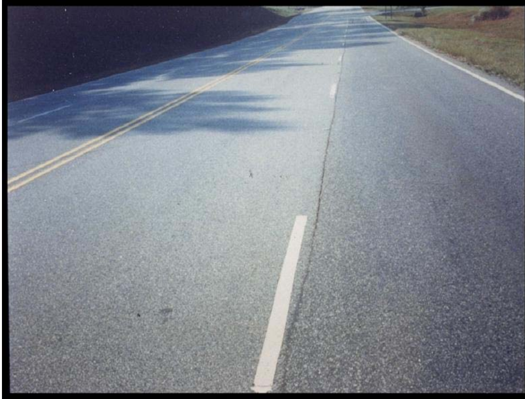
Figure 3. Typically a crack develops at the longitudinal joint
