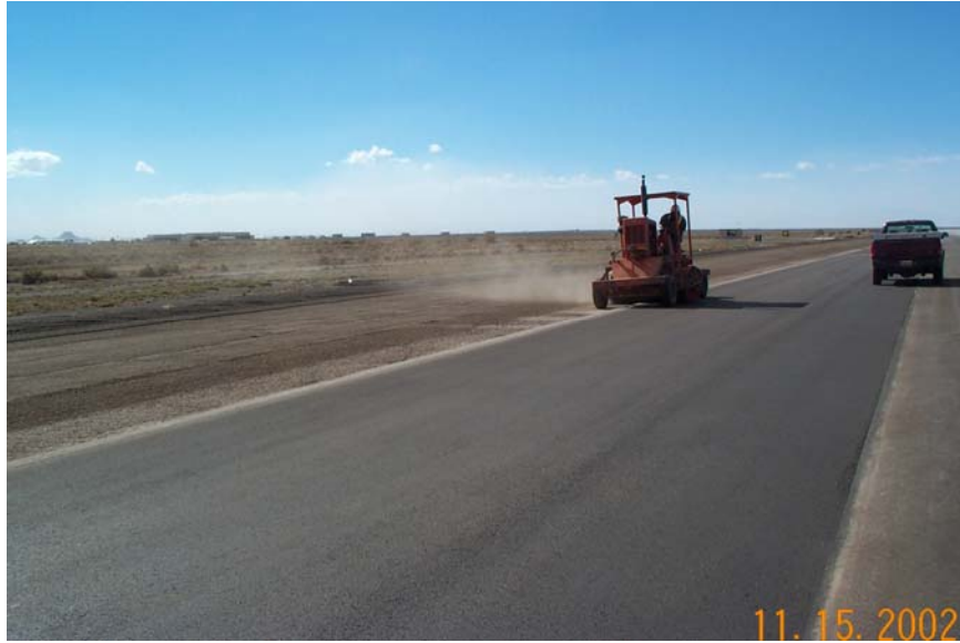
Figure 7. Cleaning joint prior to tack application
