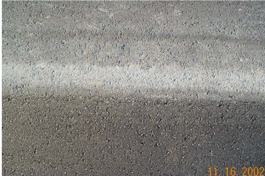
Figure 13. Properly compacted longitudinal joint
