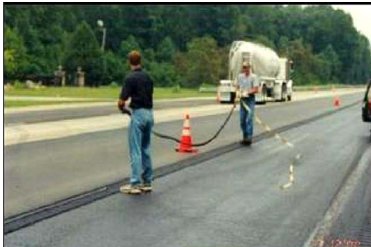
Figure 31. HMA joint tape being applied to a notched wedge joint
