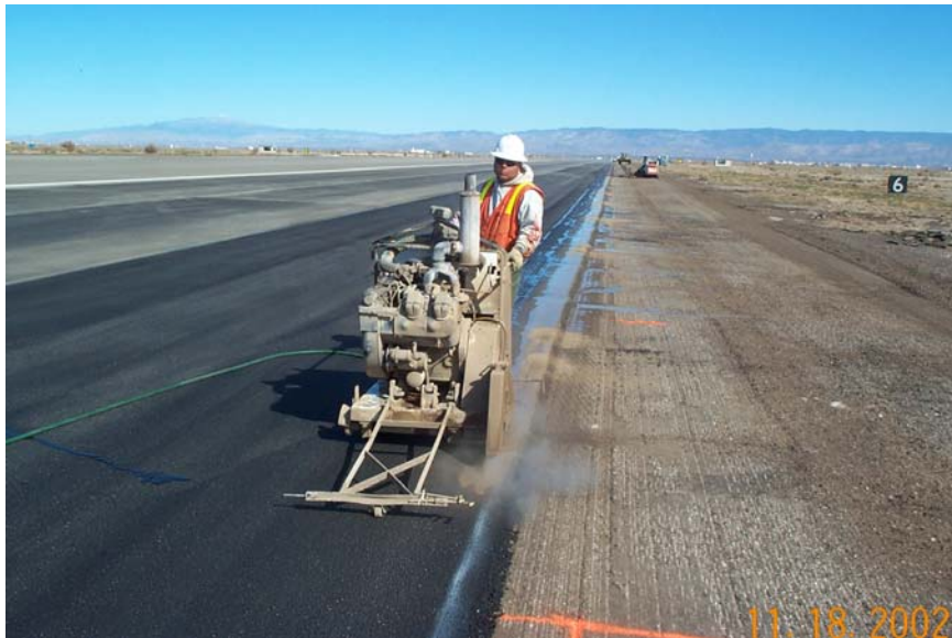
Figure 2. Sawing operations
