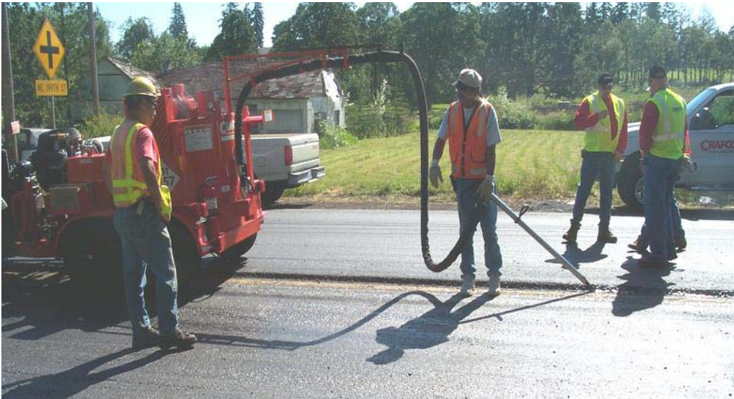
Figure 11. Application equipment for rubberized asphalt tack coat (joint adhesive)
