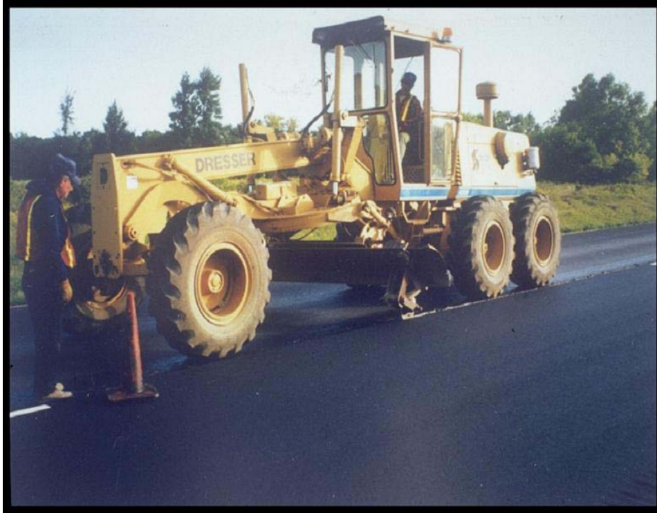
Figure 21. Cutting wheel mounted on a motor grader
