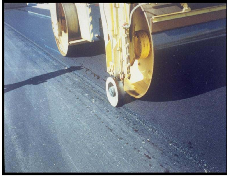
Figure 25. Close up of edge restraining device
