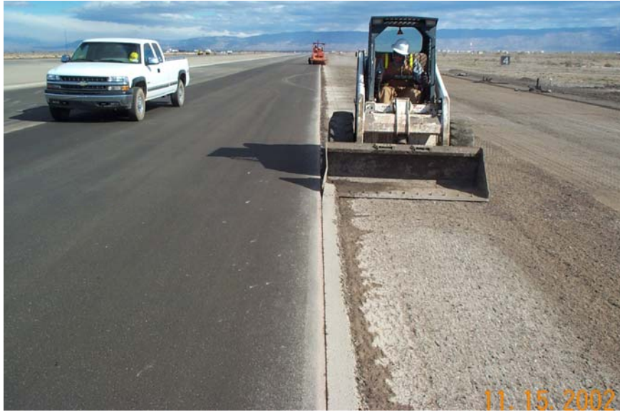
Figure 3. Removing approximately 200 mm of unconfined edge
