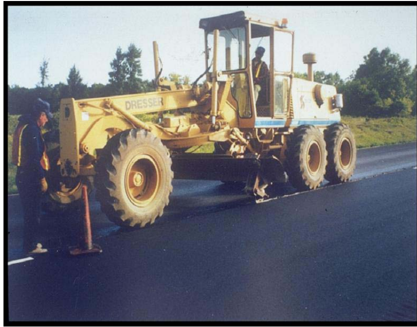
Figure 13. Cutting wheel mounted on a motor grader
