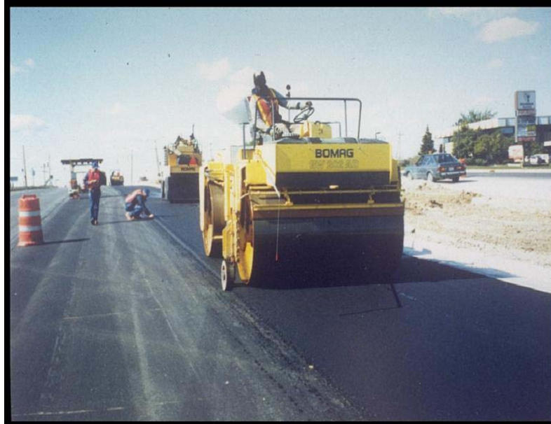
Figure 24. Edge restraining device being used
