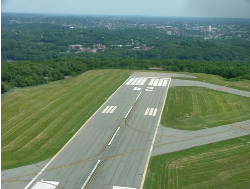
Figure 1. Aerial view of airport runway showing longitudinal joints
