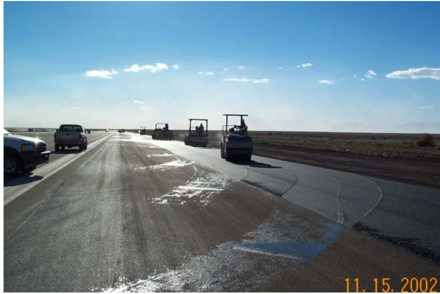
Figure 11. Compaction rolling pattern
