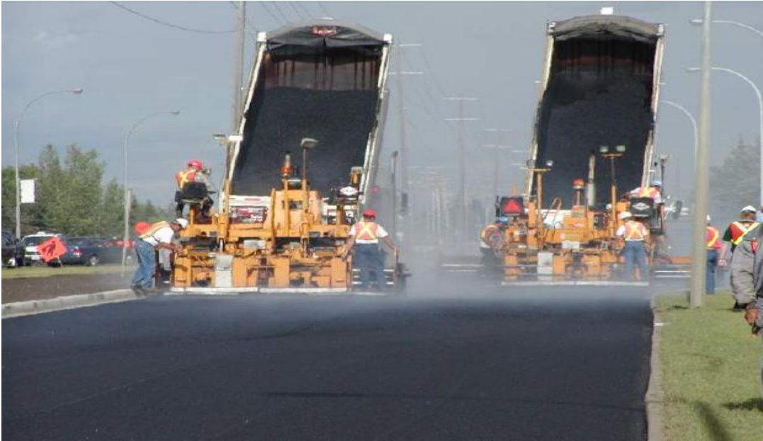
Figure 3. Paving in echelon
