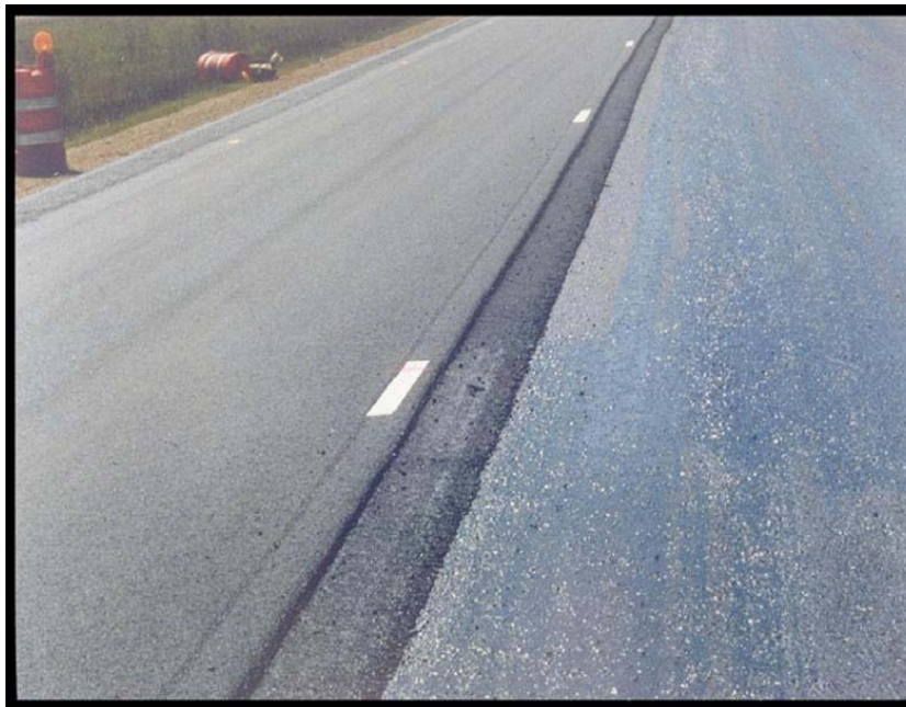
Figure 19. View of finished notched wedge joint
