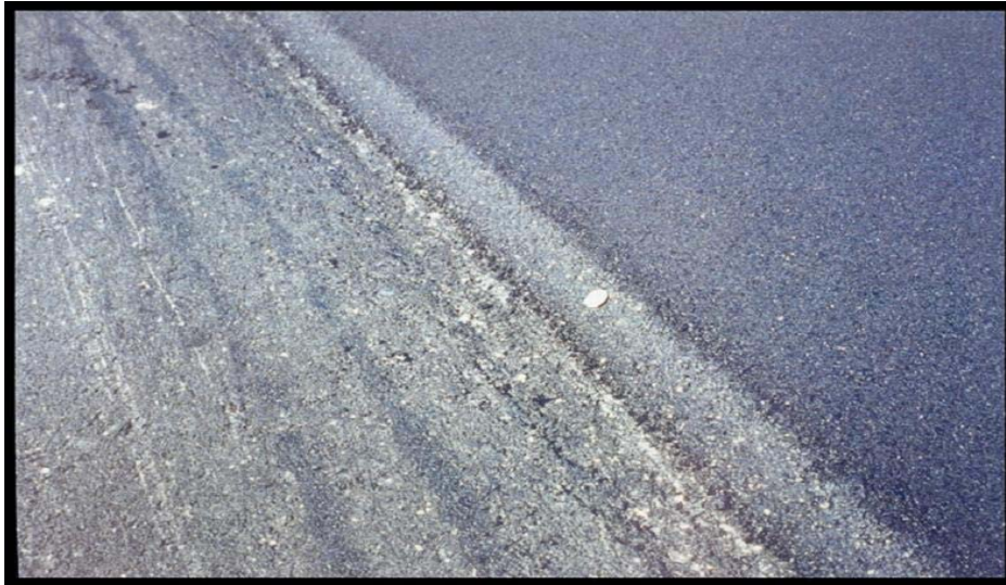
Figure 26. View of the edge compacted with the edge restraining device
