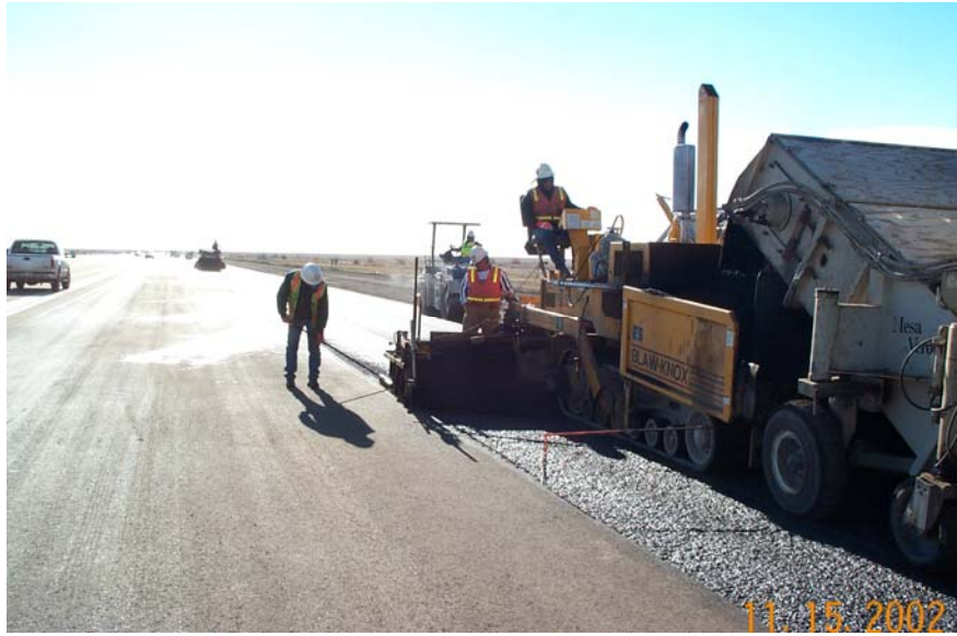
Figure 9. Minimum raking
