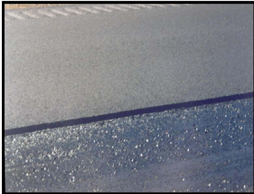
Figure 14. View of the edge after the use of cutting wheel
