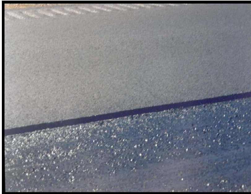
Figure 22. View of the edge after the use of cutting wheel
