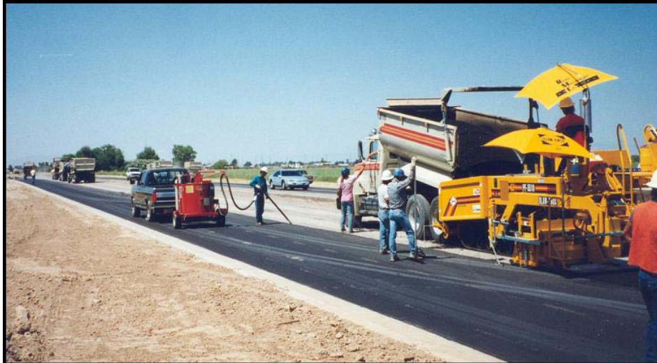
Figure 10. Application of rubberized asphalt tack coat at joint ahead of paving
