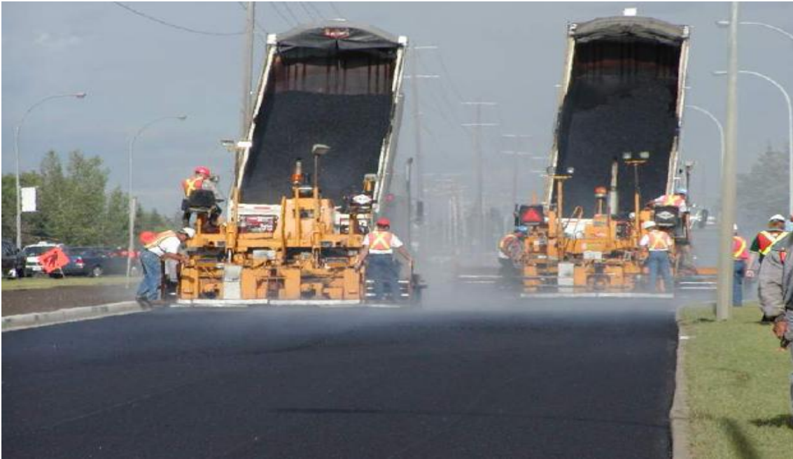
Figure 8. Paving in echelon
