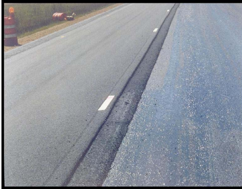
Figure 9. View of finished notched wedge joint
