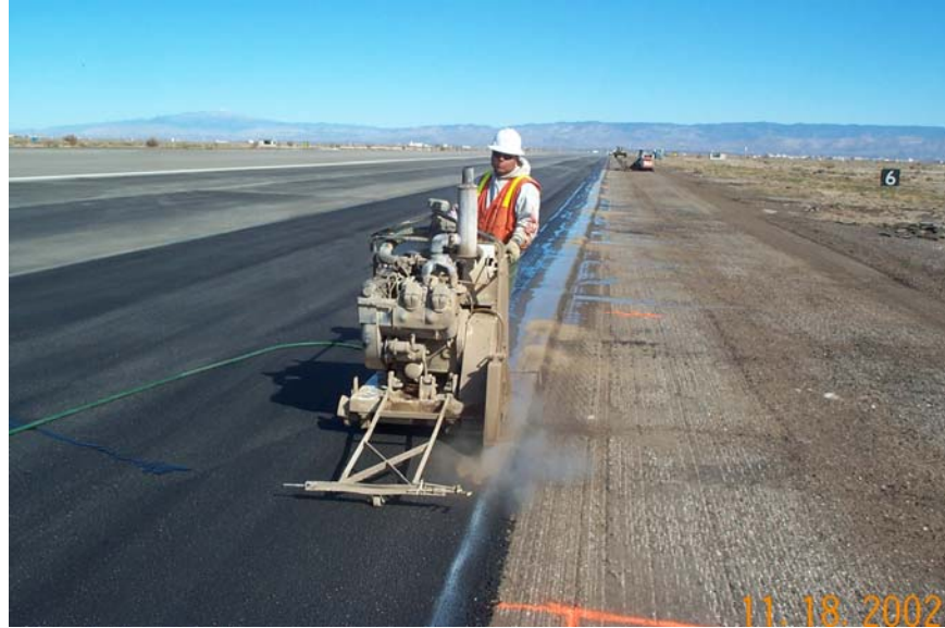
Figure 34. Sawing operations
