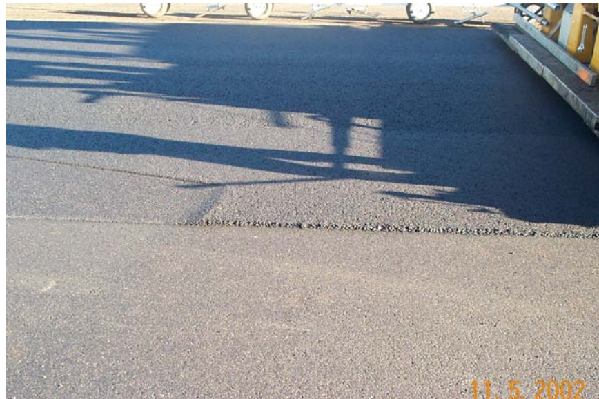
Figure 12. Rolling joint behind paver
