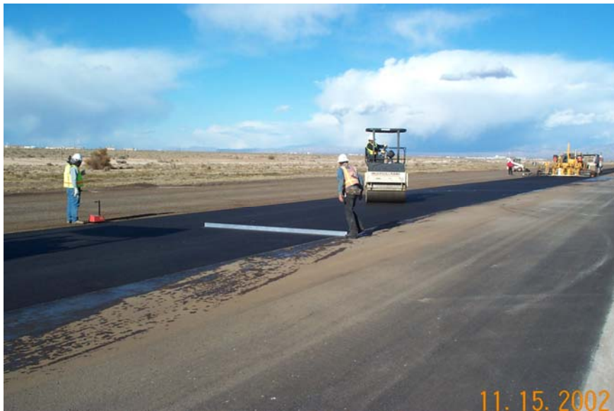
Figure 10. Quality control process during paving operation
