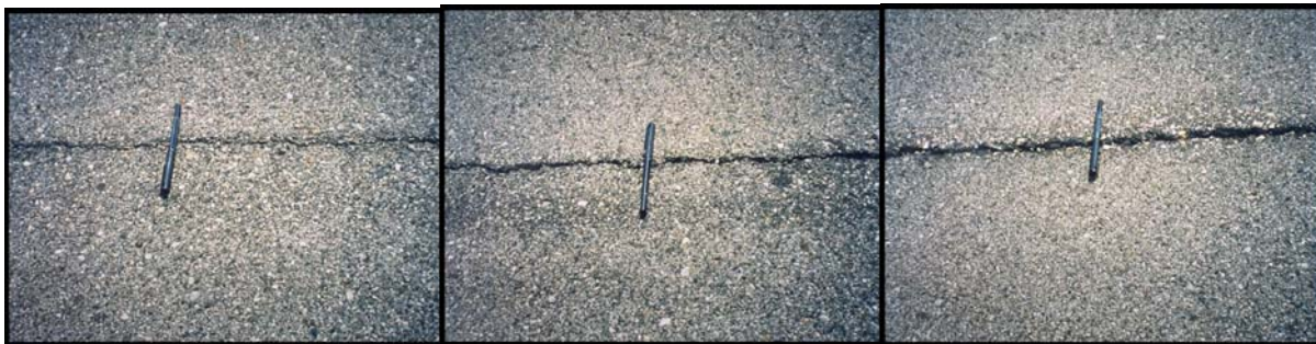
Figure 3. Typically a crack develops at the longitudinal joint
