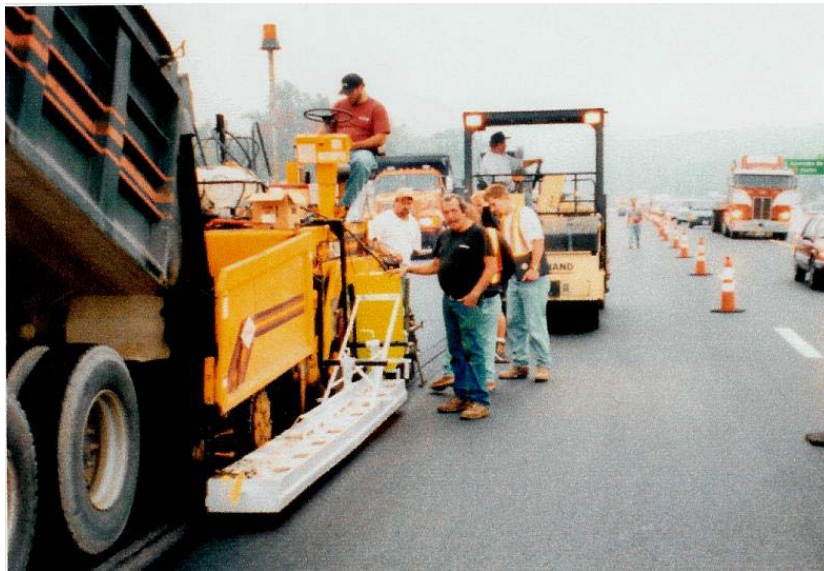
Figure 30. Infrared heater mounted on the paver
