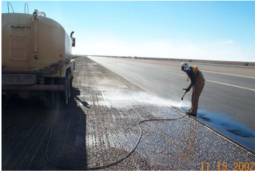
Figure 5. Power washing cut edge joint
