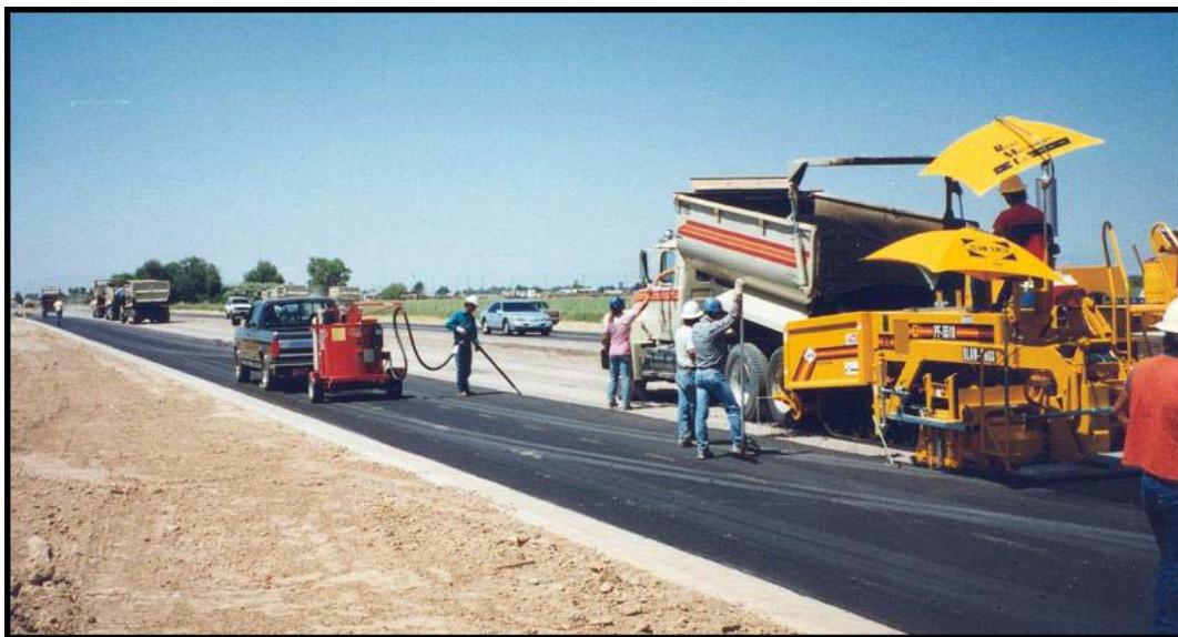
Figure 14. Application of rubberized asphalt tack coat at joint ahead of paving
