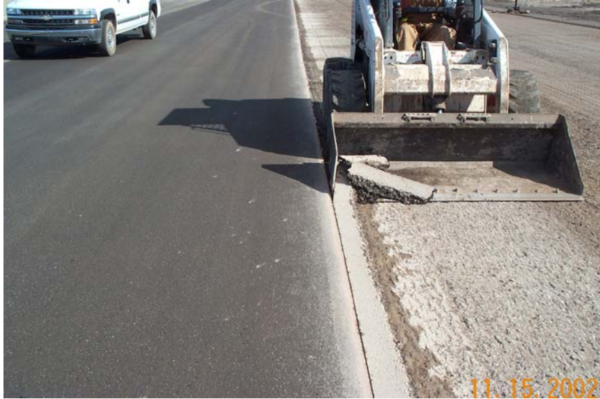
Figure 36. Removing cut edge
