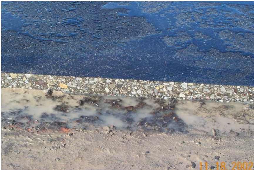
Figure 6. Clean washed cut edge
