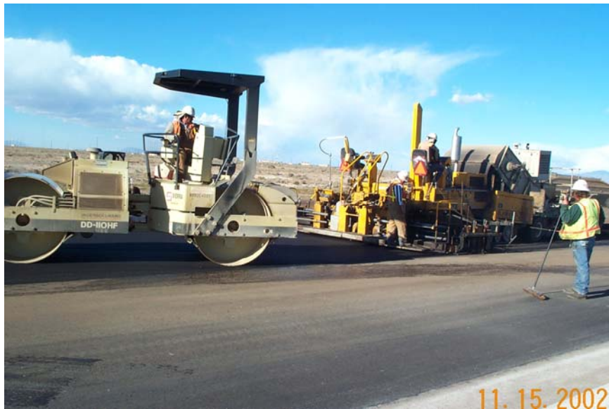
Figure 8. Heavy breakdown roller immediately behind paver rolling joint
